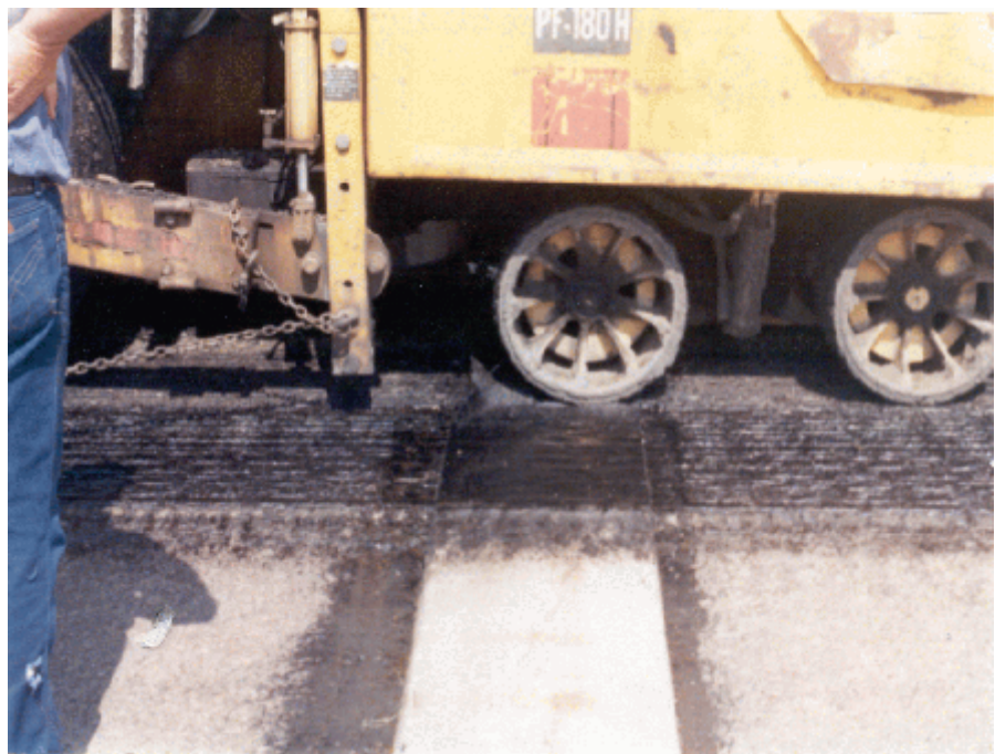
Photo 2--Paver wheels lifting PavePrep
