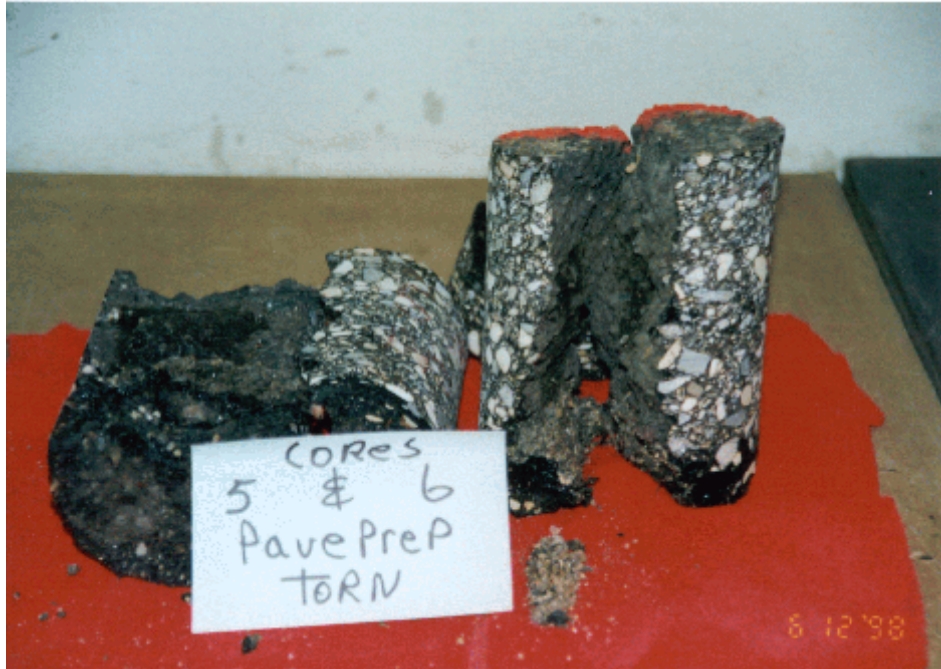
Photo 5--Cores 5&6 on Highway 17-----PavePrep torn
