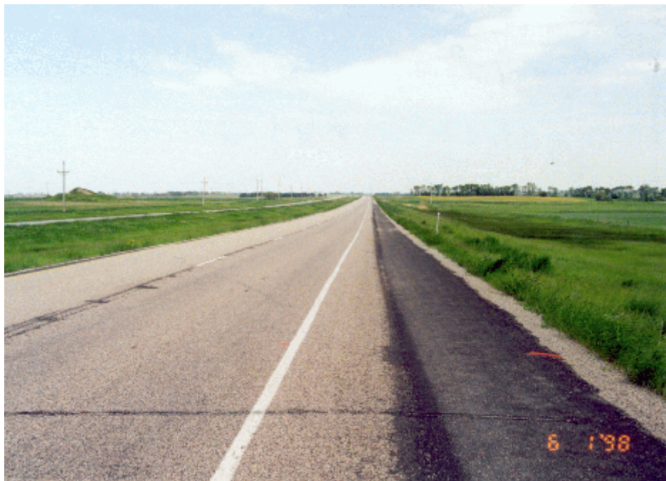
Photo 7 --PavePrep section overview--looking east
