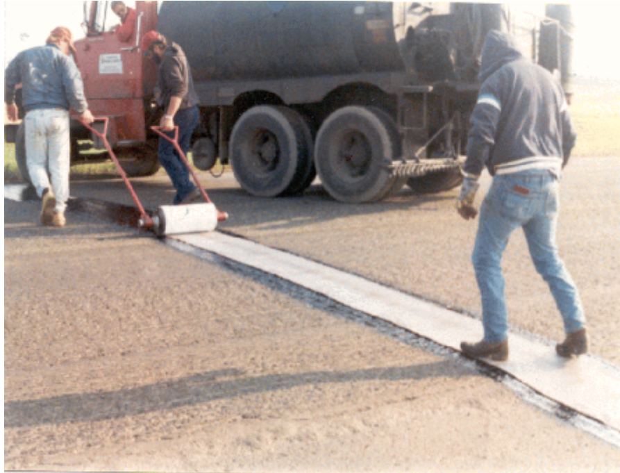
Photo 1--PavePrep installation
