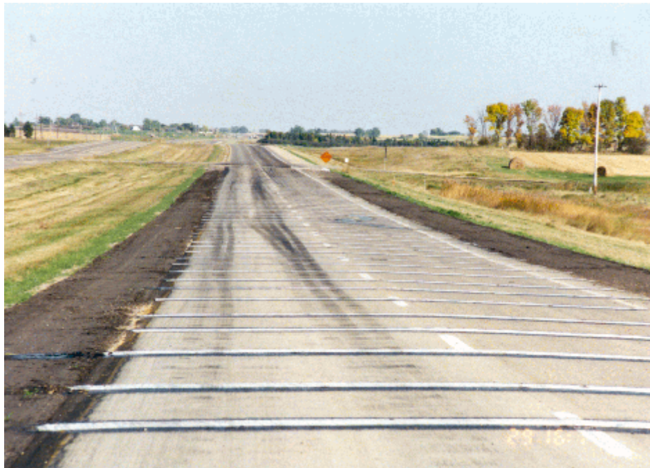
Photo 6 --East end overview of PavePrep section
