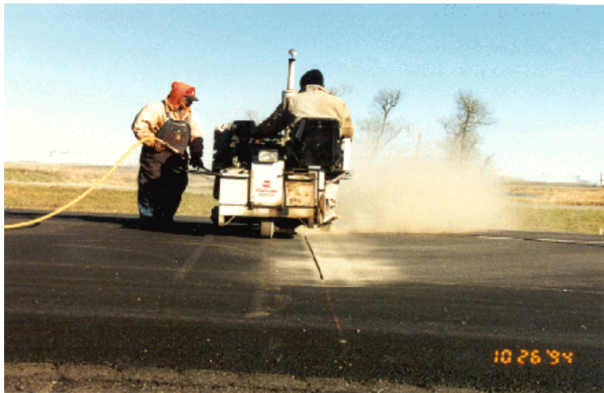
Photo 3 A view of the saw cutting operation
