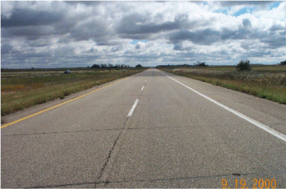
Photo 1 Overview of the Saw and Seal Section just east of Knox
