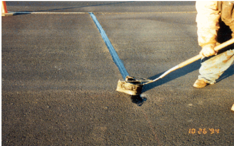
Photo 6 A view of the squeegee operation .
