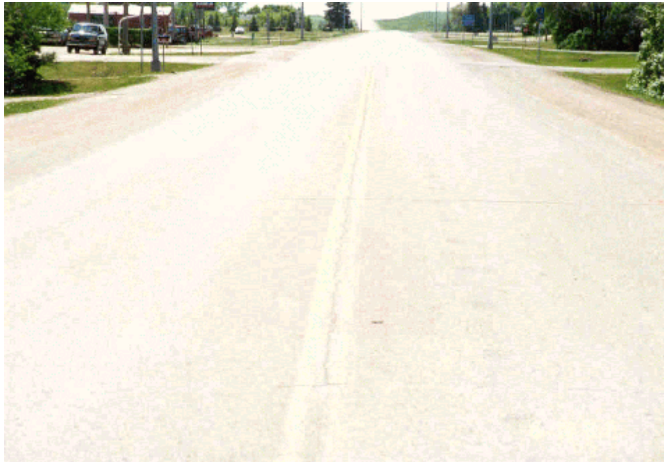
Photo 8. Overview of the test section looking north.
