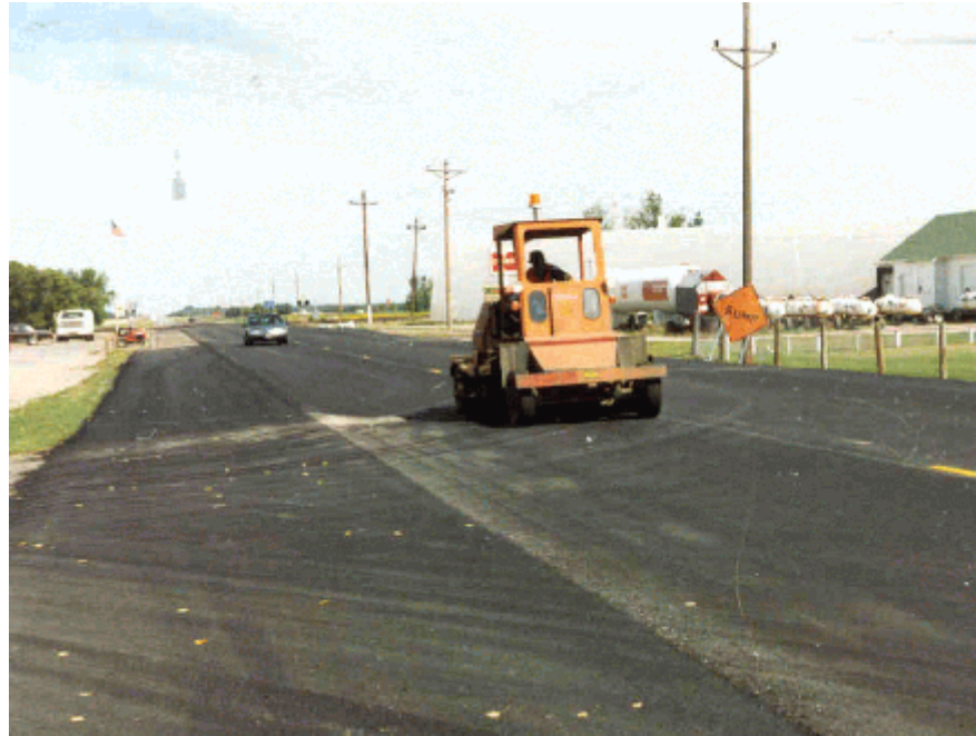
Photo 1. View of the sweeping process on Hwy 32.
