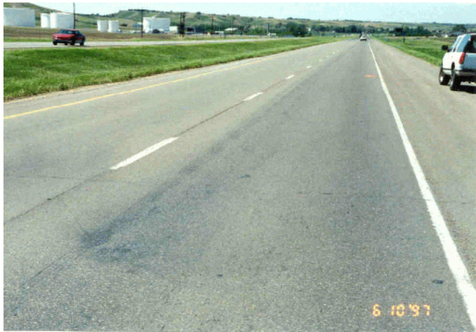
Photo 23. An overview of the west control section.
