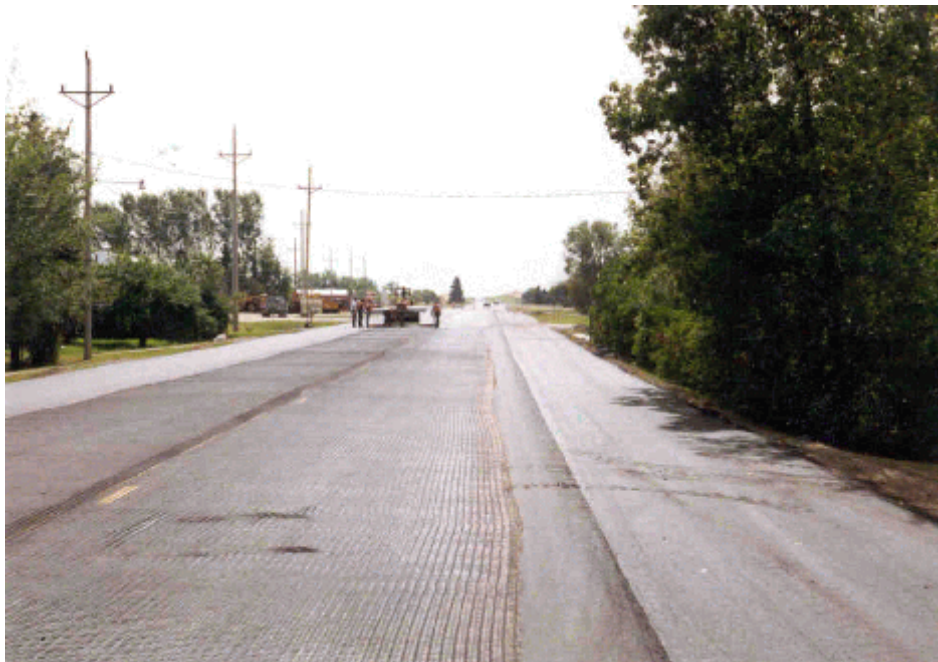
Photo 2. View of the geogrid rolled out.
