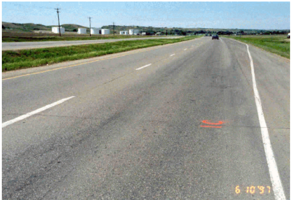
Photo 21. An overview of the east control section.
