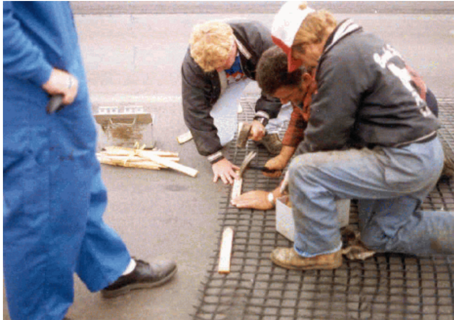
Photo 7. View of the lathe-nail system.
