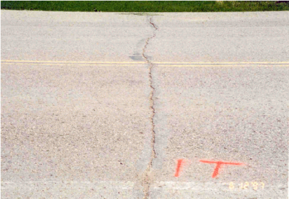
Photo 9. View of a transverse crack in the stratagid test section
