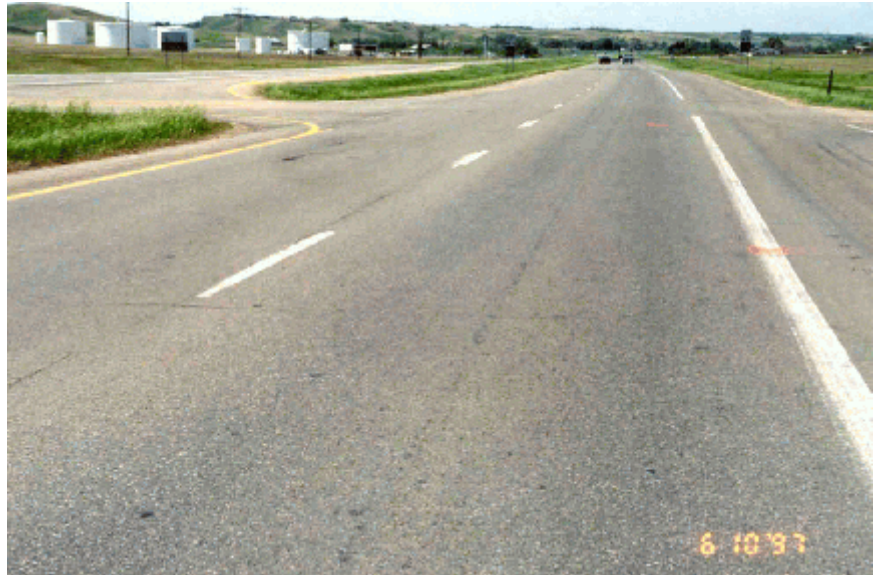
Photo 17. An overview of the stratagrid test section
