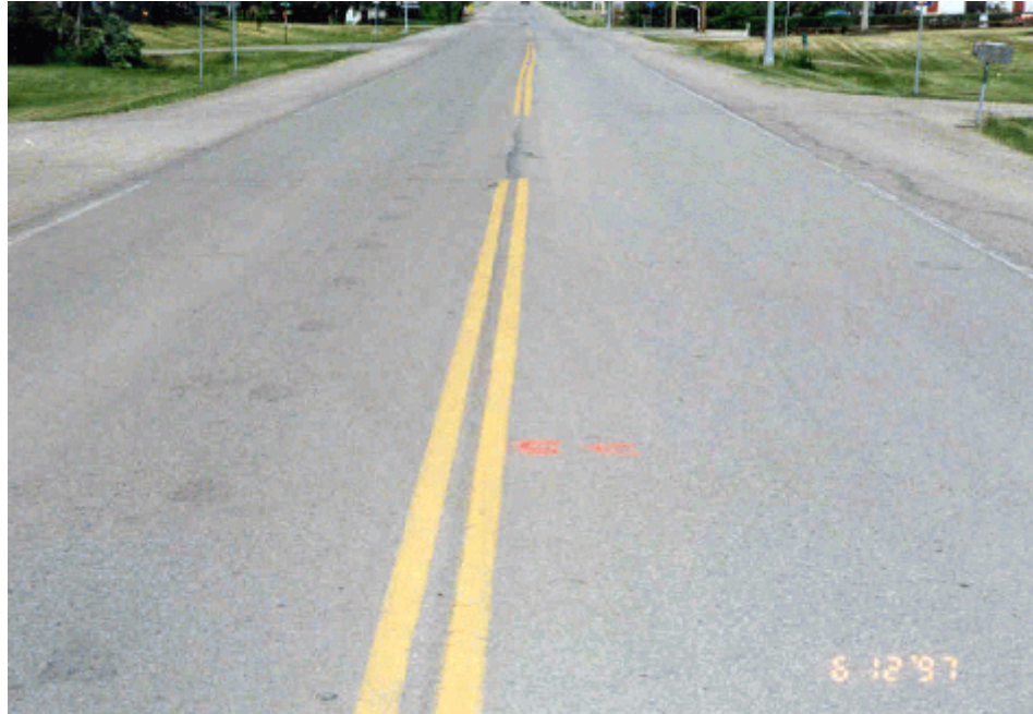
Photo 12. View of the control section looking north.
