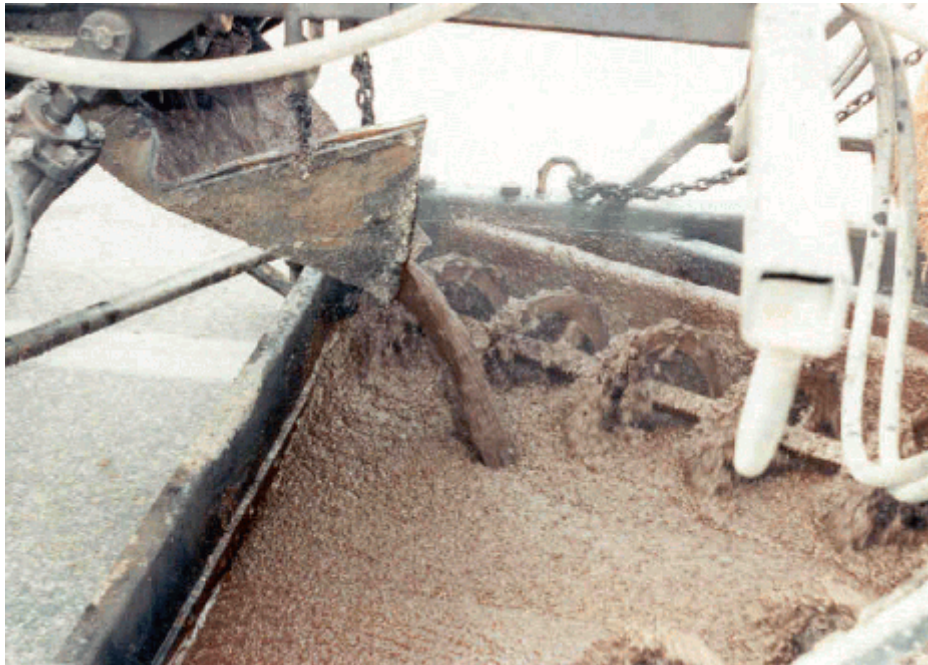
Photo 2. Continuous flow of the Ralumac slurry into the spreader box
