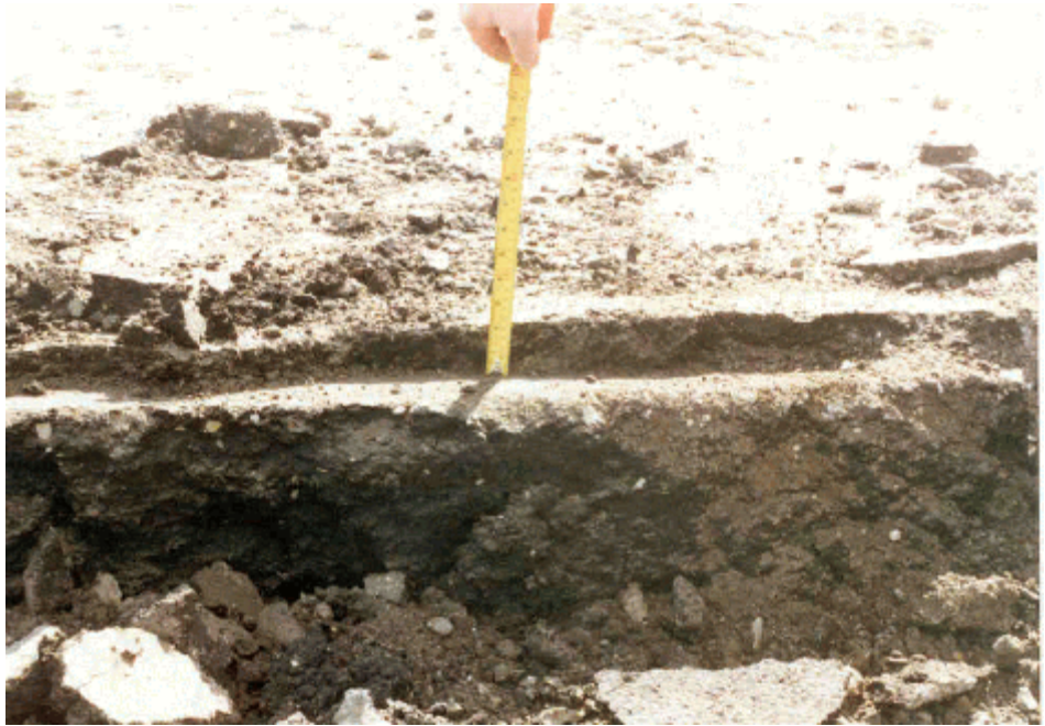
Photo 9. Subgrade repair section -- measuring Ralumac thickness
