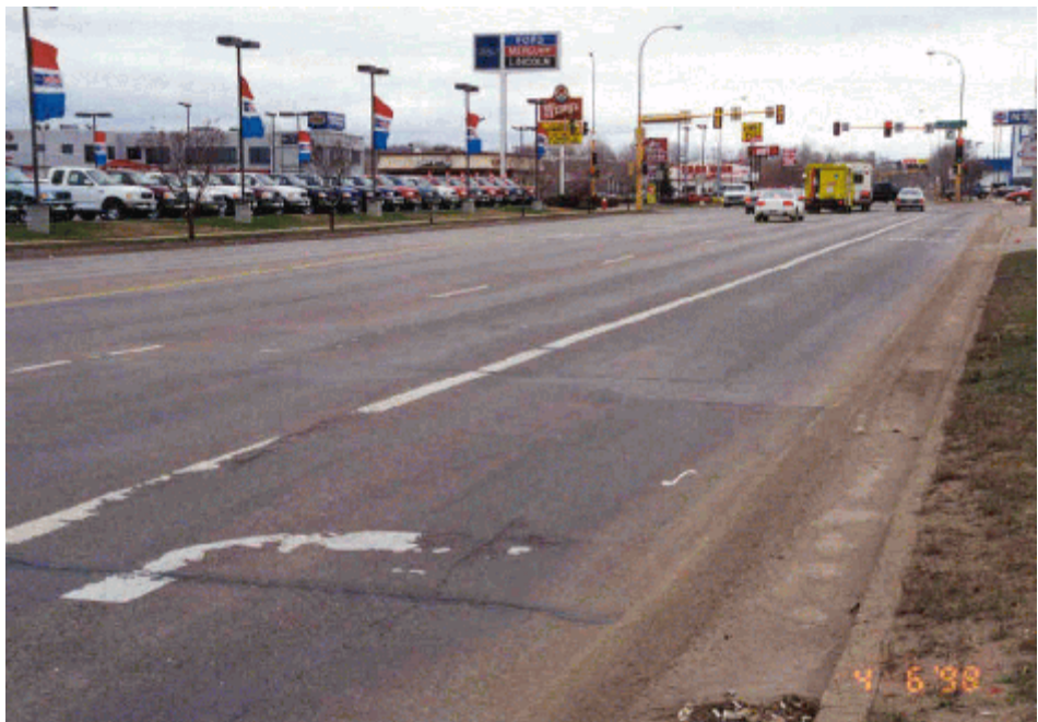
Photo 10. Line indicates where subgrade repair begins+ 370 feet
