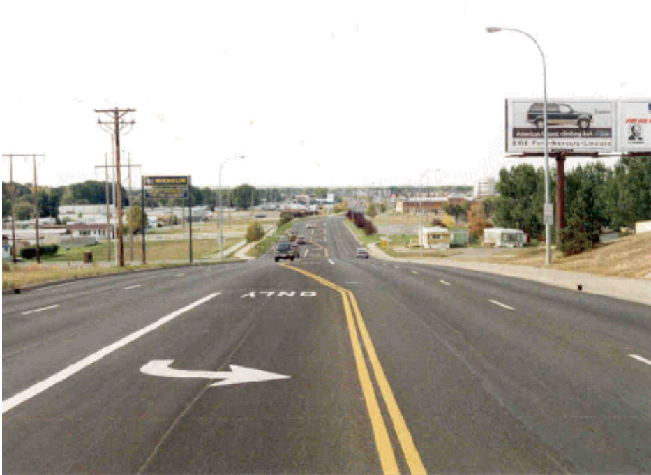
Photo 4. Finished project looking west from 18th street on Expressway
