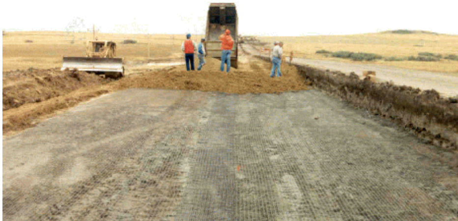
Photo 3: View of geogrid installation at test section B
