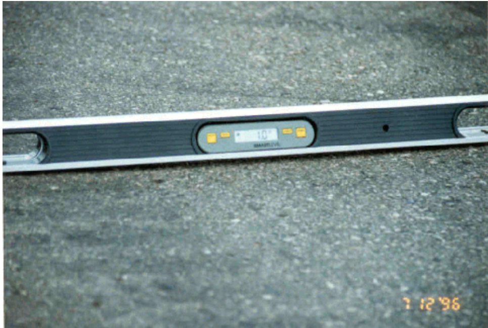
Photo 4: View of rutting in test section A
