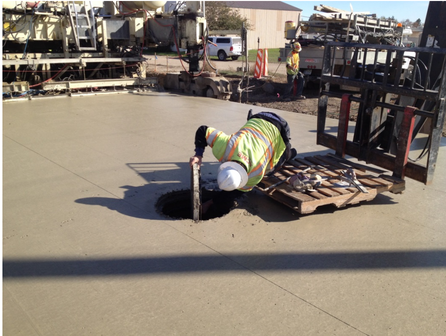
Photo 4: Concrete Finisher making elevation adjustments.
