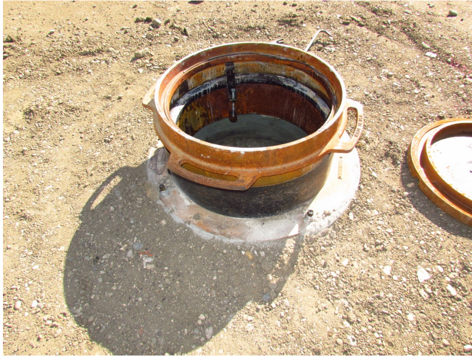
Photo 1: EJ 3025 SELFLEVEL manhole casting installed.
