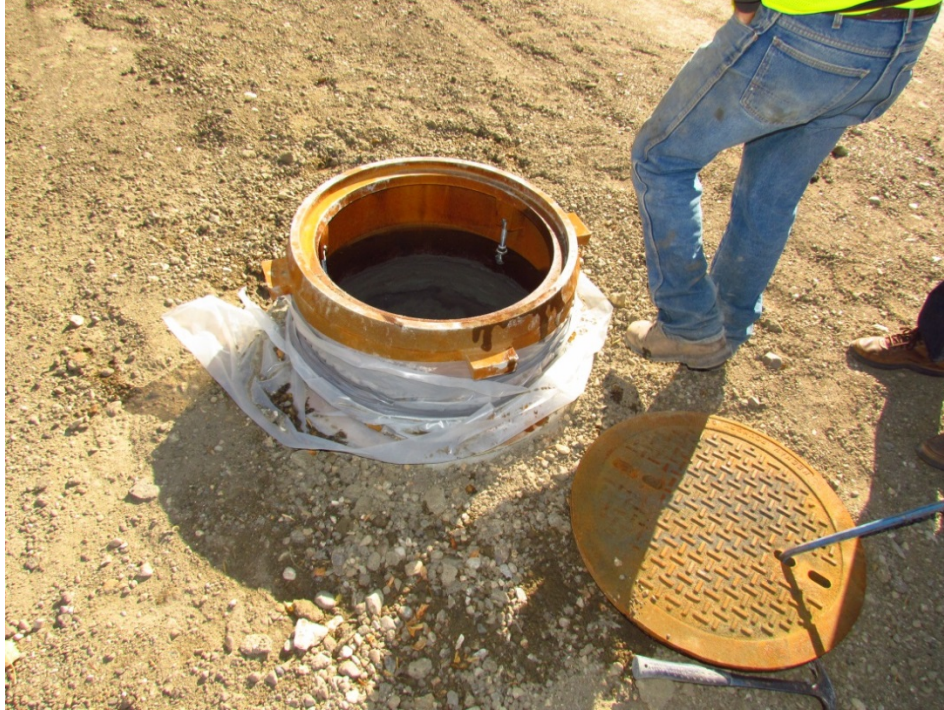
Photo 2: NDDOT typical "Manhole Casting Type 1"
