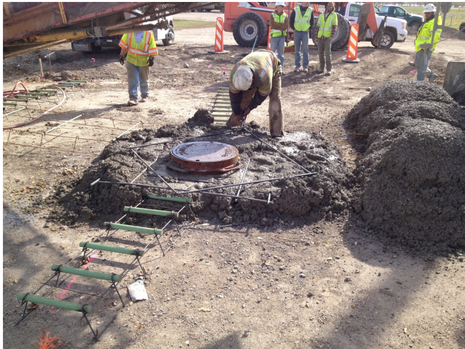
Photo 3: Rebar installation prior to paving train.
