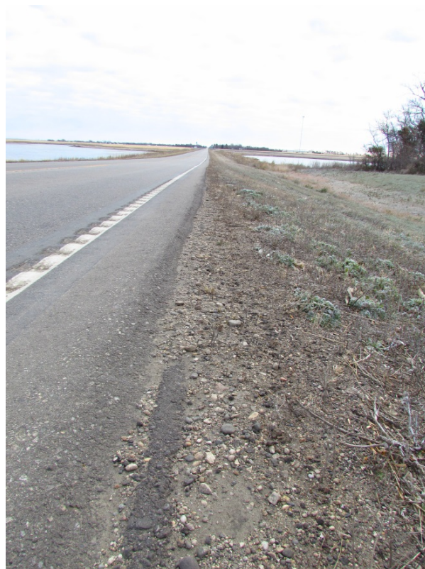
Photo 8: (ND 3, RP 8) - 30° Safety Edge Fall 2013 South Shoulder Facing East
