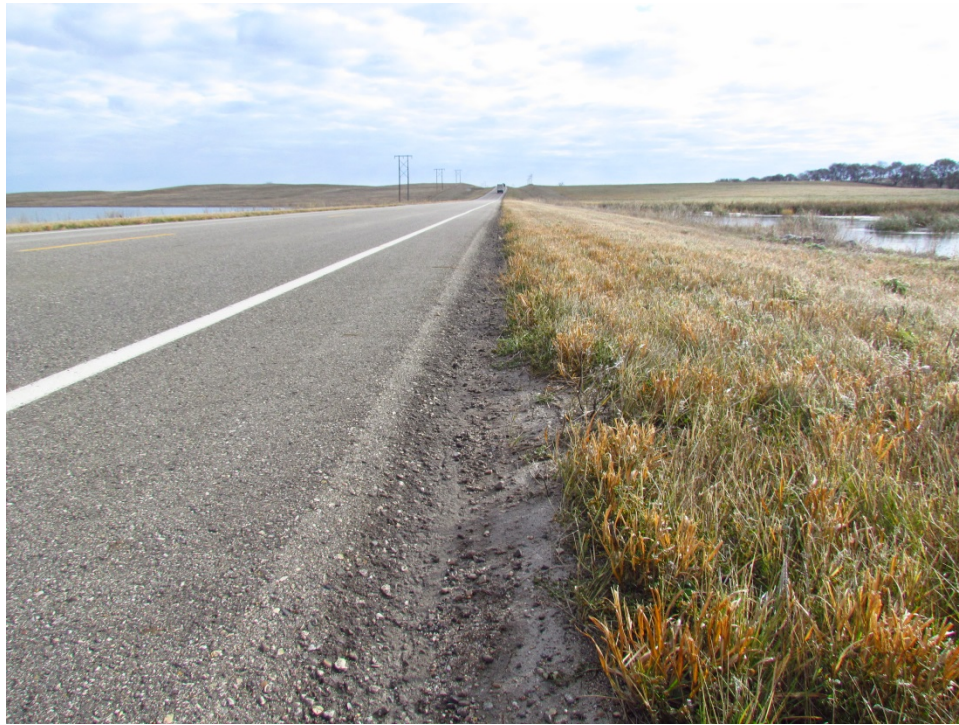
Photo 147: (ND 11, RP 47) Control, 4:1 NDDOT Standard South Shoulder Facing East
