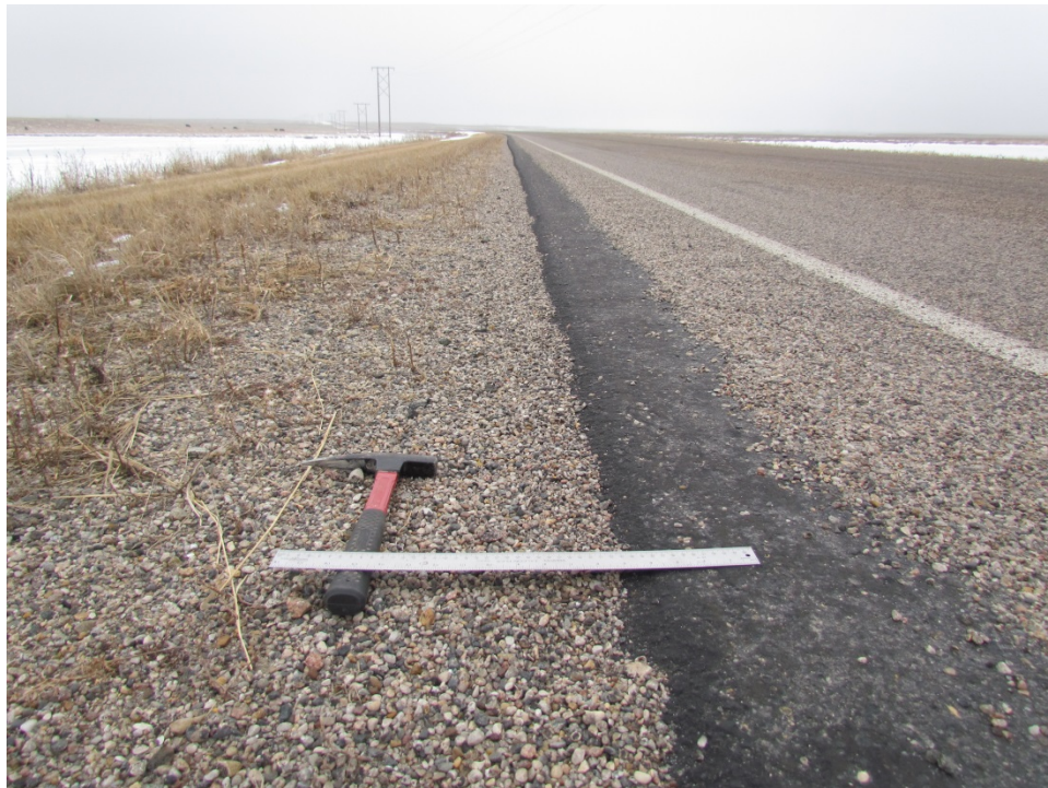
Photo 25: (ND 11, RP 41) - 30° Safety Edge 2014 North Shoulder Facing East
