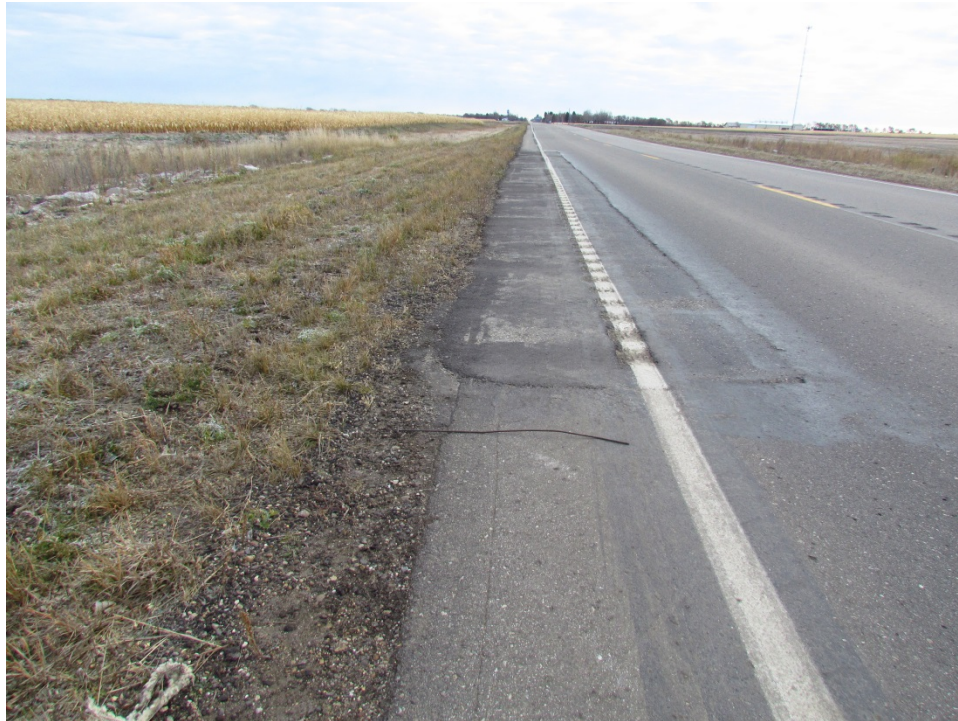
Photo 6: Project SER-2-003(018)008 localized HBP shoulder repair.
