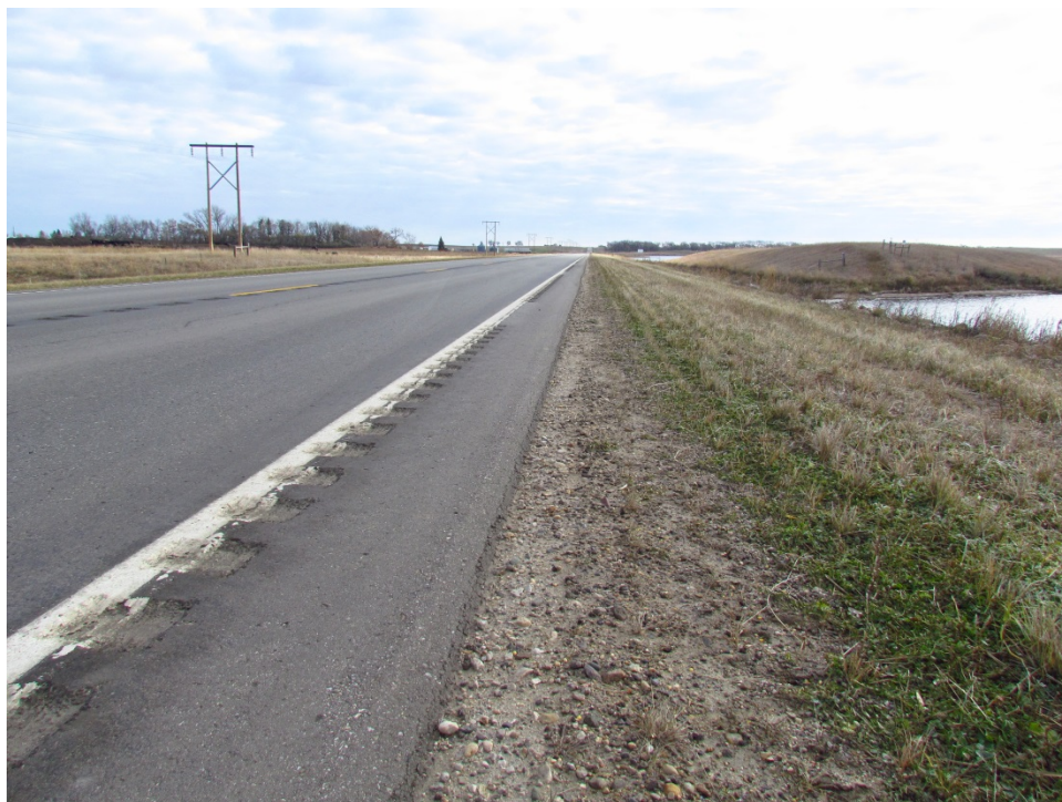
Photo 92 :( ND 11, RP 45) - 30° Safety Edge South Shoulder Facing East
