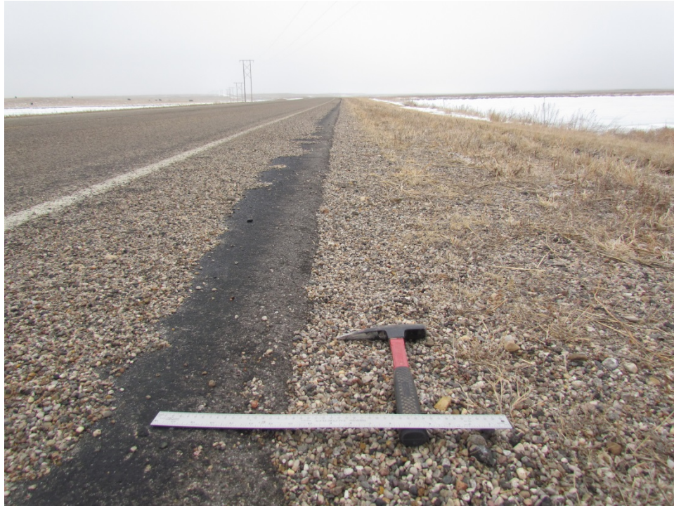
Photo 24: (ND 11, RP 41) - 30° Safety Edge 2014 South Shoulder Facing East
