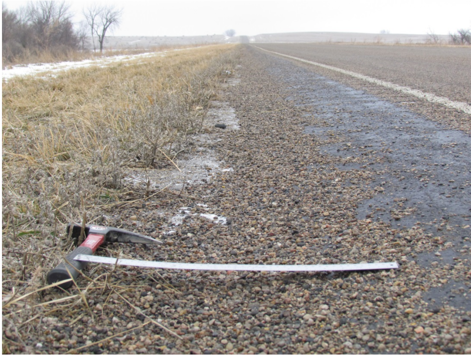
Photo 33: (ND 30, RP 7) 2014 Control 30° Contractor Constructed West Shoulder Facing North
