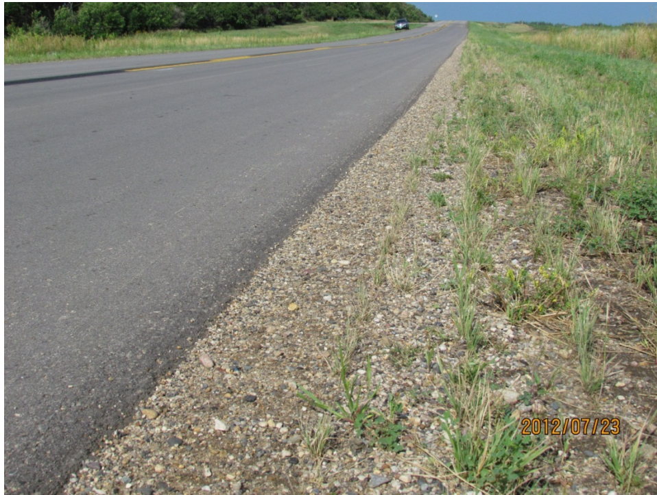
Photo 5: Finished safety edge on project #SER-2-003(018)008.
