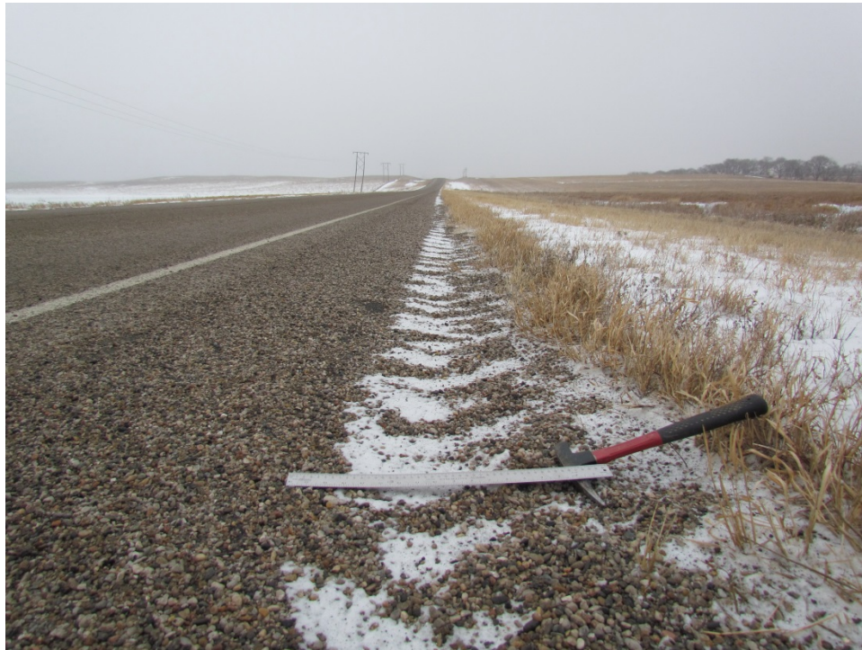
Photo 32: (ND 11, RP 47) 2014 Control, 4:1 NDDOT Standard South Shoulder Facing East
