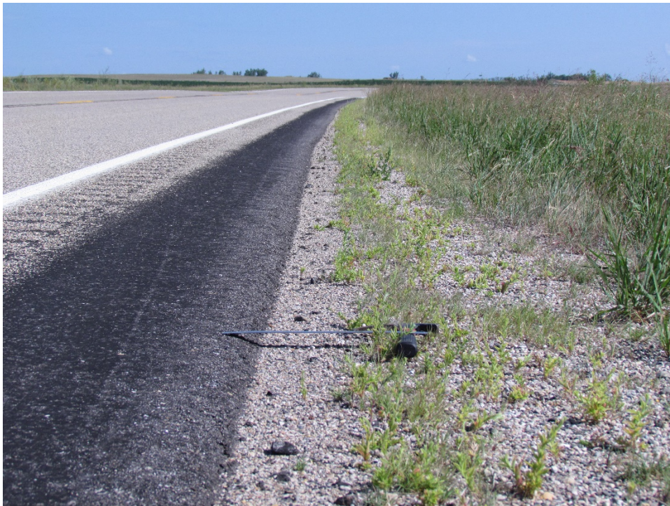
Photo 47: (ND 56, RP 7) 2014 Control 30° Contractor Constructed East Shoulder Facing North
