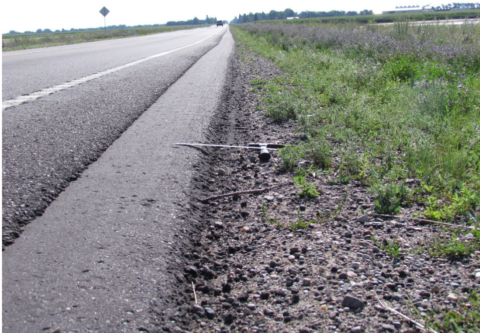
Photo 37: (ND 3, RP 8) - 30° Safety Edge Fall 2014 South Shoulder Facing East
