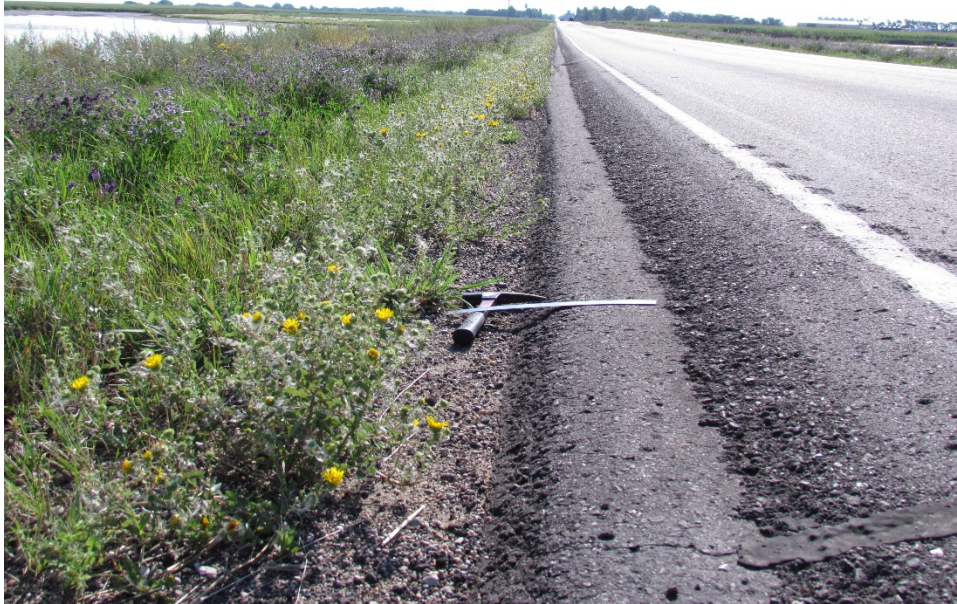
Photo 36: (ND 3, RP 8) - 30° Safety Edge Fall 2014 North Shoulder Facing East
