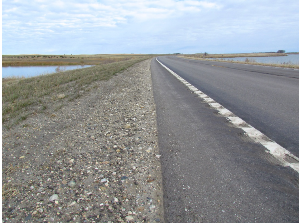
Photo 171: (ND 56, RP 7) Control 30° Contractor Constructed West Shoulder Facing North
