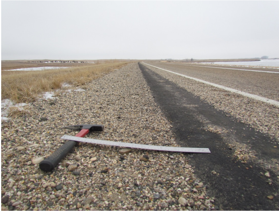
Photo 35: (ND 56, RP 7) 2014 Control 30° Contractor Constructed West Shoulder Facing North
