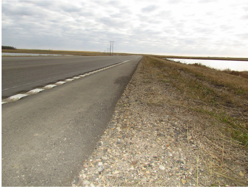
Photo 9: (ND 11, RP 41) - 30° Safety Edge South Shoulder Facing East
