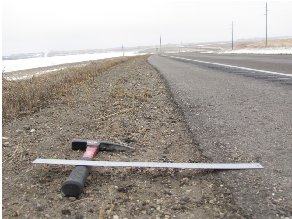
Photo 31: (ND 46, RP 13) - 30° Safety Edge 2014 North Shoulder Facing East
