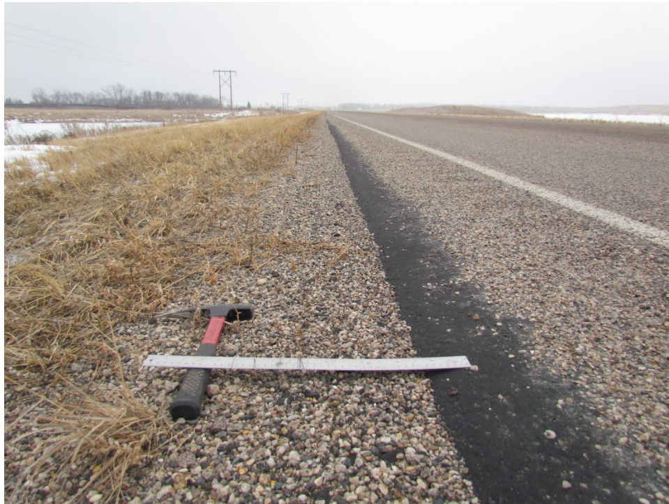
Photo 26: (ND 11, RP 45) - 30° Safety Edge 2014 North Shoulder Facing East
