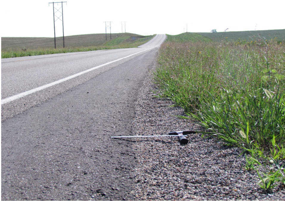
Photo 46: (ND 11, RP 47) 2014 Control, 4:1 NDDOT Standard South Shoulder Facing East
