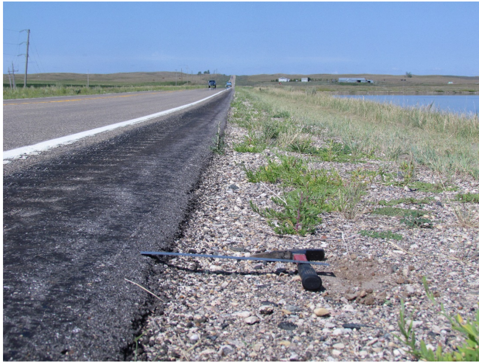
Photo 42 :( ND 13, RP 249) - 30° Safety Edge 2014 North Shoulder Facing West
