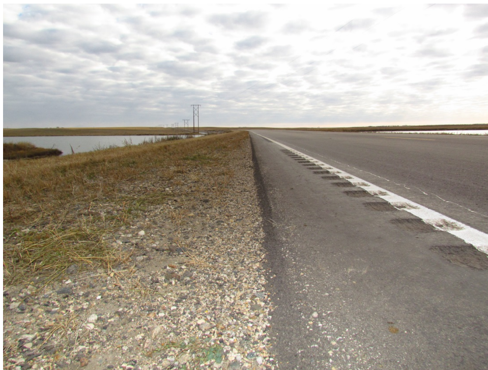
Photo 70: (ND 11, RP 41) - 30° Safety Edge North Shoulder Facing East
