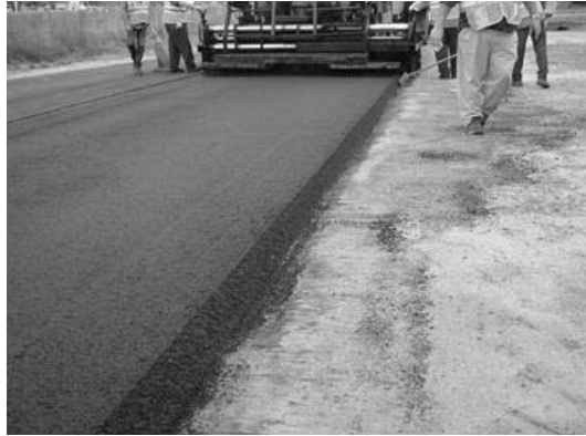
Paving road with safety edge
