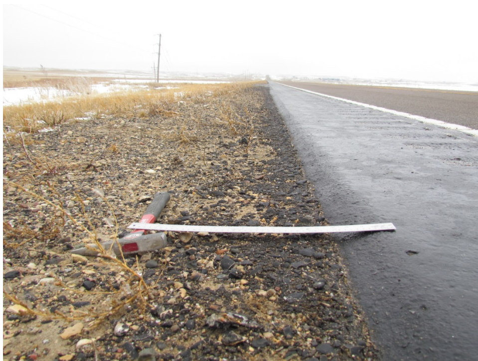
Photo 29: (ND 13, RP 249) - 30° Safety Edge 2014 South Shoulder Facing West
