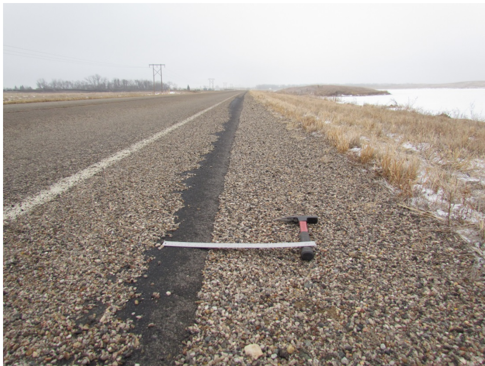
Photo 27 : ( ND 11, RP 45) - 30° Safety Edge 2014 South Shoulder Facing East
