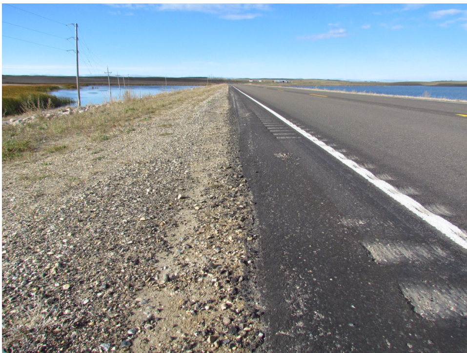
Photo 114: (ND 13, RP 249) - 30° Safety Edge South Shoulder Facing West
