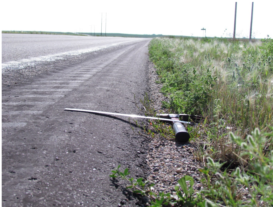
Photo 39: (ND 11, RP 41) - 30° Safety Edge 2014 South Shoulder Facing East
