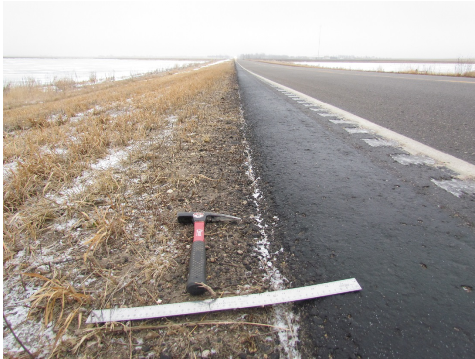
Photo 22: (ND 3, RP 8) - 30° Safety Edge Fall 2014 North Shoulder Facing East
