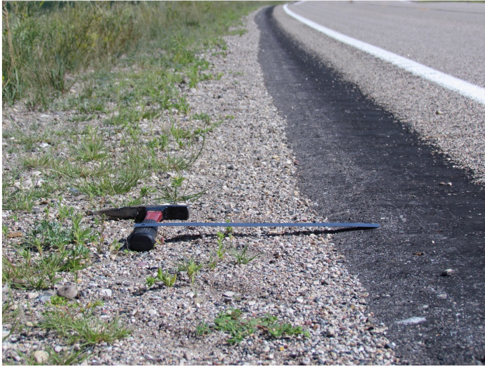
Photo 48: (ND 56, RP 7) 2014 Control 30° Contractor Constructed West Shoulder Facing North
