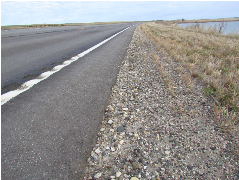
Photo 160: (ND 56, RP 7) Control 30° Contractor Constructed East Shoulder Facing North
