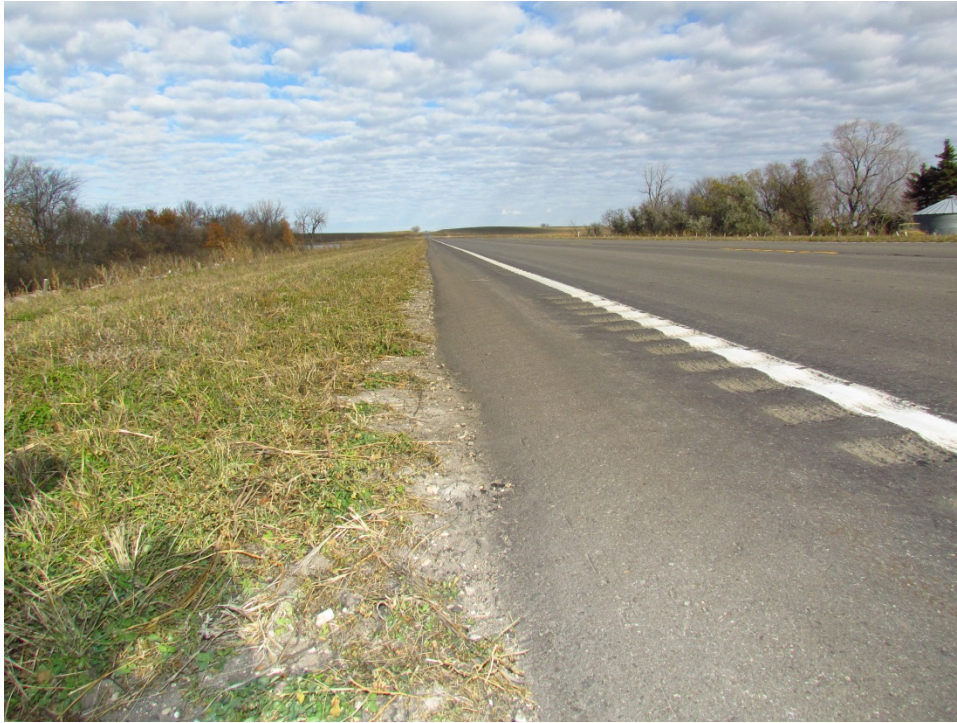
Photo 19: (ND 30, RP 7) Control 30° Contractor Constructed West Shoulder Facing North
