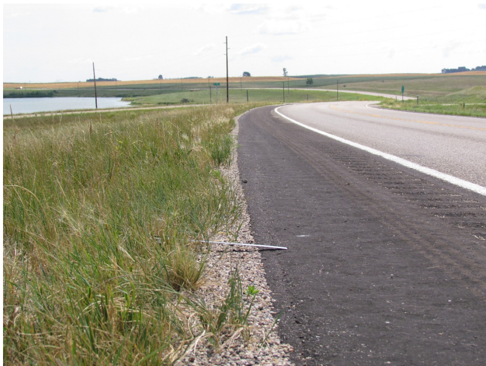
Photo 45: (ND 46, RP 13) - 30° Safety Edge 2014 North Shoulder Facing East
