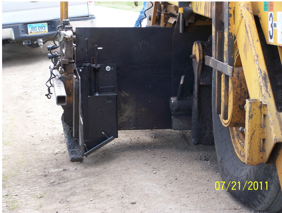
Photo 2: Ramp Champ paving shoe attached to paver.
