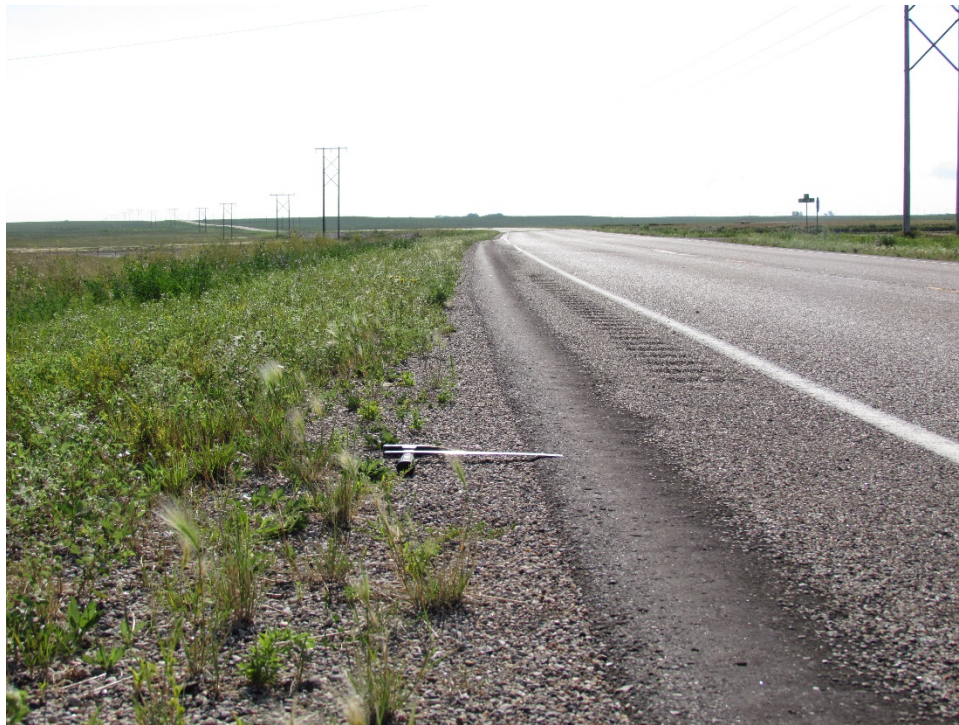
Photo 38: (ND 11, RP 41) - 30° Safety Edge 2014 North Shoulder Facing East
