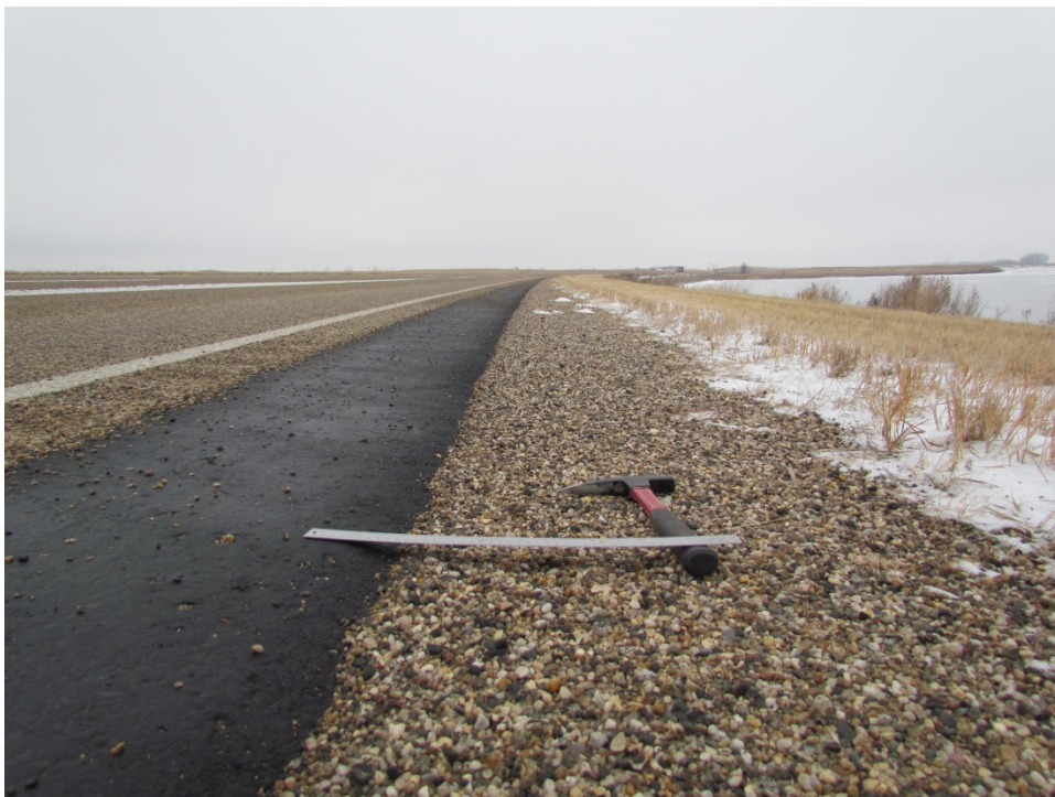
Photo 34: (ND 56, RP 7) 2014 Control 30° Contractor Constructed East Shoulder Facing North
