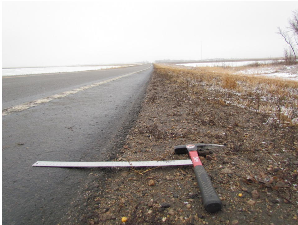
Photo 23: (ND 3, RP 8) - 30° Safety Edge Fall 2014 South Shoulder Facing East
