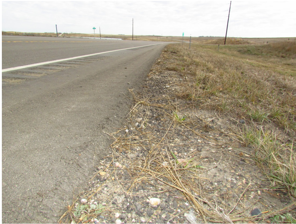
Photo 125: (ND 46, RP 13) - 30° Safety Edge South Shoulder Facing East
