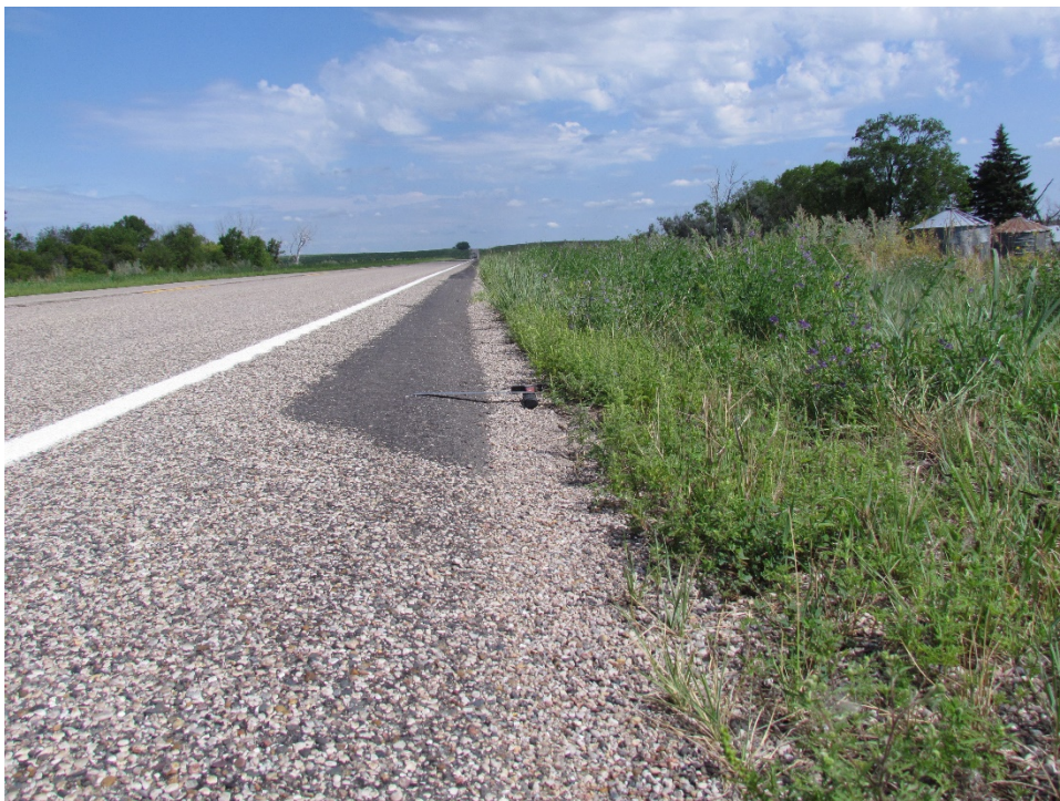
Photo 49: (ND 30, RP 7) Control 30° Contractor Constructed East Shoulder Facing North
