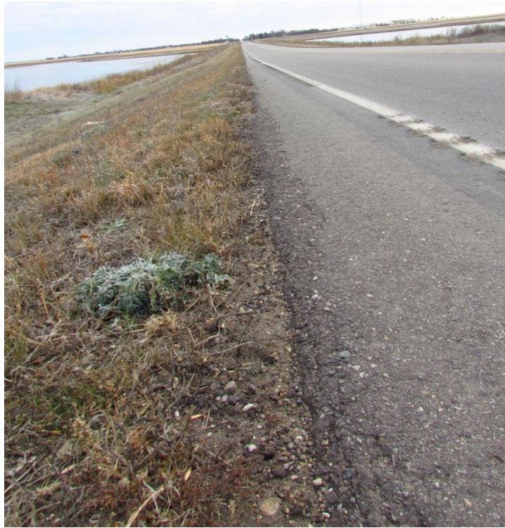
Photo 7: (ND 3, RP 8) - 30° Safety Edge Fall 2013 North Shoulder Facing East
