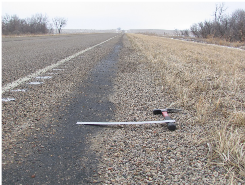
Photo 32: (ND 30, RP 7) 2014 Control 30° Contractor Constructed East Shoulder Facing North
