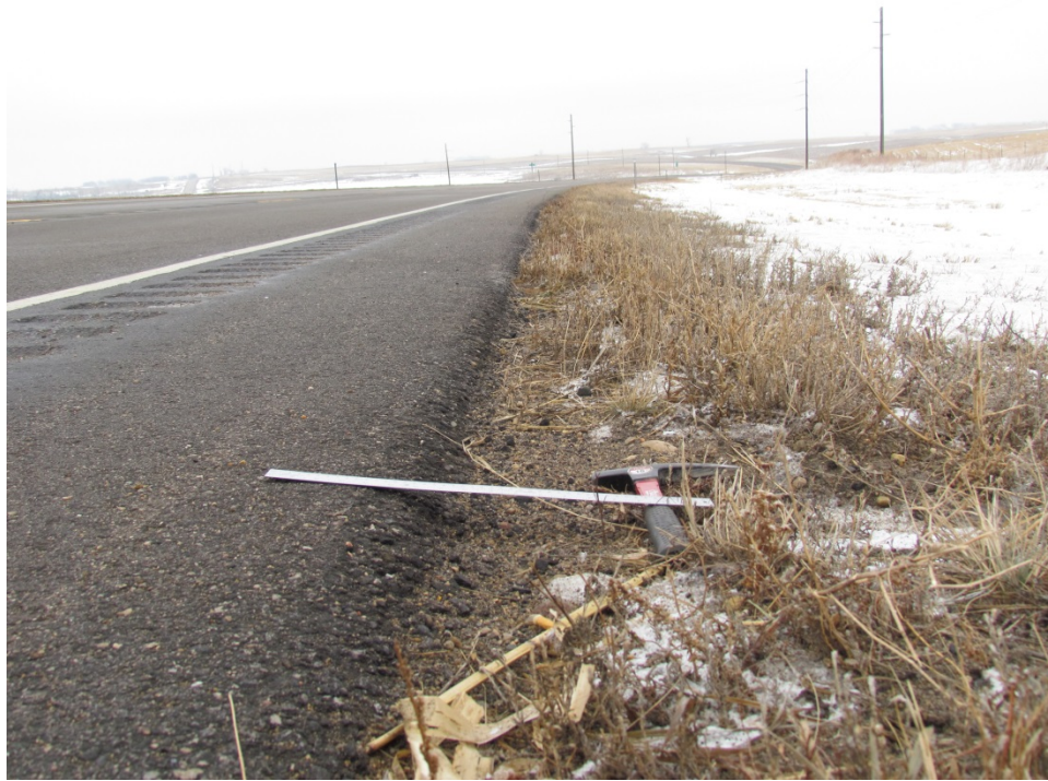
Photo 30: (ND 46, RP 13) - 30° Safety Edge 2014 South Shoulder Facing East
