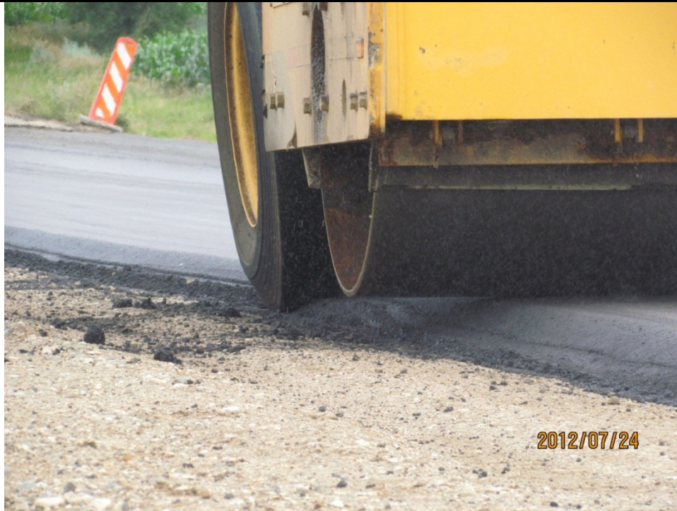
Photo 3: Breakdown roller compacting the safety edge.
