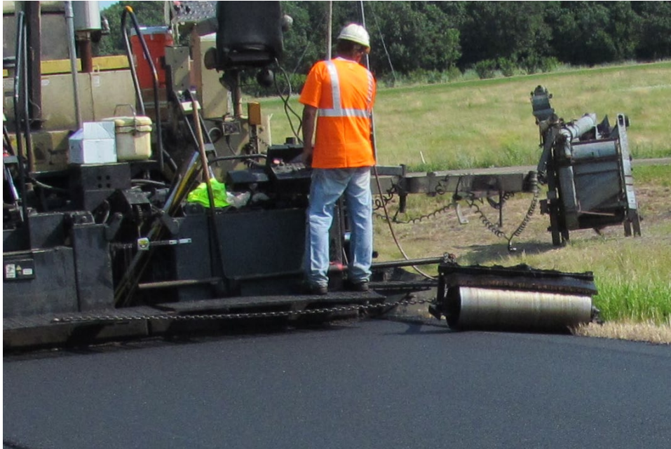
Photo 1 : Typical ND contractor slough box paving operation.
