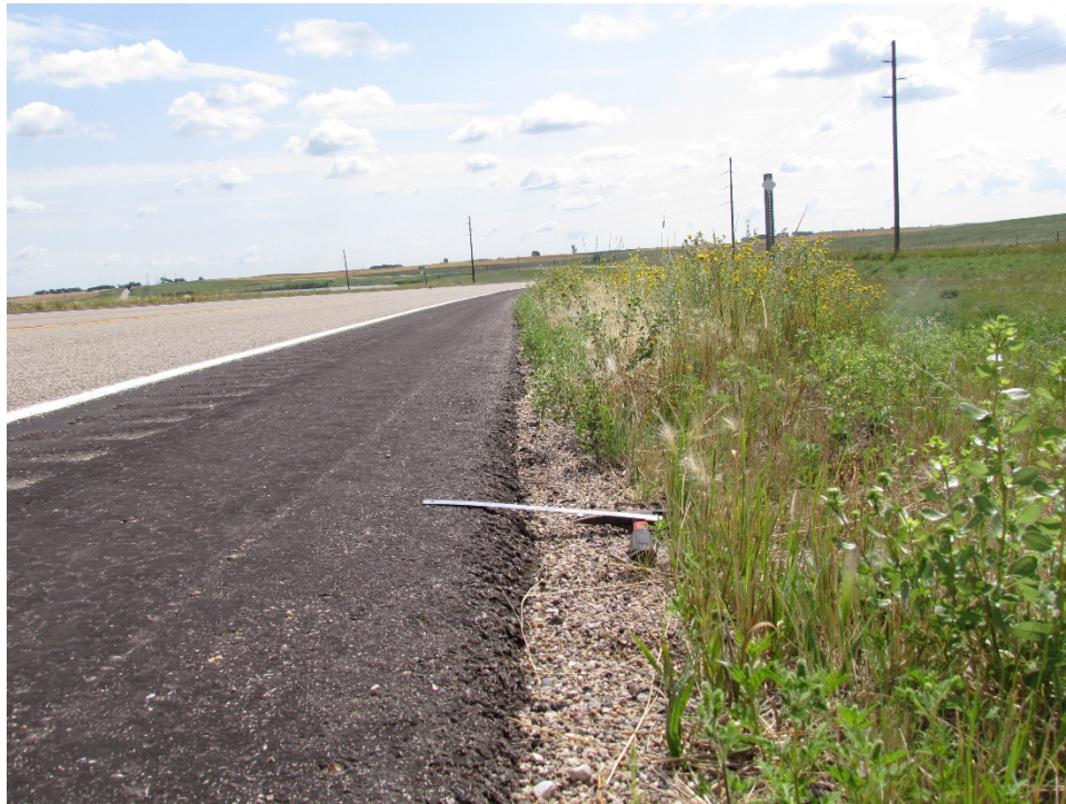
Photo 44: (ND 46, RP 13) - 30° Safety Edge 2014 South Shoulder Facing East
