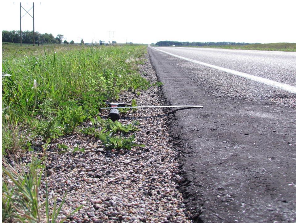
Photo 41: (ND 11, RP 45) - 30° Safety Edge 2014 North Shoulder Facing East
