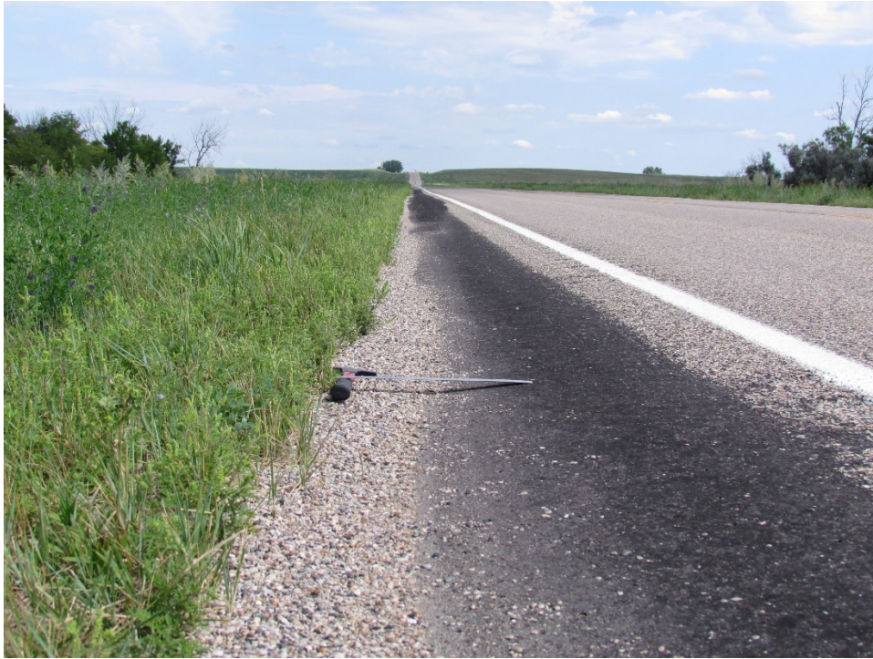
Photo 50: (ND 30, RP 7) Control 30° Contractor Constructed West Shoulder Facing North
