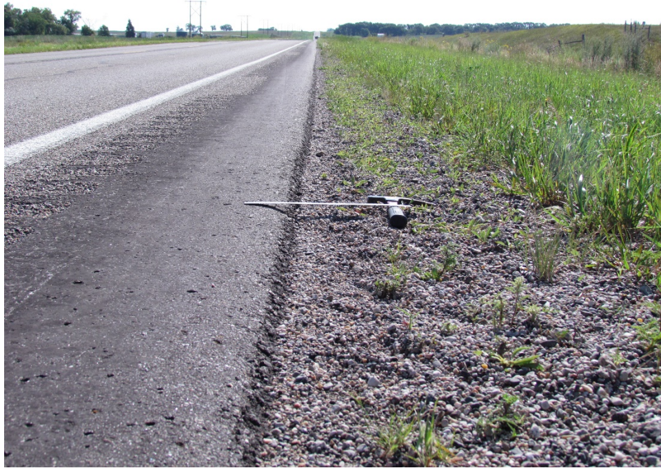
Photo 40: (ND 11, RP 45) - 30° Safety Edge 2014 South Shoulder Facing East
