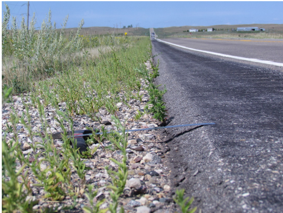
Photo 43 :( ND 13, RP 249) - 30° Safety Edge 2014 South Shoulder Facing West
