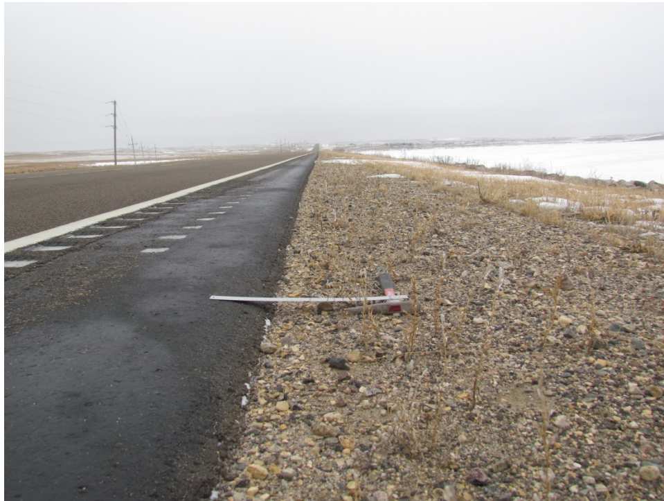
Photo 28 :( ND 13, RP 249) - 30° Safety Edge 2014 North Shoulder Facing West
