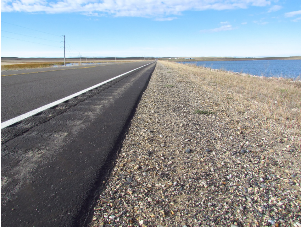
Photo 103 :( ND 13, RP 249) - 30° Safety Edge North Shoulder Facing West
