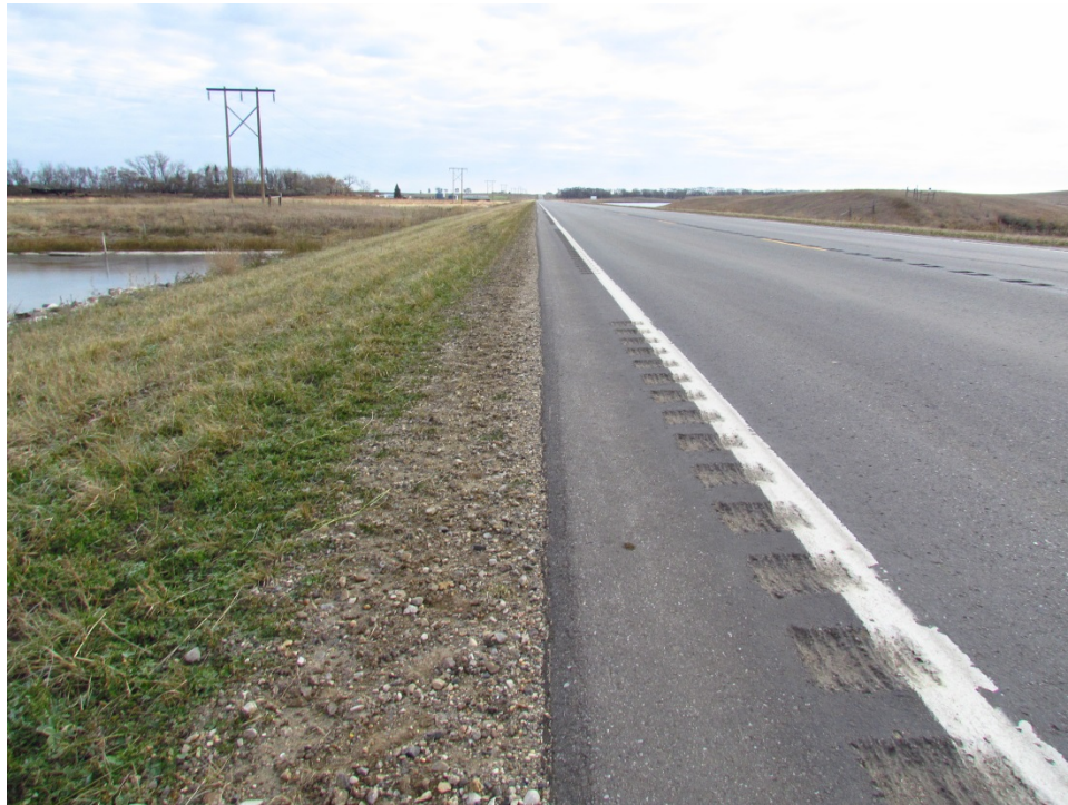
Photo 81: (ND 11, RP 45) - 30° Safety Edge North Shoulder Facing East
