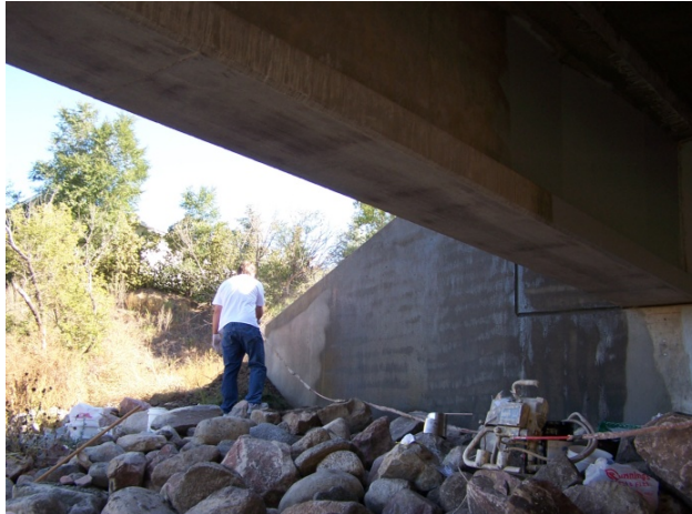
Photo 17: Spraying Top Coat on wing wall
