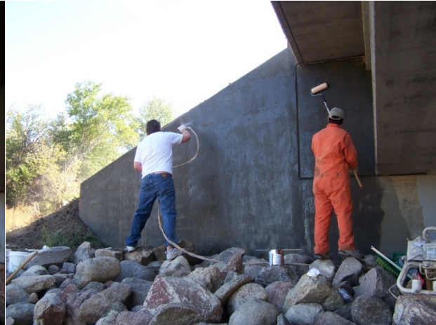
Photo 18: Backrolling wing wall
