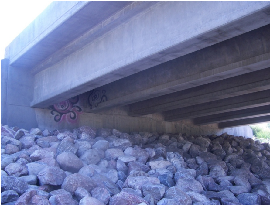
Photo 2: Heart River Bridge: East Abutment
