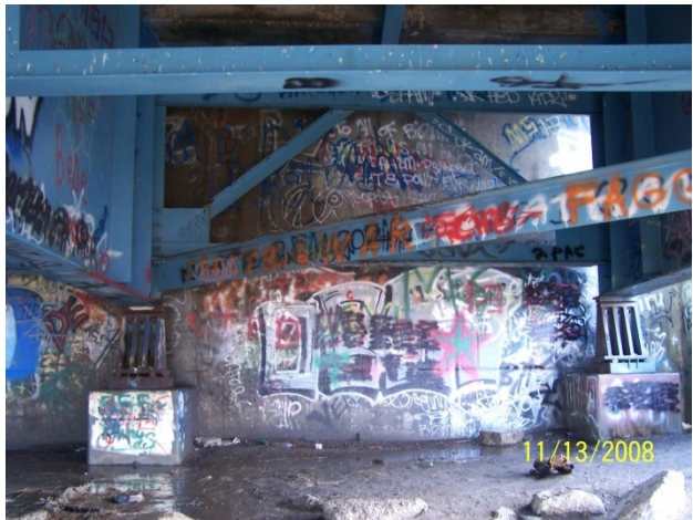
Photo 33: Portion of Expressway Bridge abutment
