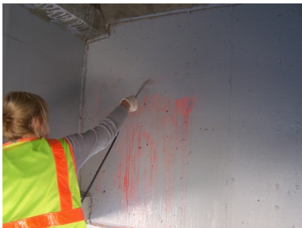
Photo 28: Rinsing with low-pressure
