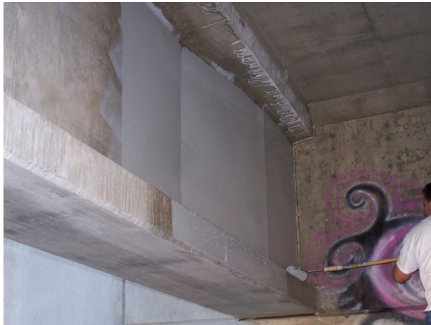
Photo 12: Rolling on pigmented coat
