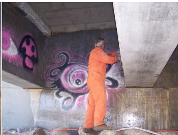
Photo 7: Backrolling base coat
