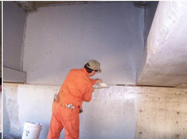
Photo 13: Touching up Joint
