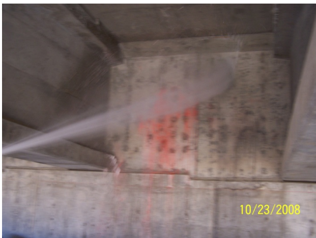
Photo 31: Rinsing with moderately pressurized water
