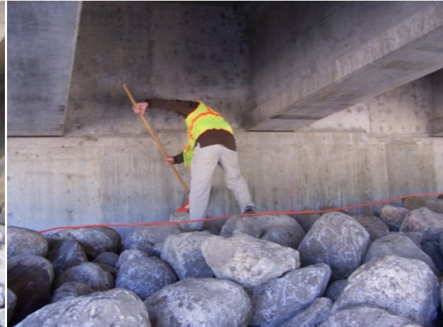
Photo 4: Brooming off debris from abutment
