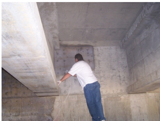
Photo 6: Base coat application
