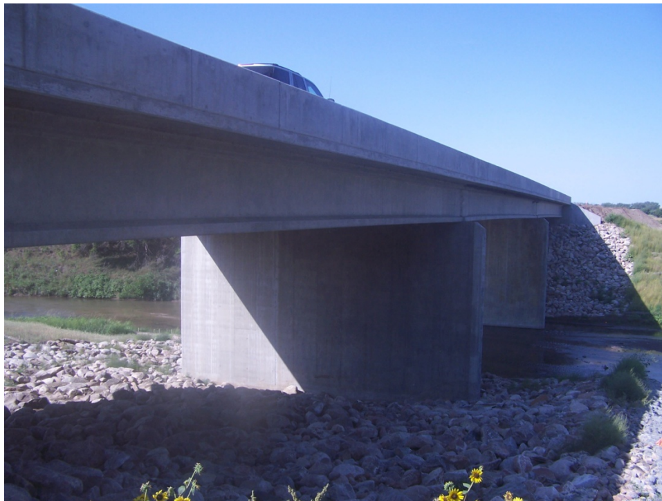
Photo 1: Heart River Bridge, looking West
