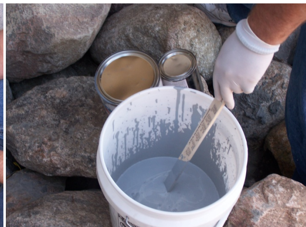
Photo 11: Mixing "Part A" & "Part B"
