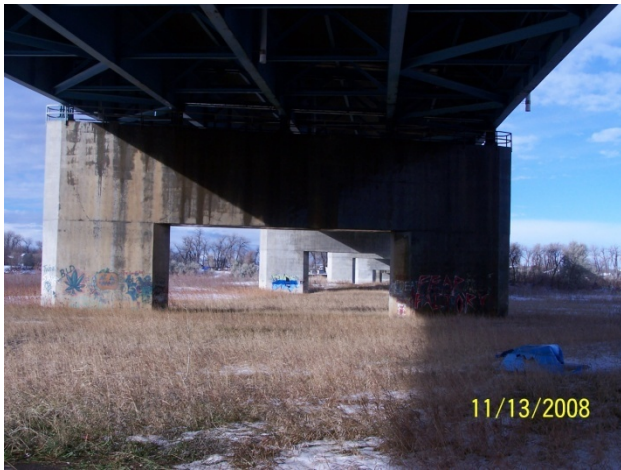
Photo 34: Expressway Bridge piers
