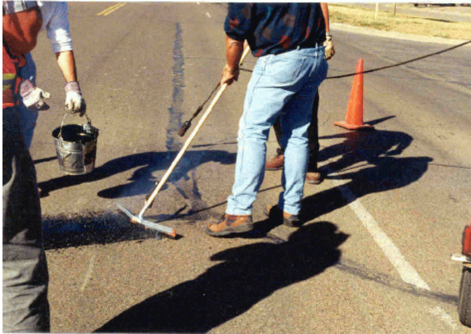
Photo 4 -- Preheating surface with torch and new straight-edge
