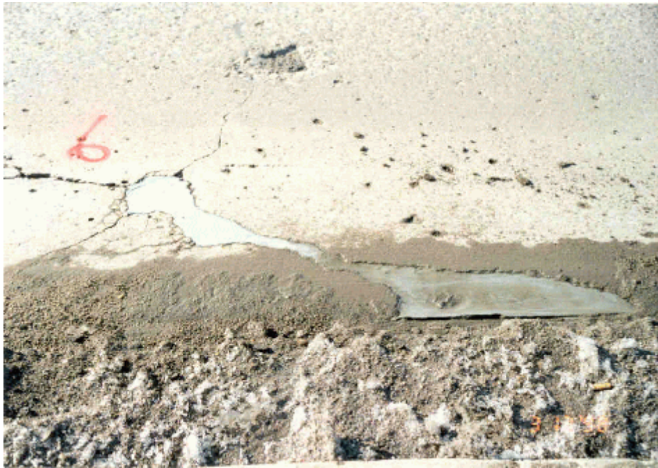
Photo 15 -- Cold weather repair material --looks good
