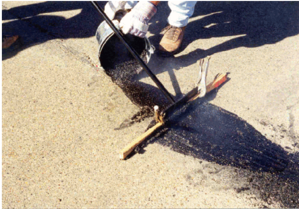
Photo 2 -- Pouring poly-patch material and straight-edging
