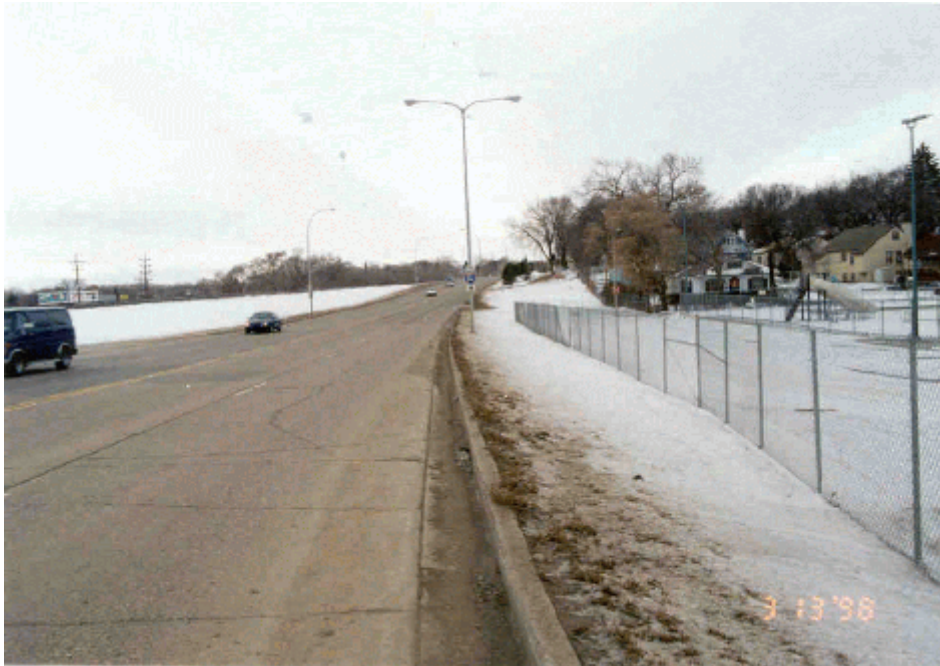
Photo 13 -- Overview of test section--driving lane
