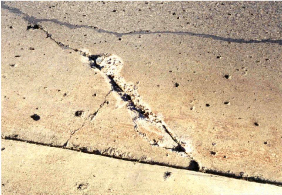
Photo 10 --Spall area cleaned by sandblasting and high pressure air
