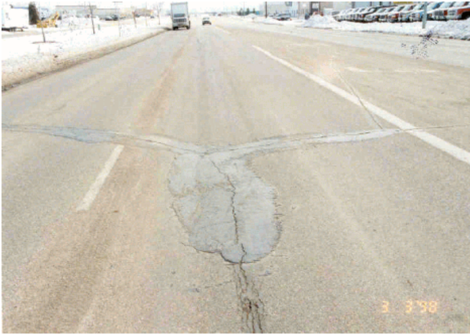
Photo 8 -- Poly-patch material in good condition
