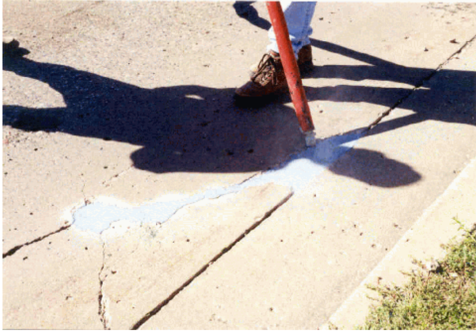
Photo 11 -- Applying final lift of spall repair material
