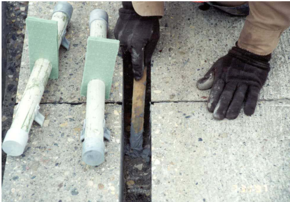
Photo 3 - View of caulking process.
