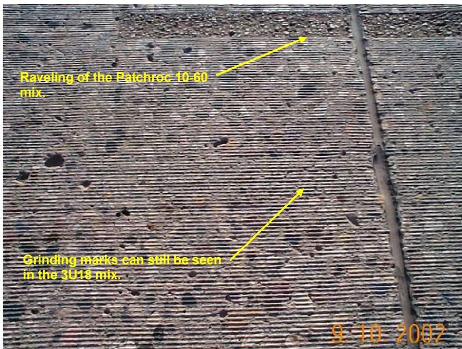
Photo 17 - Durability of both mixes.
