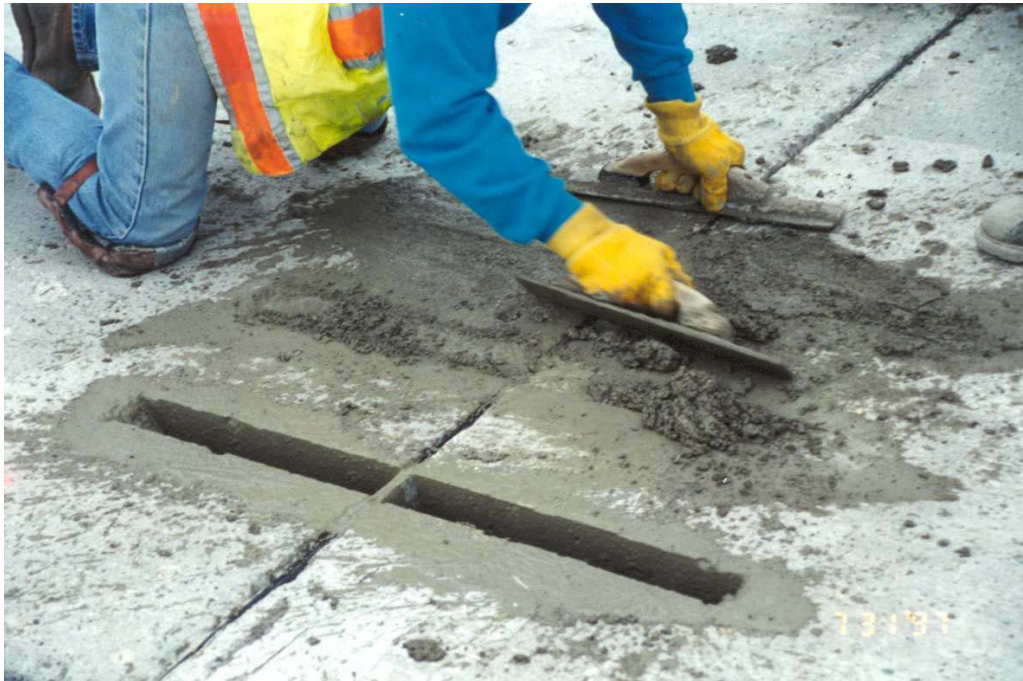
Photo 10 - View of the 3U18 patch mix being troweled and finished.
