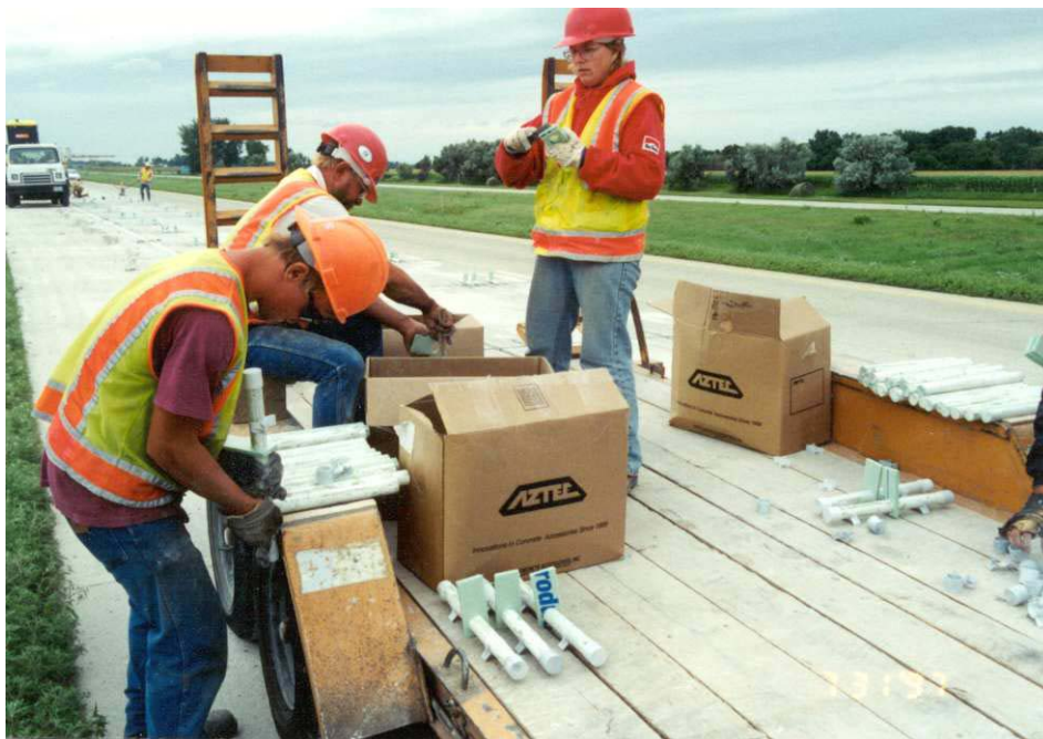
Photo 5 - View of the core board fabrication process.
