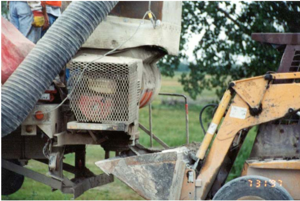
Photo 7 - View of the batch mix unit used to batch the 3U18 patch mix.
