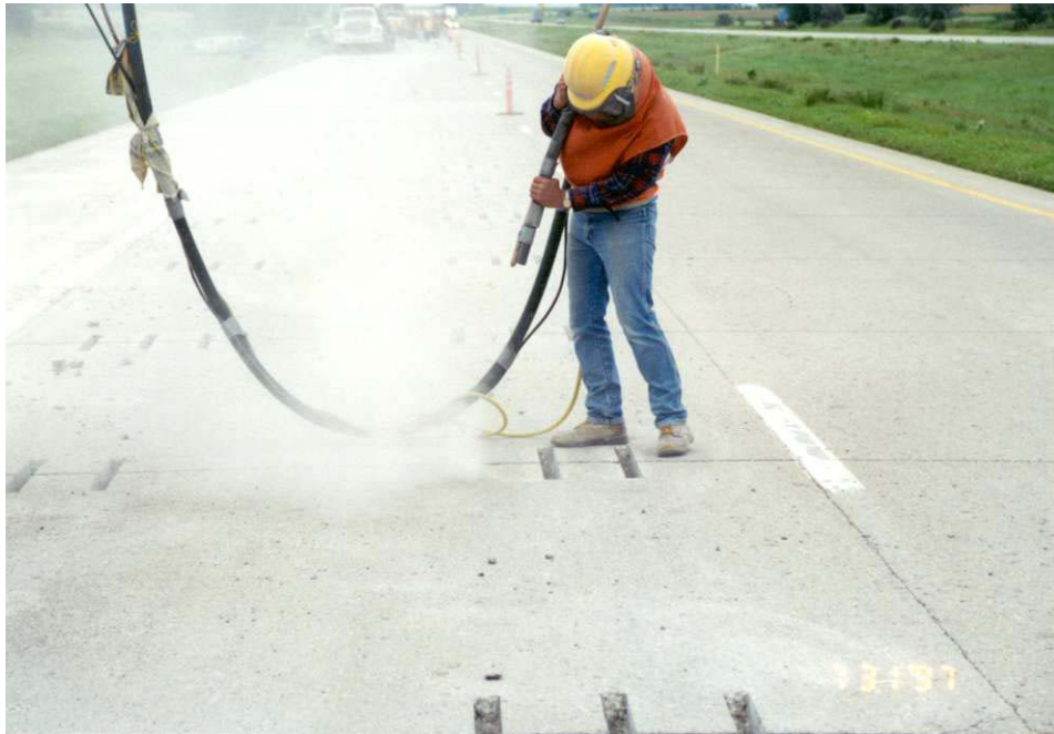
Photo 2 - View of the sandblasting process.
