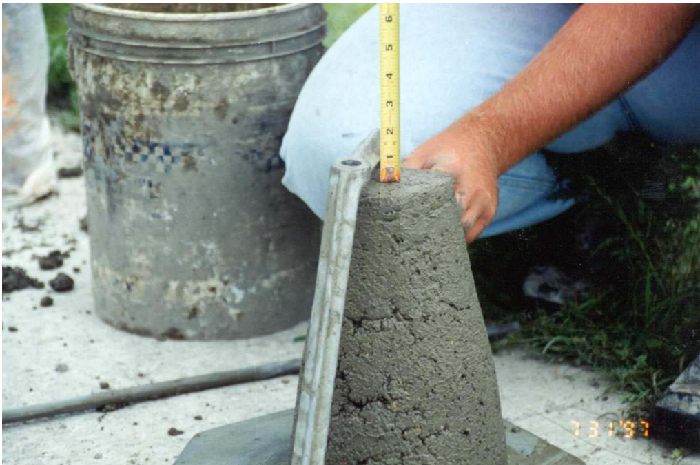
Photo 8 - View of a slump test being performed on the 3U18 mix.
