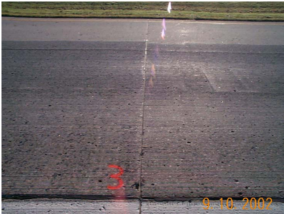
Photo 15 - Dowel bar slots containing 3U18.
