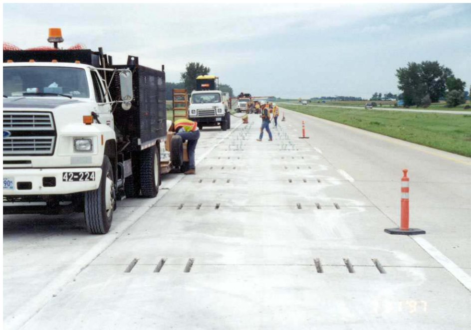
Photo 1 - Overview of the dowel bar retrofit operation.
