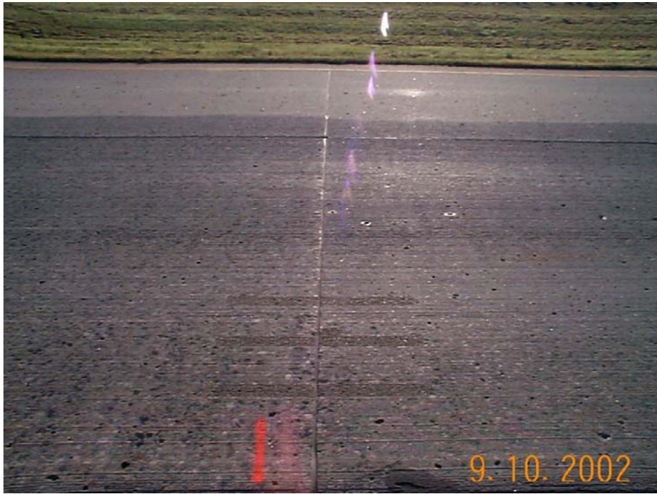
Photo 14 - Dowel bar slots containing Patchroc 10-60.
