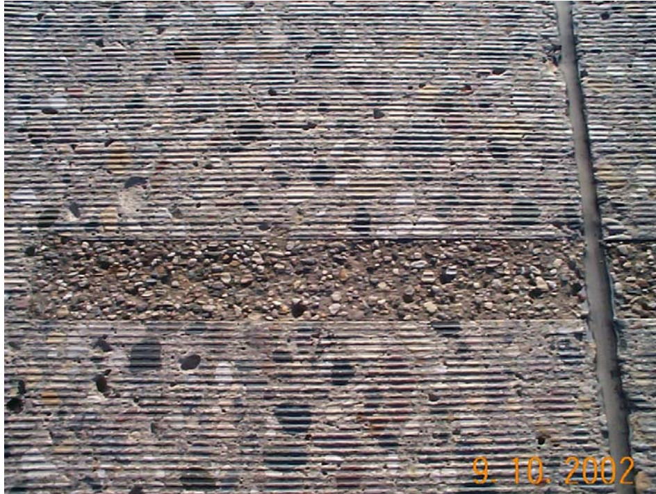
Photo 18 - Close up view of the Patchroc 10-60 mix shown in photo 17.
