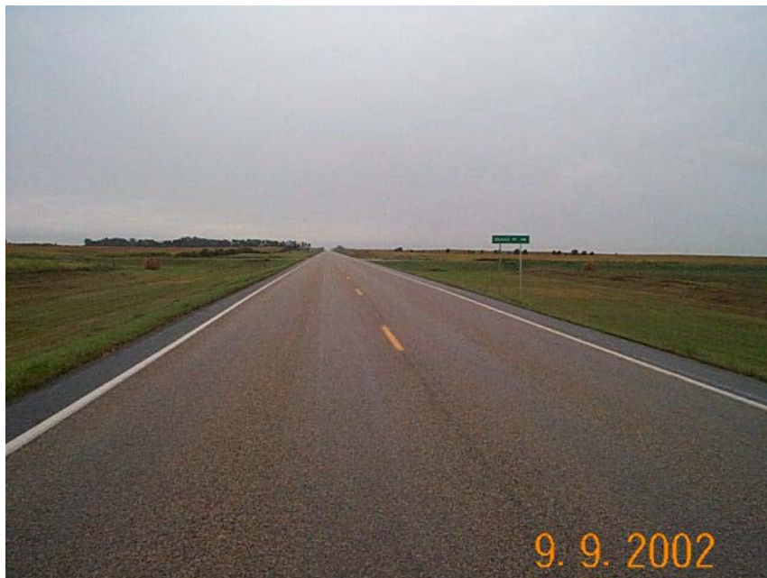
Photo 11 - Base section stabilized with cement, looking south.
