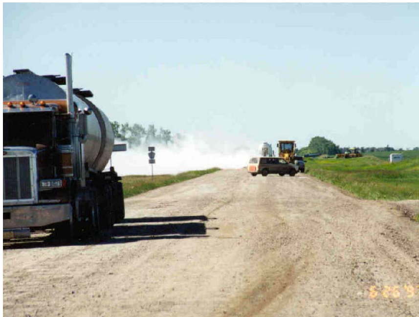
Photo 9 - Note the dust created during the blending operation of the lime section.
