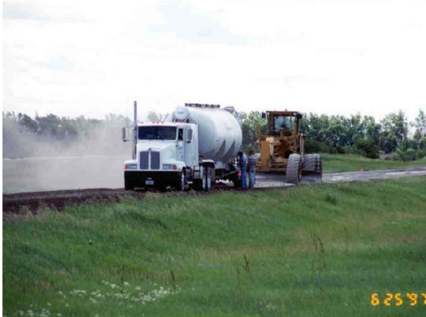
Photo 2 - Placing cement on blended base.
