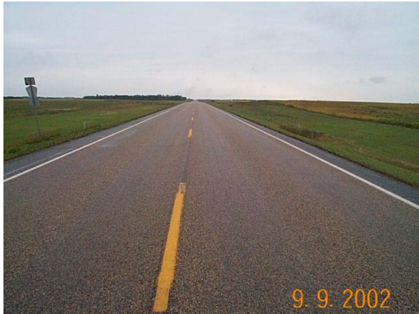
Photo 12 - Base stabilized with Consolid, looking north.
