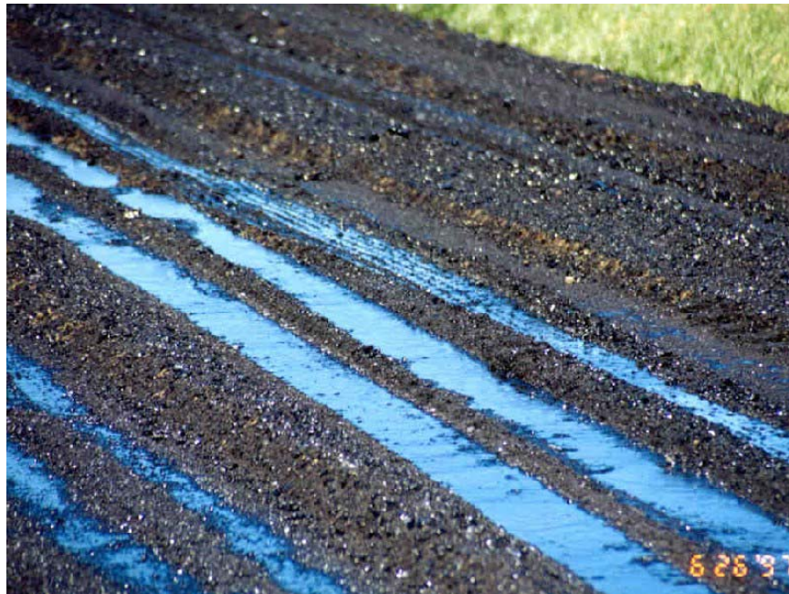
Photo 5 - Consolid after laydown.
