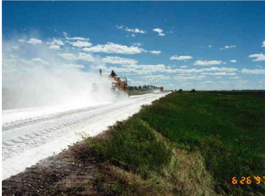
Photo 8 - Blending lime into the blended base.
