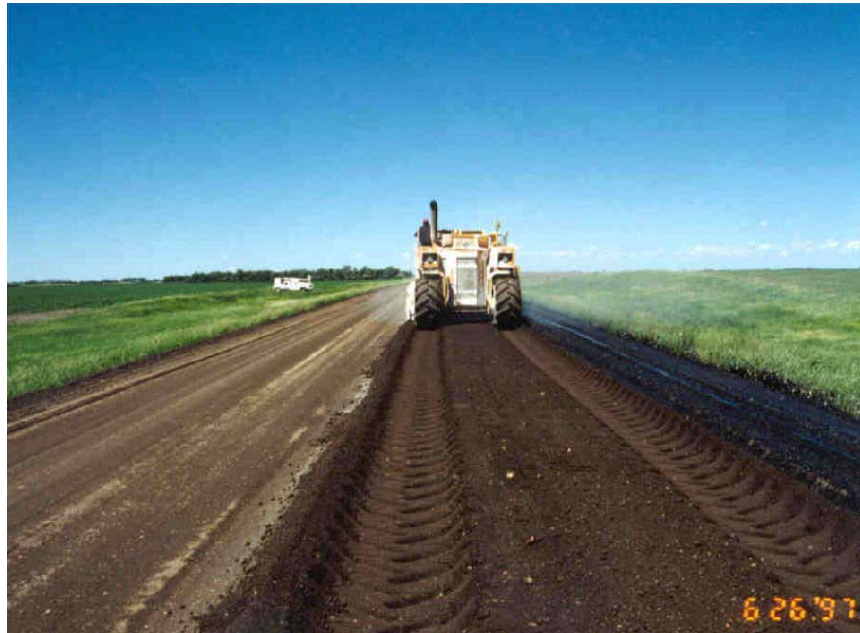
Photo 6 - Blending Consolid into blended base.
