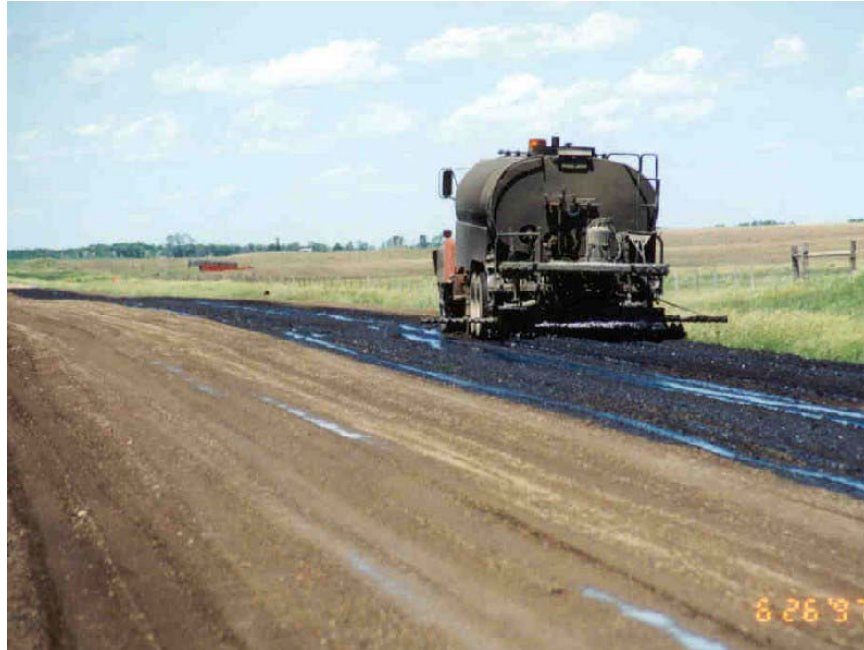
Photo 4 - Placing Consolid on blended base.
