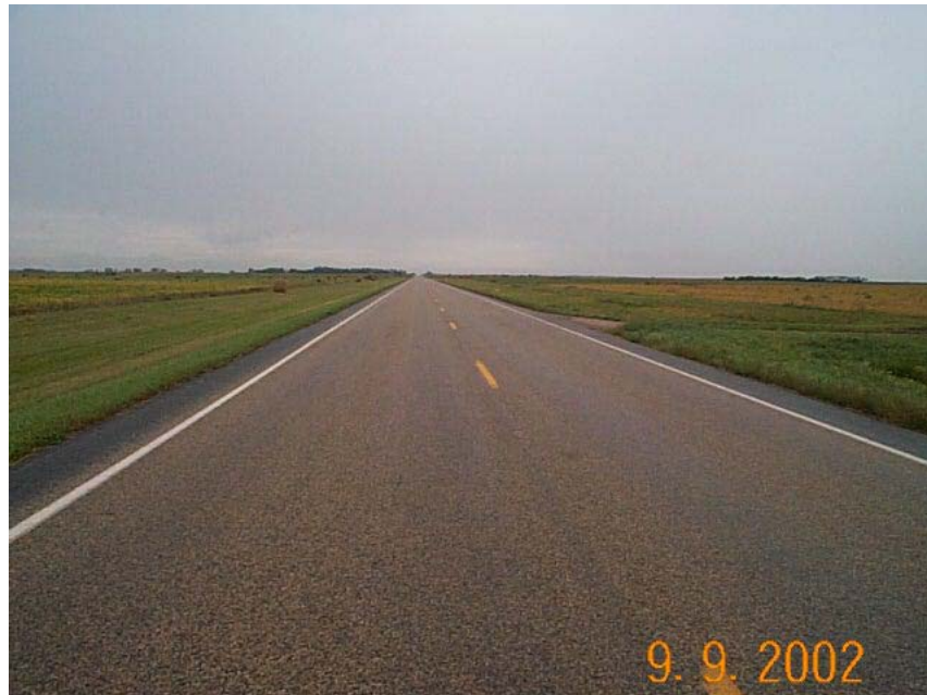
Photo 13 - Base section with no stabilization, looking south.
