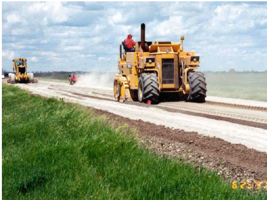
Photo 3 - Blending cement into blended base.
