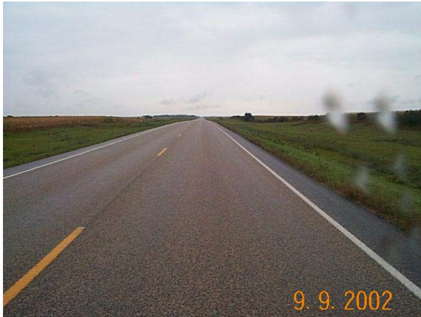
Photo 10 - Base section stabilized with lime, looking north.
