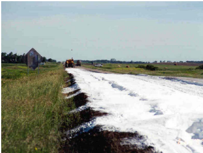
Photo 7 - Lime after laydown.
