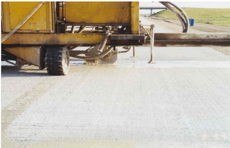
Photo 6 - Sawing process as it finishes from right to left.
