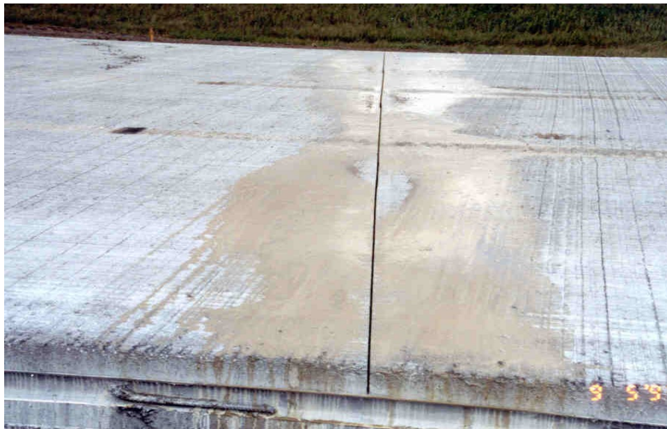
Photo 2 - Typical sawed joint.
