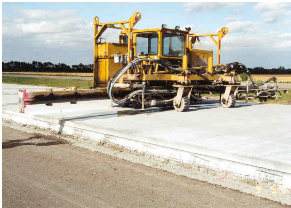
Photo 1 - Typical gang sawing machine used on project IM-6-029(027)161 in the Grand Forks District.
