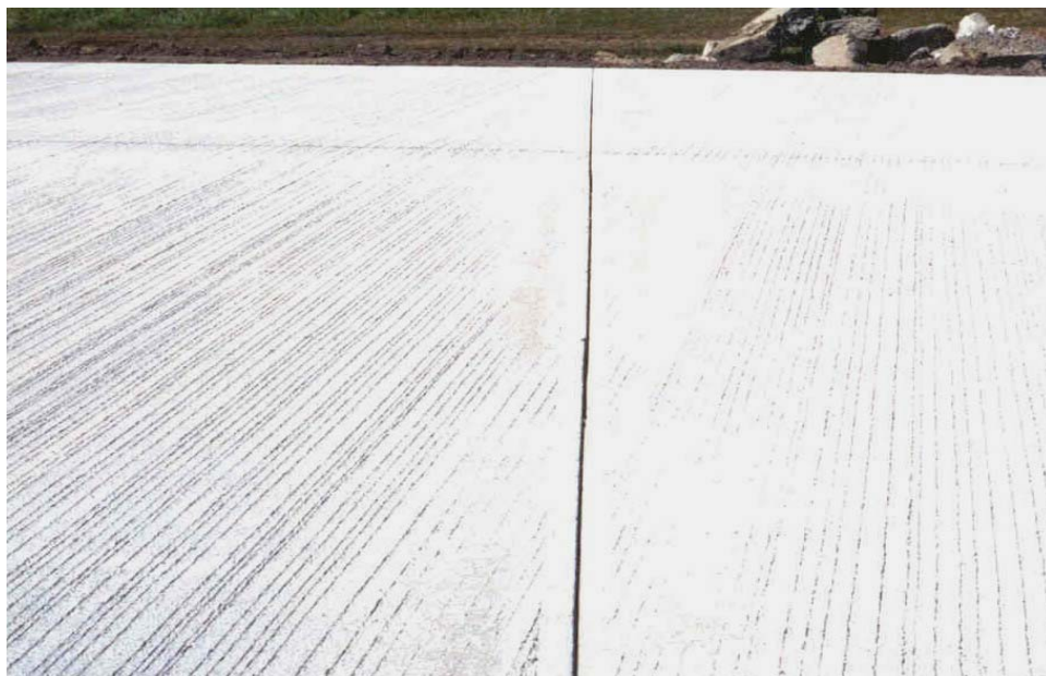
Photo 9 - Typical unsealed joint.
