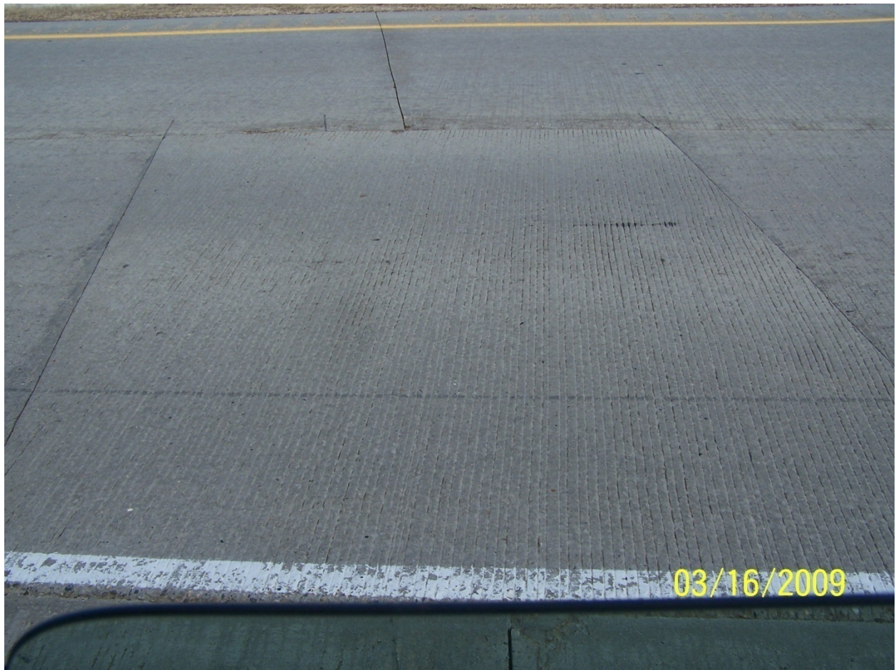
Photo 26 – Photo of repaired joint.
