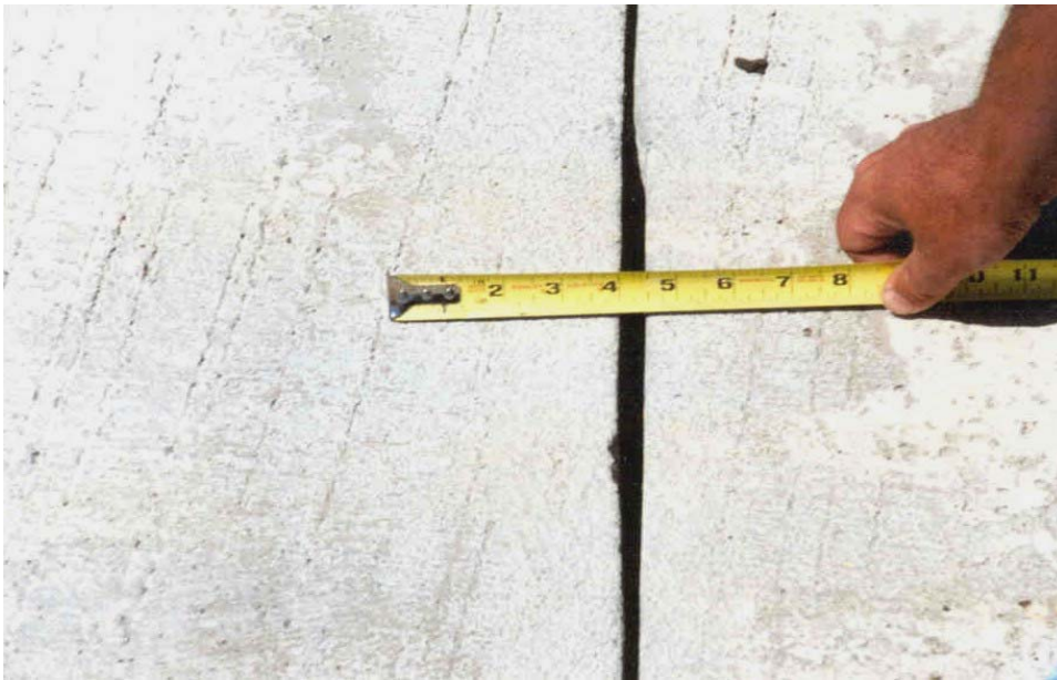
Photo 10 - Close-up view of an extra wide segment.
