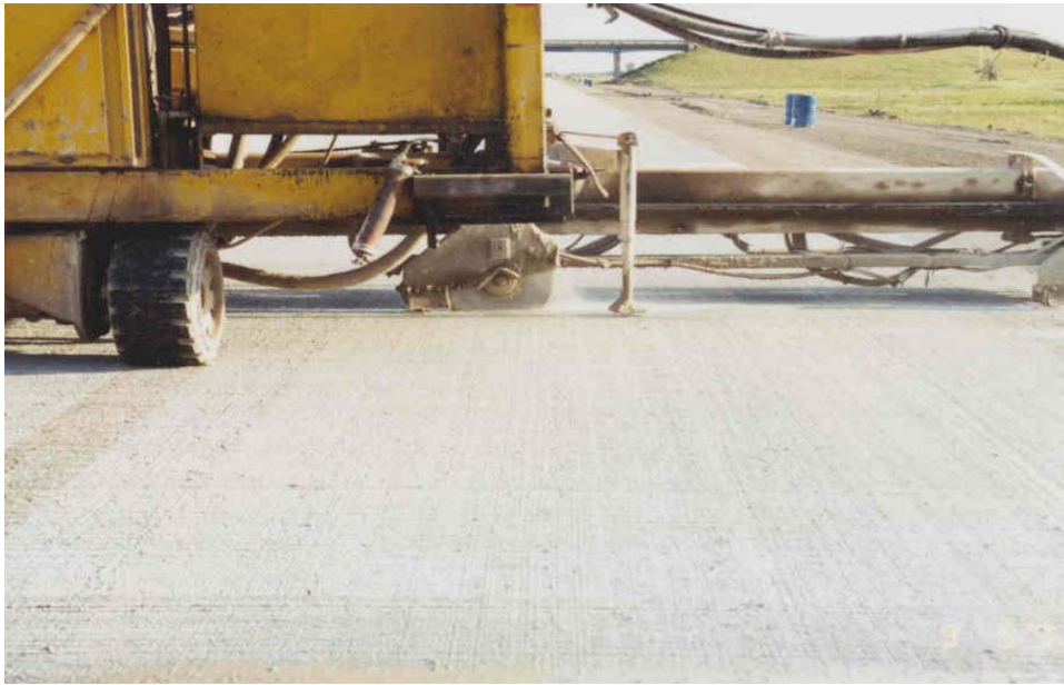
Photo 5 - Sawing process as it commences from right to left.
