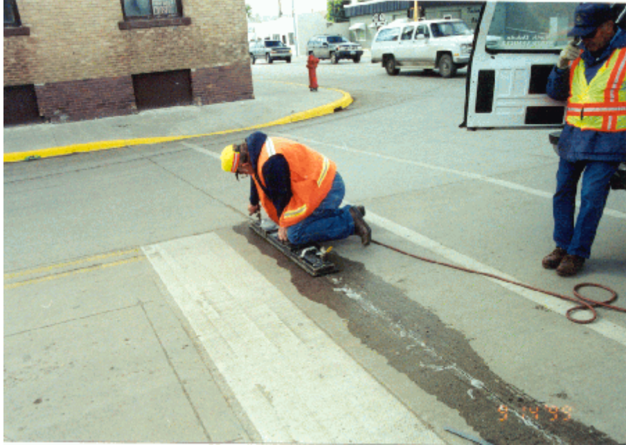
Photo 2: I - Vac test.
