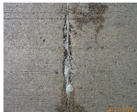
Photo 5 Typical Joint Close-up.
