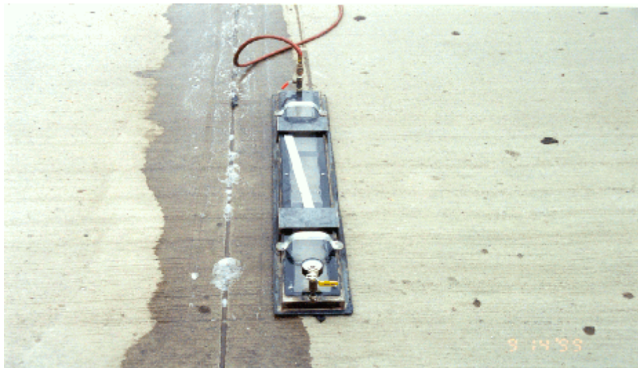
Photo 1: I-Vac testing chamber and leaking areas.
