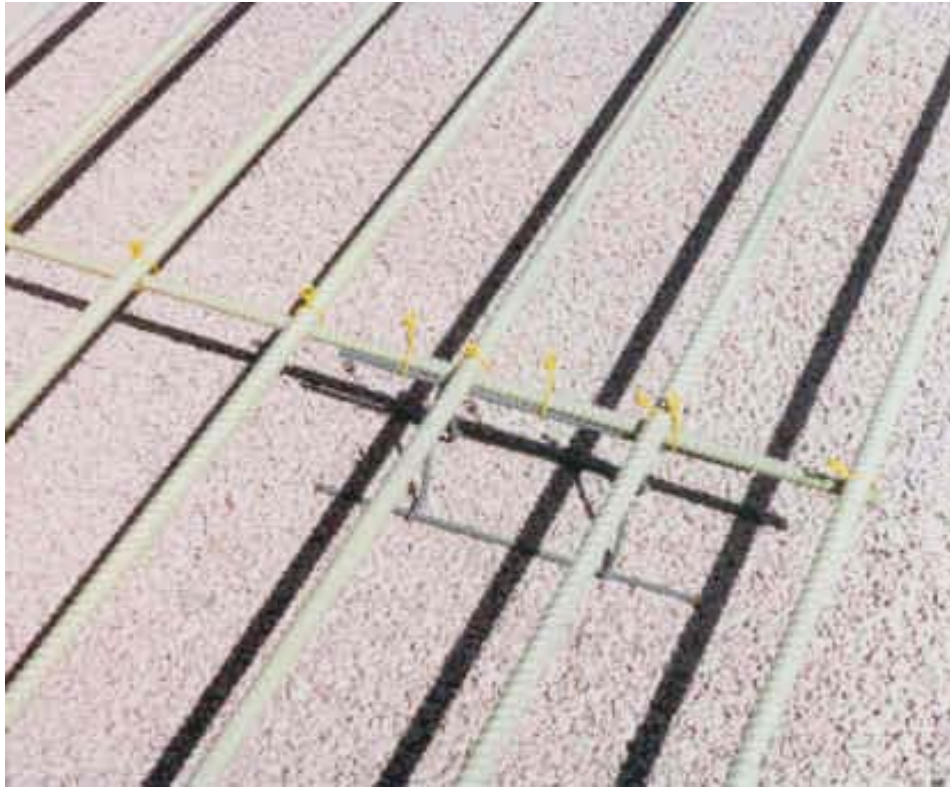
Photo 2 – View of finished product placed and fastened.
