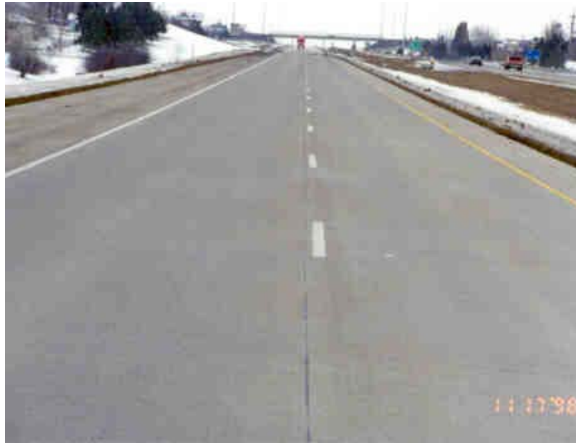
Photo 3 – Depicts an overall view of the test section looking east.
