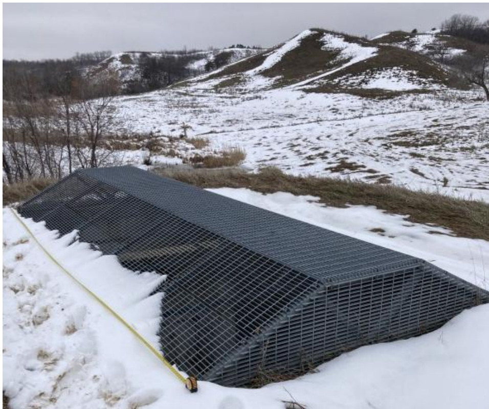
Figure 28, Sawyer Flood Control Structure
