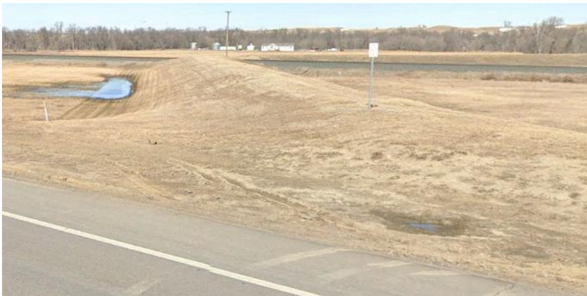
Figure 25, Velva Flood Protection Levee
