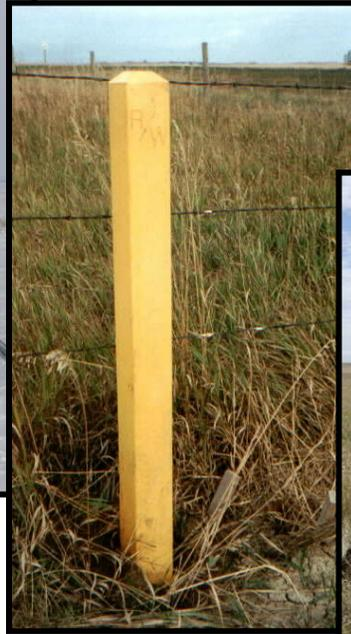
**Plastic R/W Marker**
