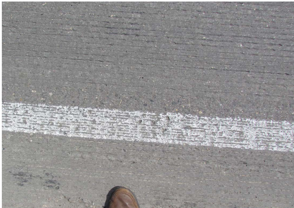
Photo 6 – White Water-based Paint Southbound – Standard Paint – 6/3/14
