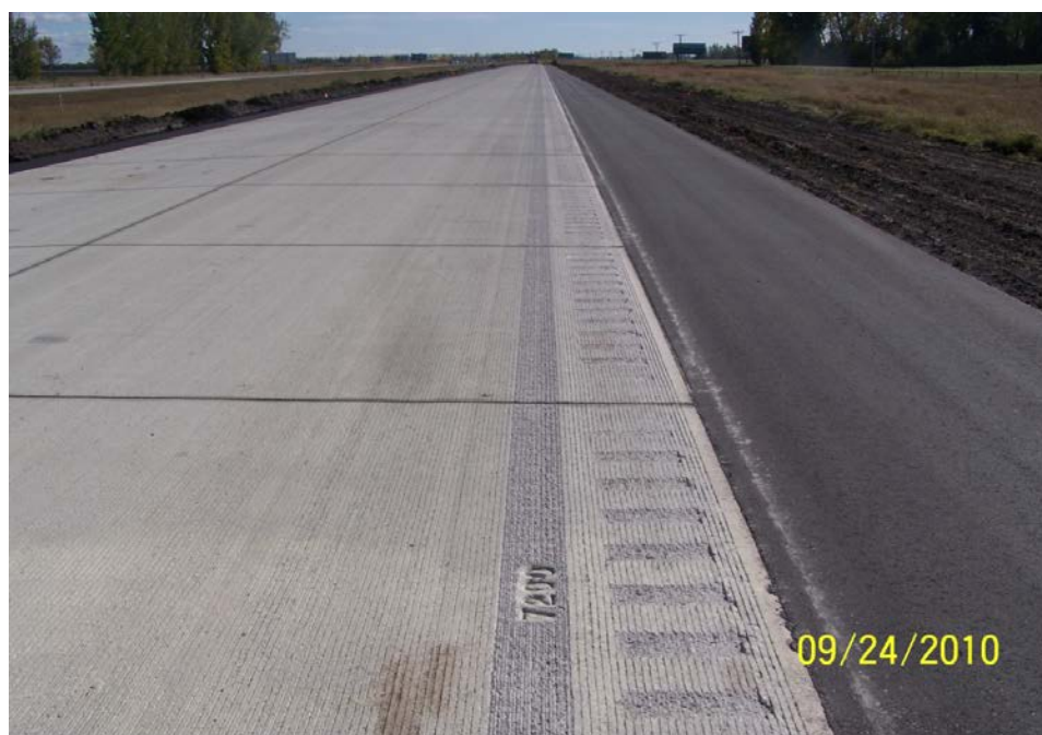
Photo 1 : Cure Removed Prior to Painting
