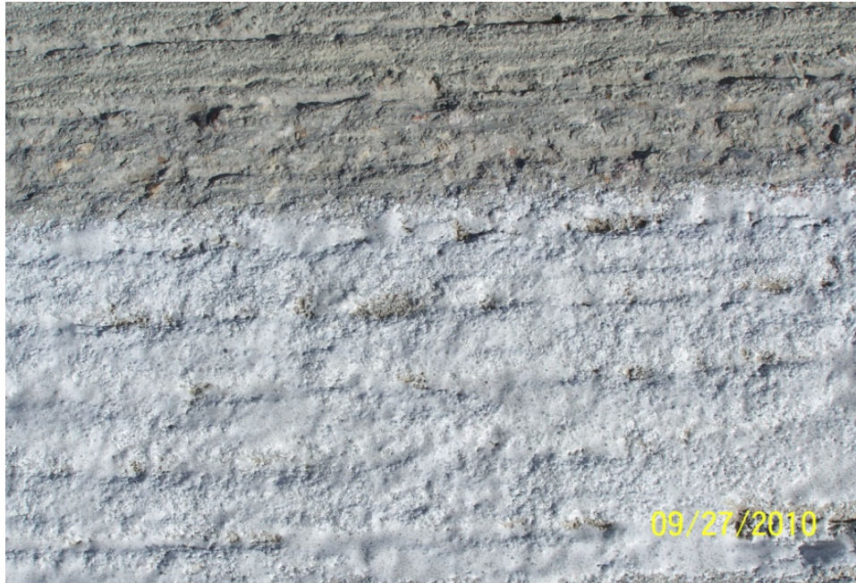
Photo 2 : Southbound White Edge-line with Standard Glass Beads
