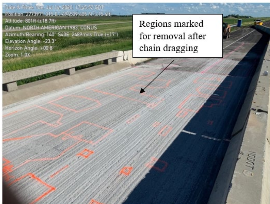
Figure 6. Forest River Bridge deck markings after chain dragging for removal of delaminated sub-surface.
