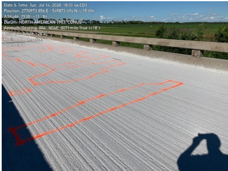
Figure 19. Park River Bridge deck markings prepared for class 2 removal after chain drag and class one removal.
