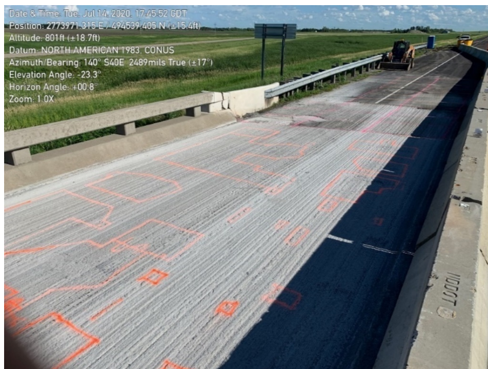
Figure 18. Forest River Bridge deck markings prepared for class 2 removal after chain drag and topping removal
