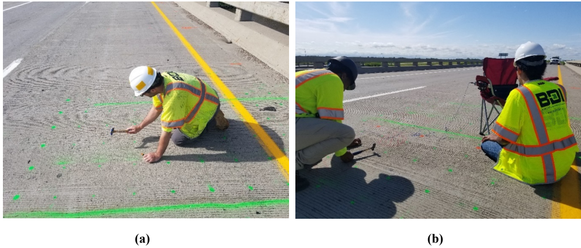
Figure 28.BDI crew member (a) preparing deck surface points for IE test (b) marking carrying out IE test on Forest River NB bridge deck.
