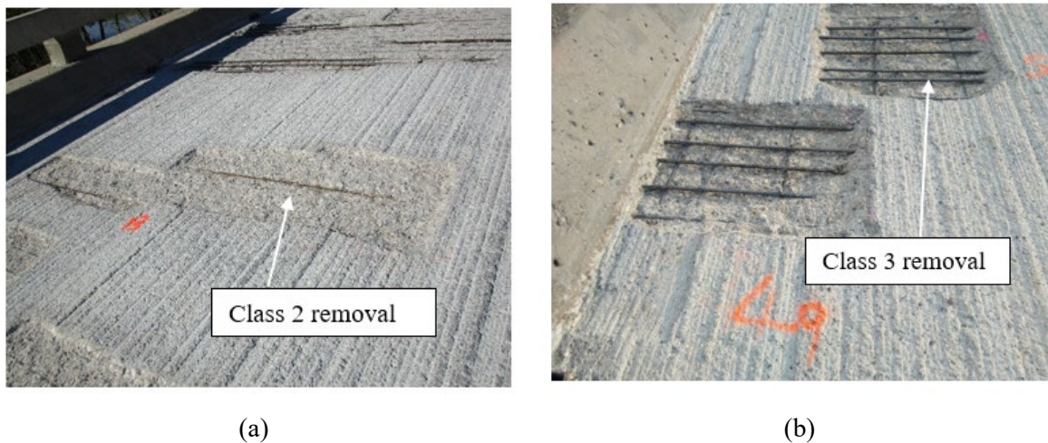
Figure 21. Image showing portion of (a) class 2 and (b) class 3 removal for Park River south Bound.
