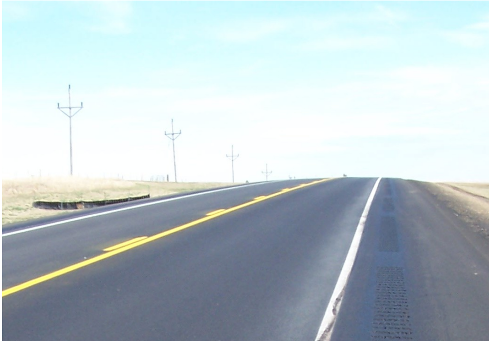
Photo 5 – US 12 just after placement of pavement markings and shoulder rumble strips.
