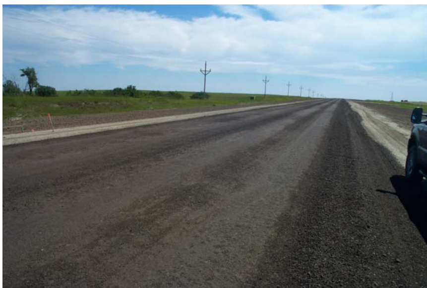
Photo 4 – Test segment with salvaged HBP on top of the pavement.
