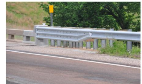
**MGS TRANSITION TO 28" GUARDRAIL:** You should transition from a 27-3/4 inch tall barrier or terminal to a 31-inch tall barrier over the span of two 12-foot, 6-inch pieces of w-beam rail. When replacing or repairing long portions of a damaged rail the new rail should be installed at the proper design height, transitioning down to the existing rail over the length of two 12 foot, 6- inch pieces of rail at either end.
