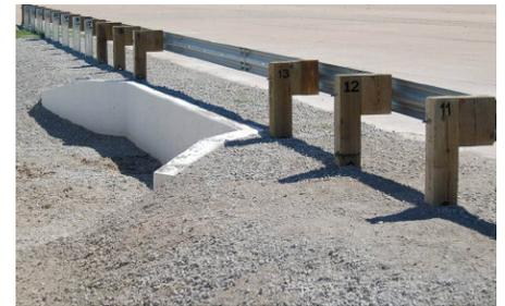
**MGS TRANSITION DESIGN:** The MGS system is compatible with most existing Thrie-beam to rigid barrier/bridge railing transition designs with the use of a non-symmetrical W-beam to Thrie beam transition section and a modified post layout. The recommended design was successfully crash-tested under MASH criteria. Refer to NDDOT Standard Drawing D764-60.
