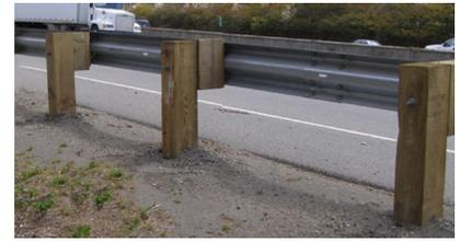
**MGS DEFLECTION:** The standard MGS (6'-3" post spacing) resulted in a somewhat increased dynamic deflection when MASH tested. Crash test with wood post resulted in a working width of 53.8 to 58.4 inches. ( Ref. FHWA letters B-230 and 230A.) (Since the NDDOT's Design Manual has not been updated for the MGS, the allowable offsets have not been found.)
