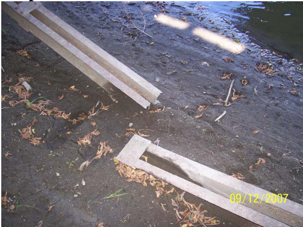
South pier crossframe – bottom strut fractured
