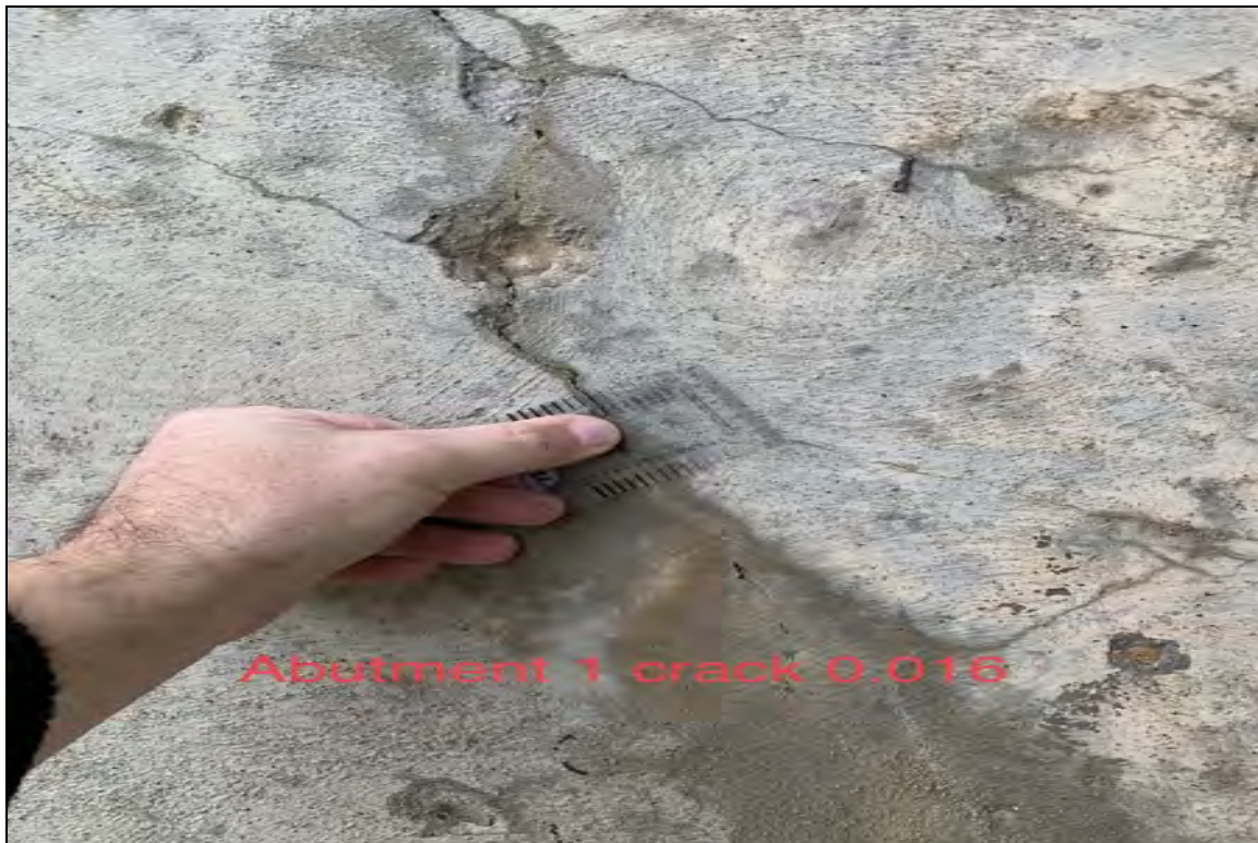
Abutment 1 crack .016
