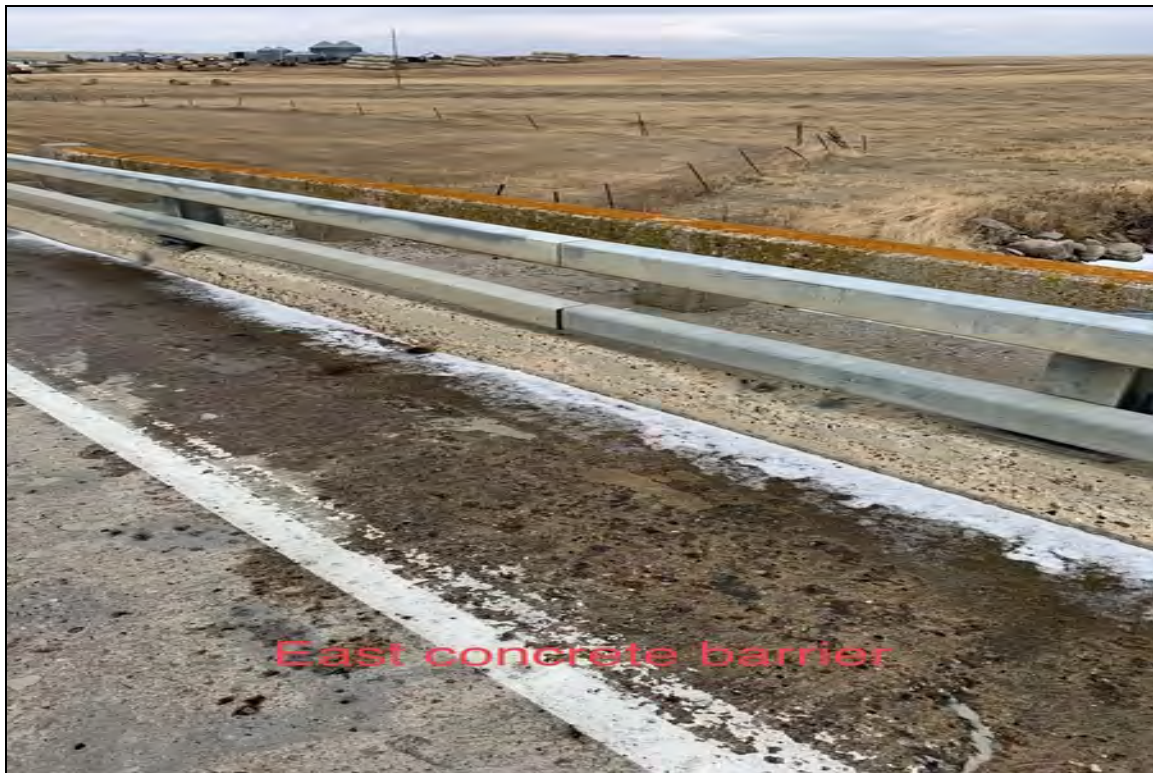
East concrete barrier
