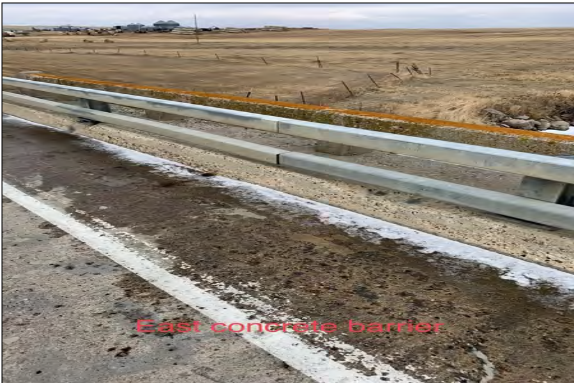
East concrete barrier
