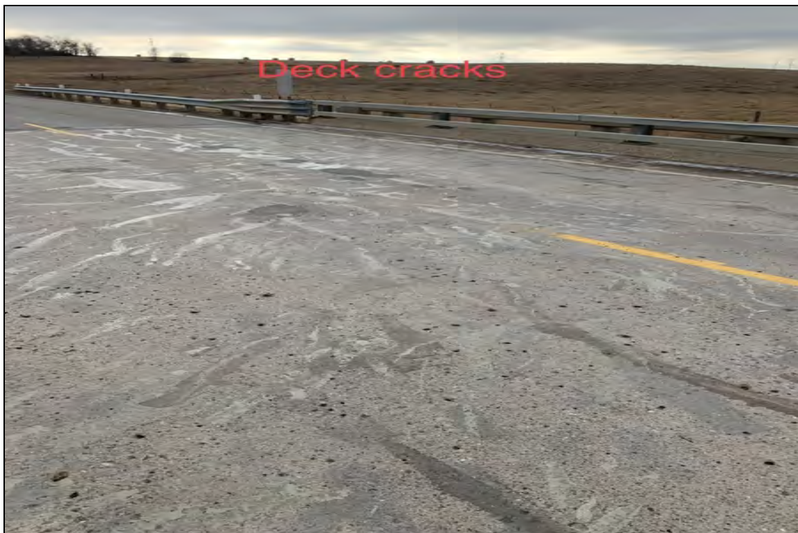
Deck cracks
