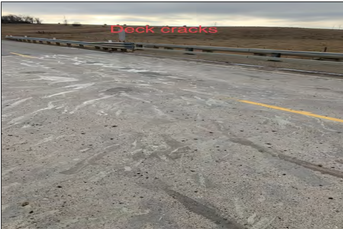
Deck cracks
