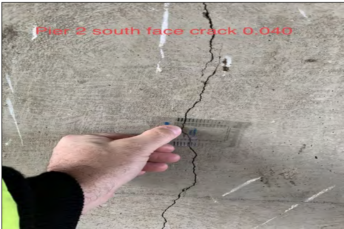
Pier 2 south face crack .040
