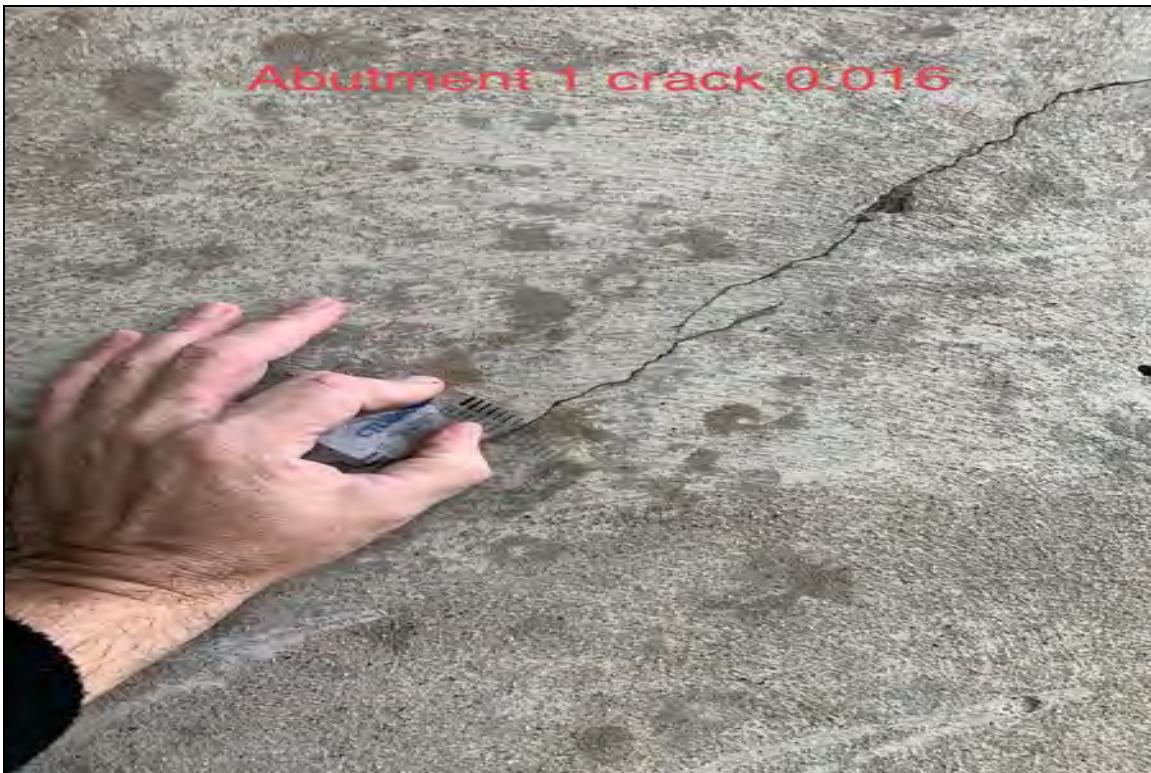
Abutment 1 crack .016
