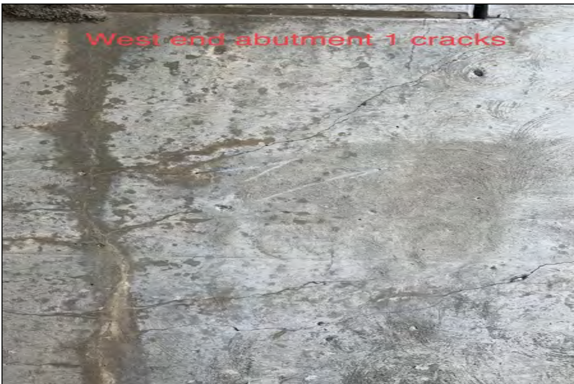
West end abutment 1 cracks
