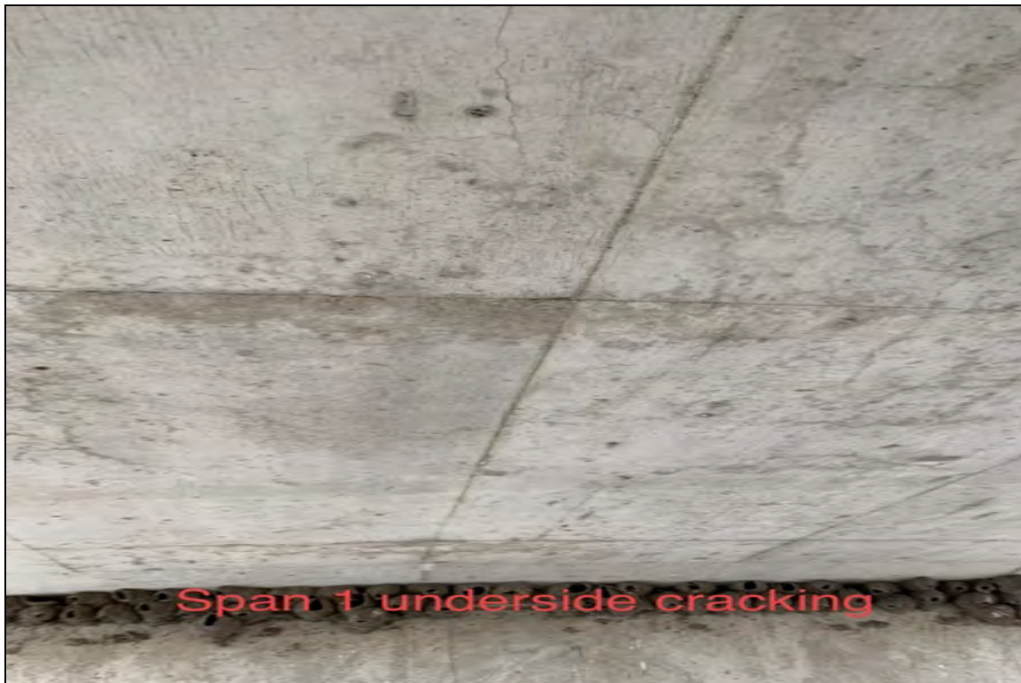
Span 1 underside deck cracking
