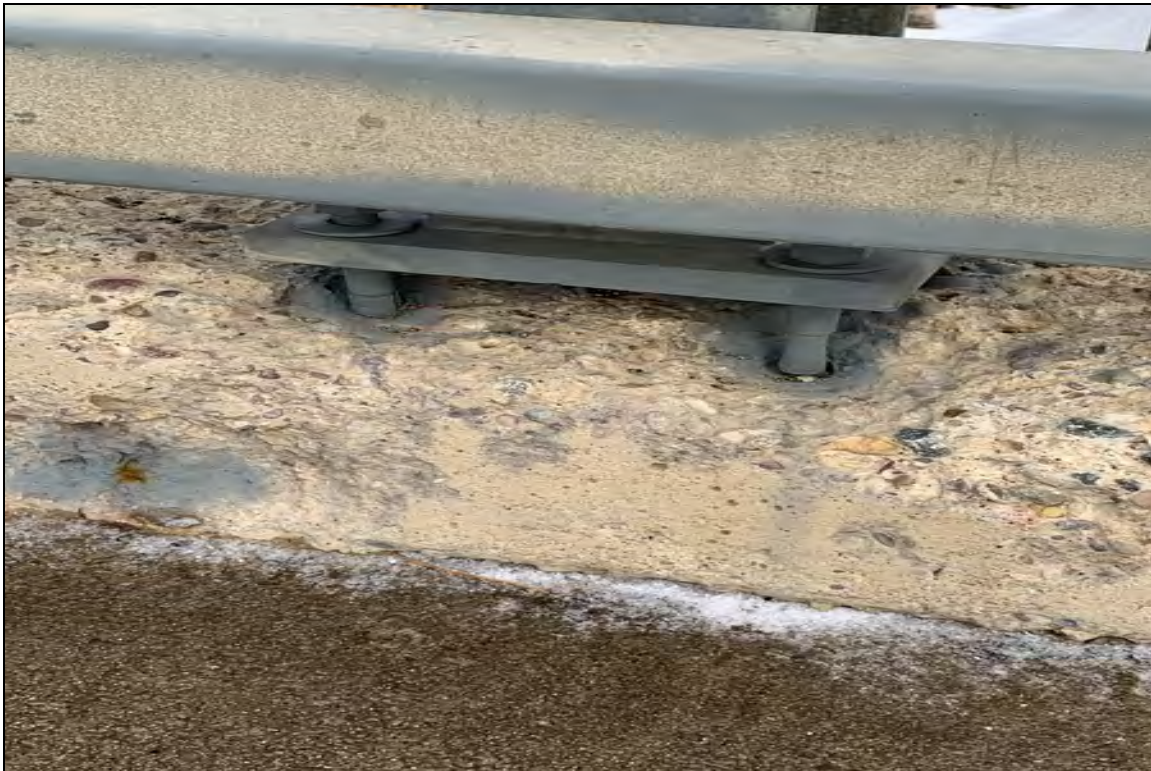
East box rail attachment
