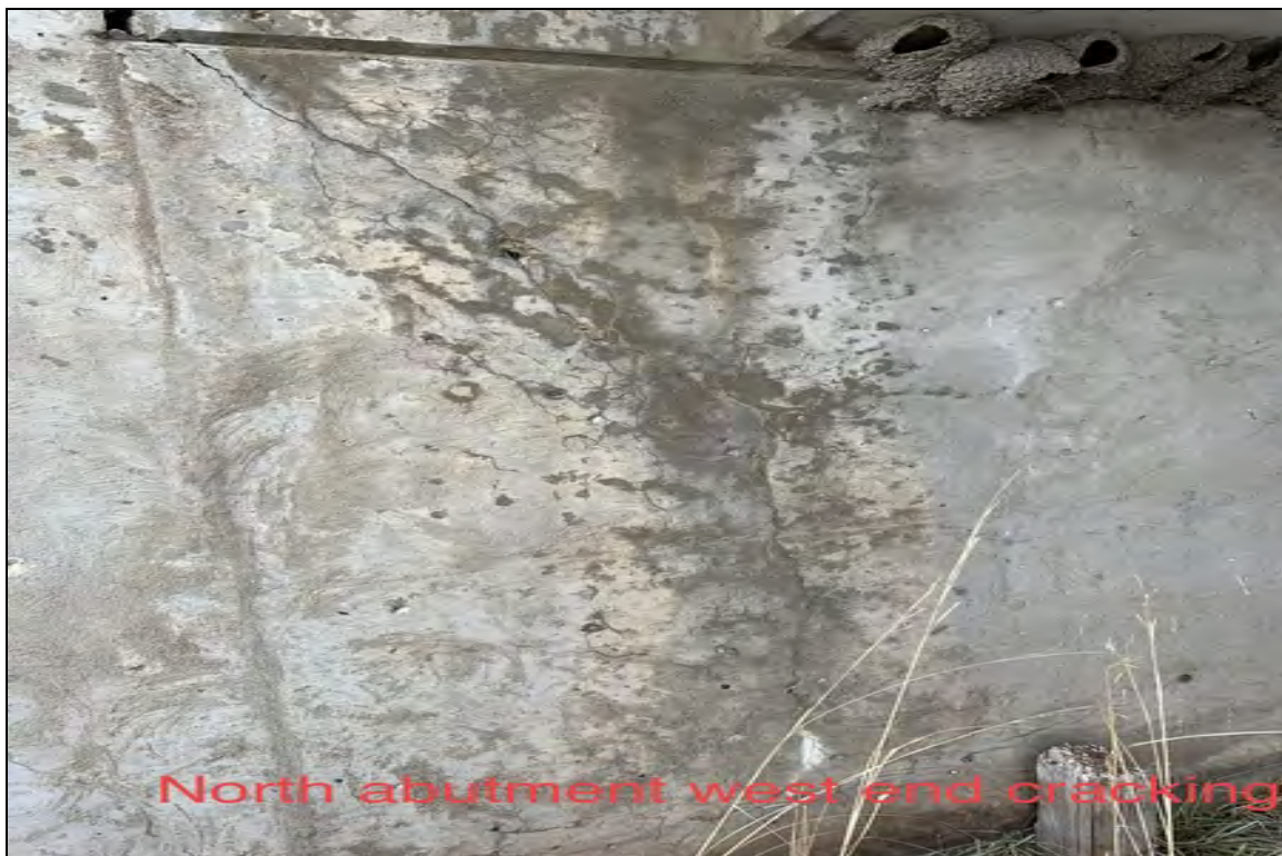
North abutment west end cracking
