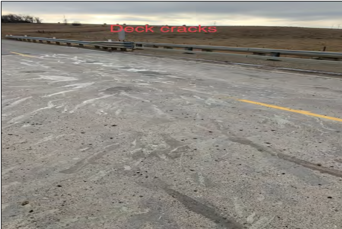
Deck cracks
