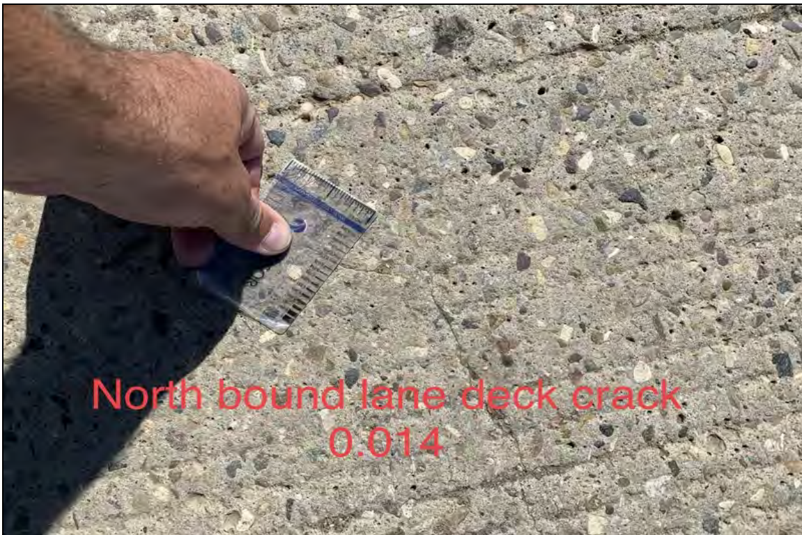
North bound deck lane crack .014
