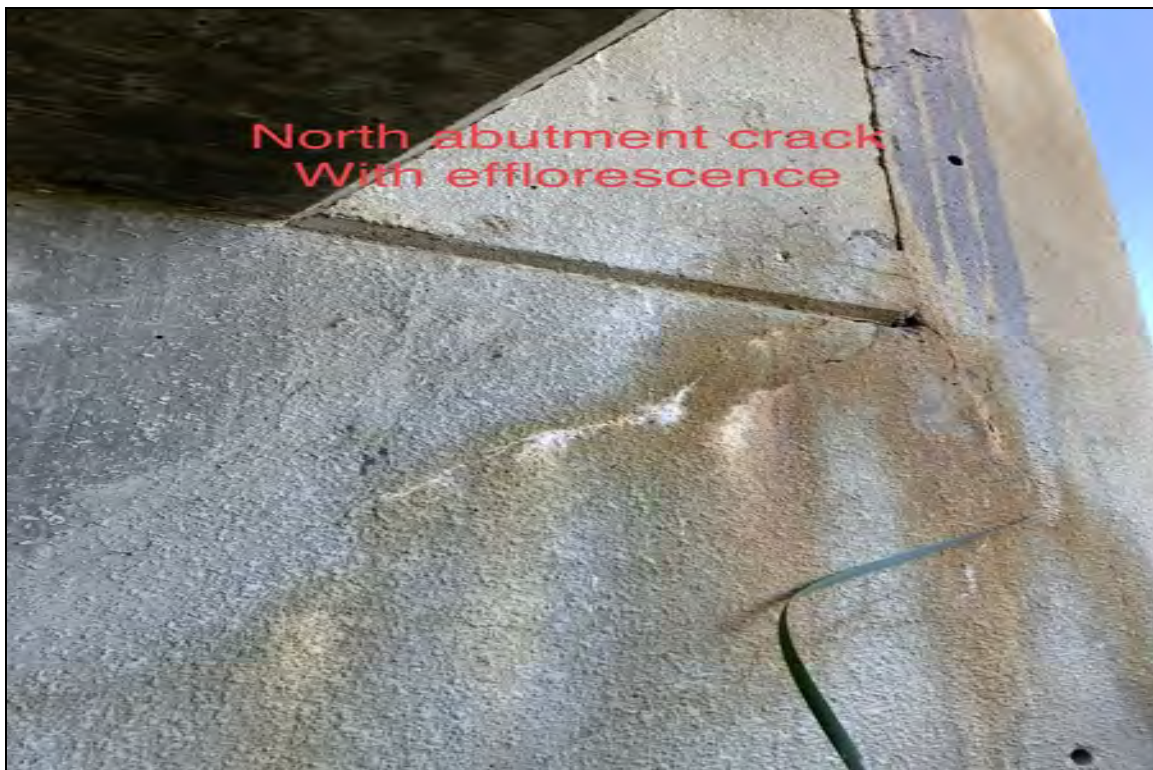
North abutment crack with efflorescence
