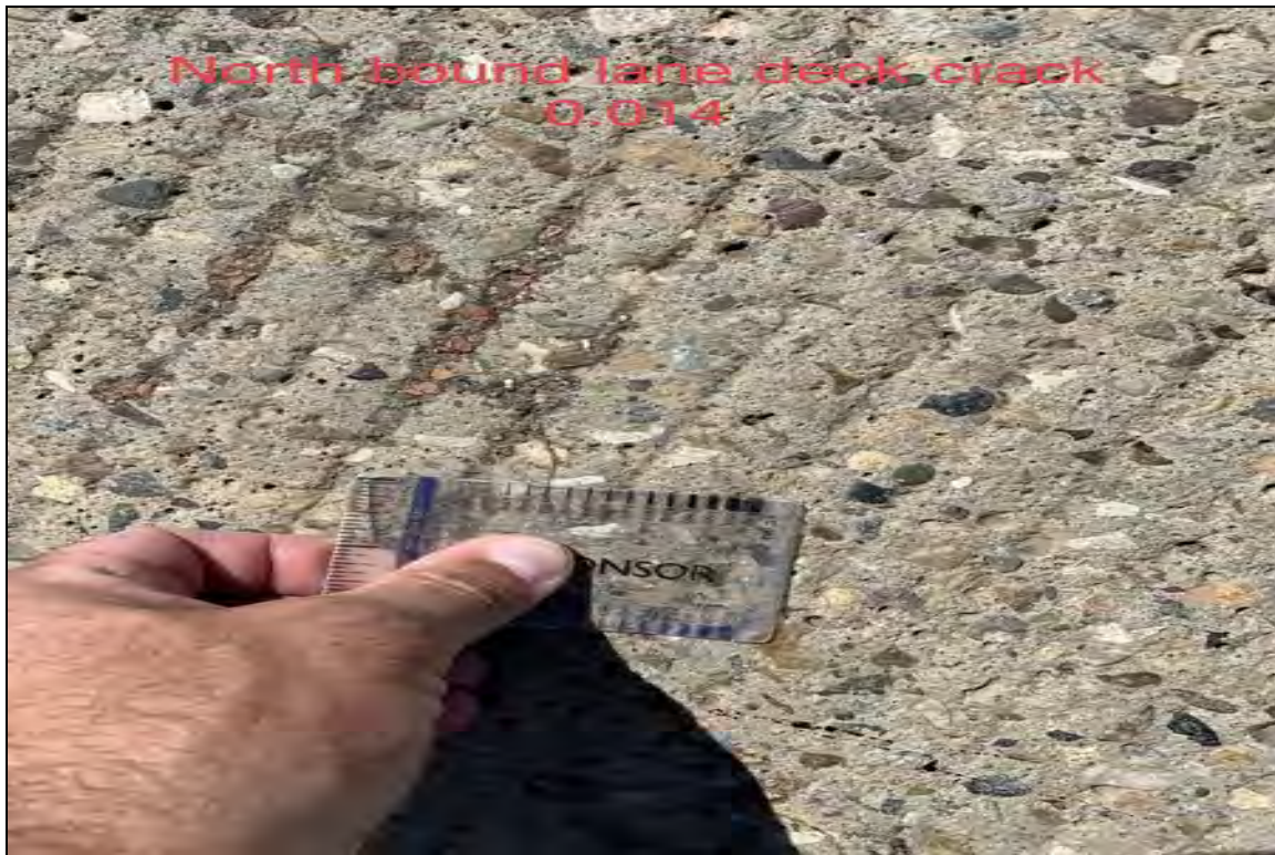
North bound lane deck crack .014
