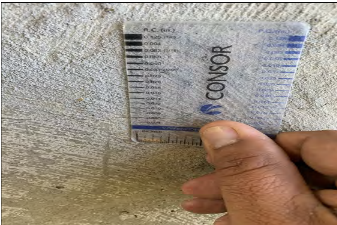
South abutment crack.006
