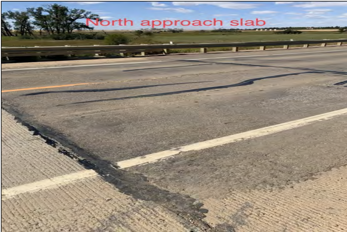
North approach slab covered with asphalt
