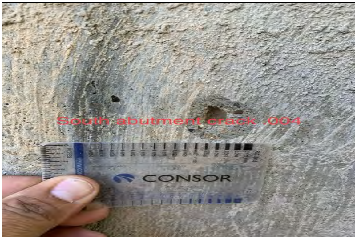
South abutment crack .004
