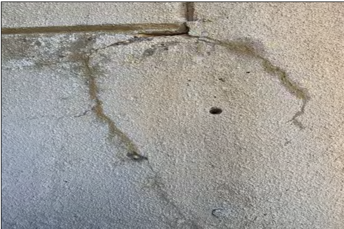
South abutment west end cracks under backwall
