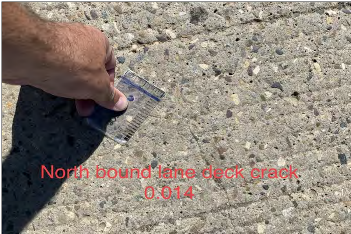
North bound deck lane crack .014
