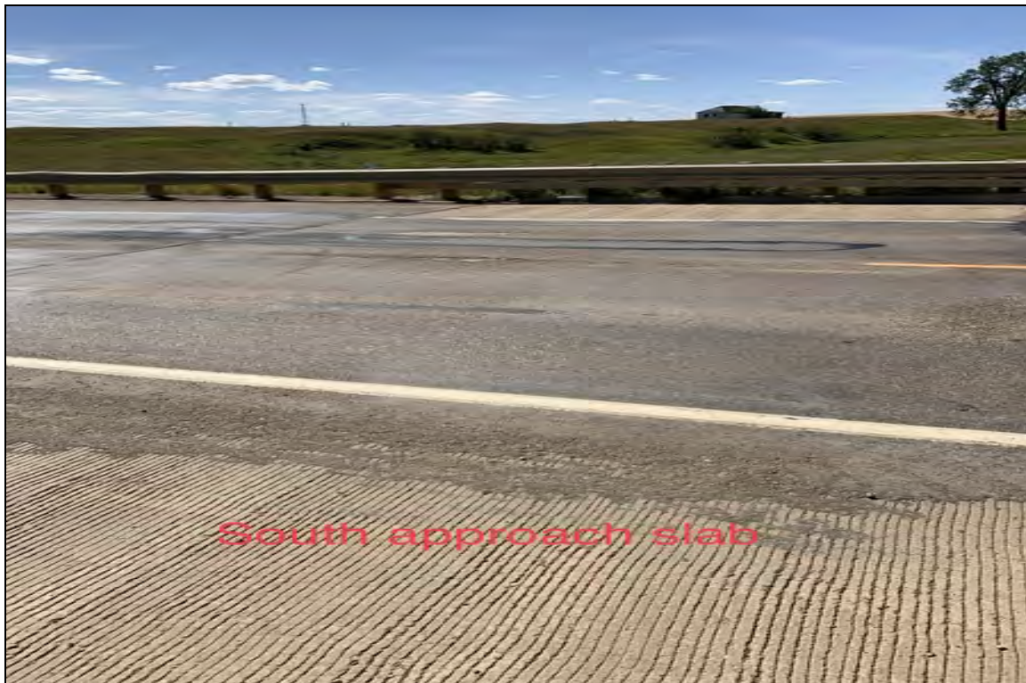
South approach slab covered with asphalt
