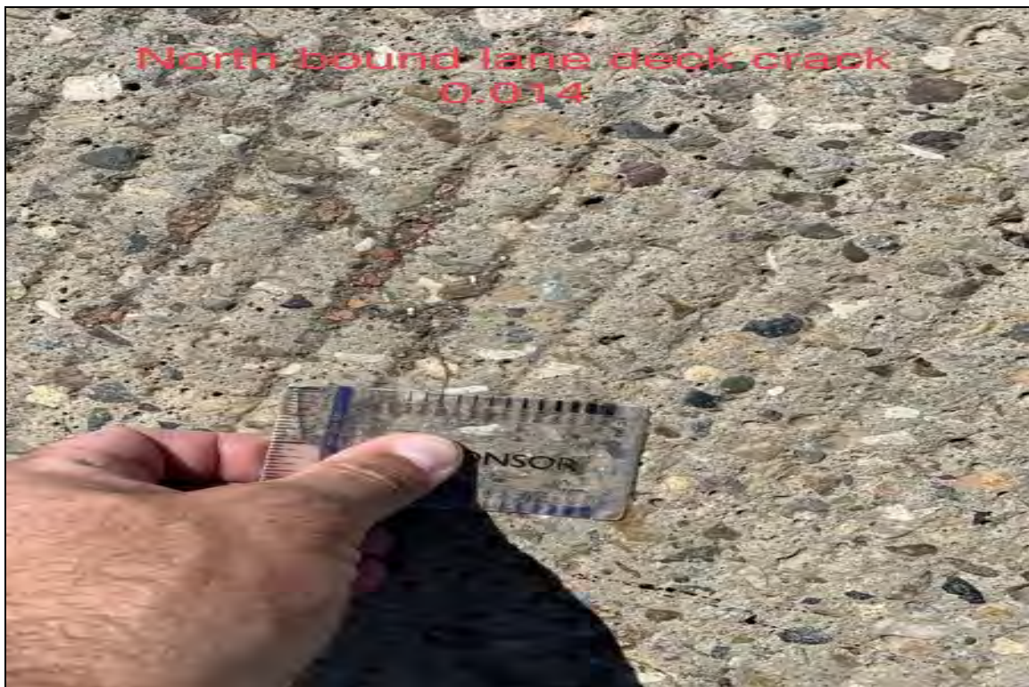
North bound lane deck crack .014
