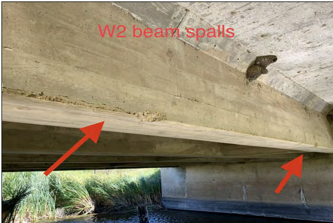
W2 beam spalls
