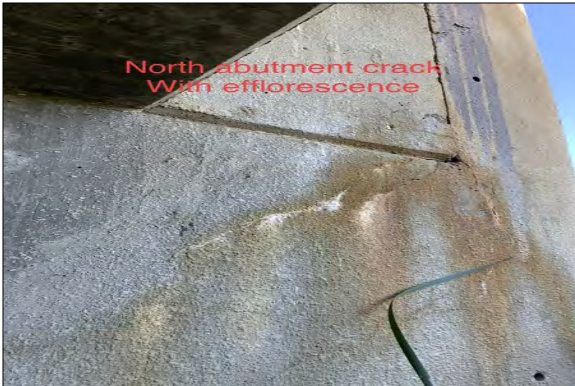
North abutment crack with efflorescence
