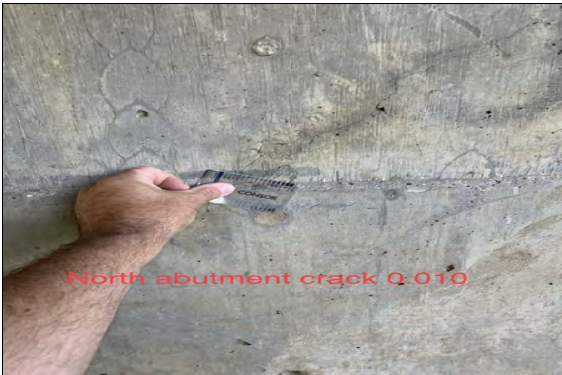
North abutment crack .010
