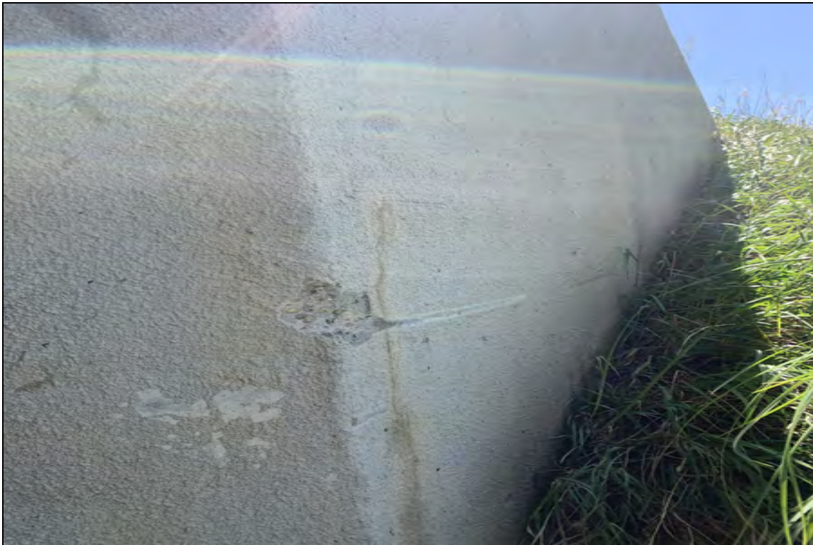
SW wing minor spall 5"x5"
