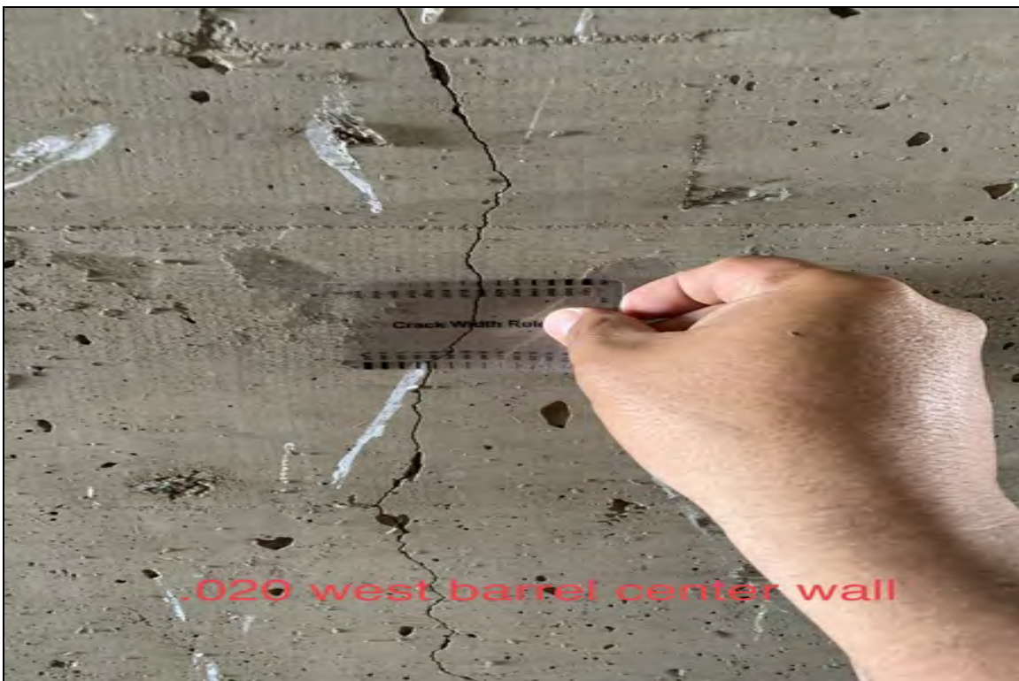
.020 west barrel center wall crack
