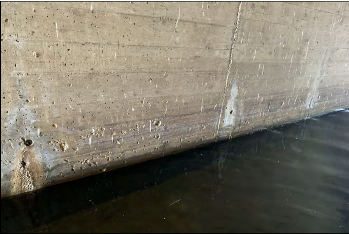
West barrel west wall cracks and efflorescence
