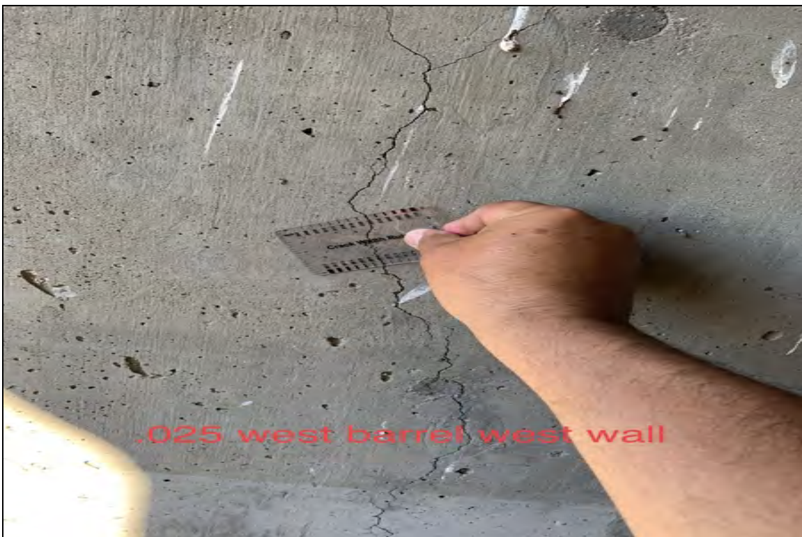
.025 west barrel west wall crack
