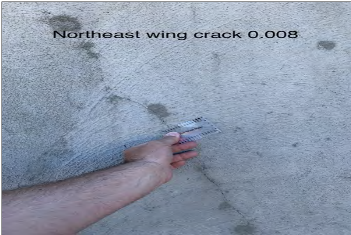
NE wing crack.008
