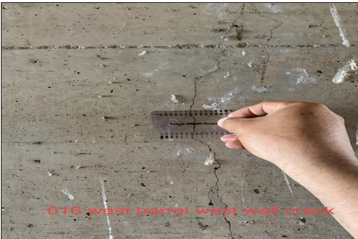
.016 west barrel west wall crack
