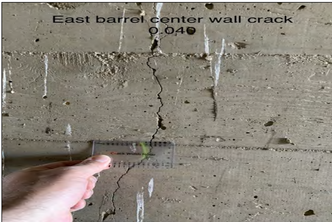
East barrel center wall crack .040
