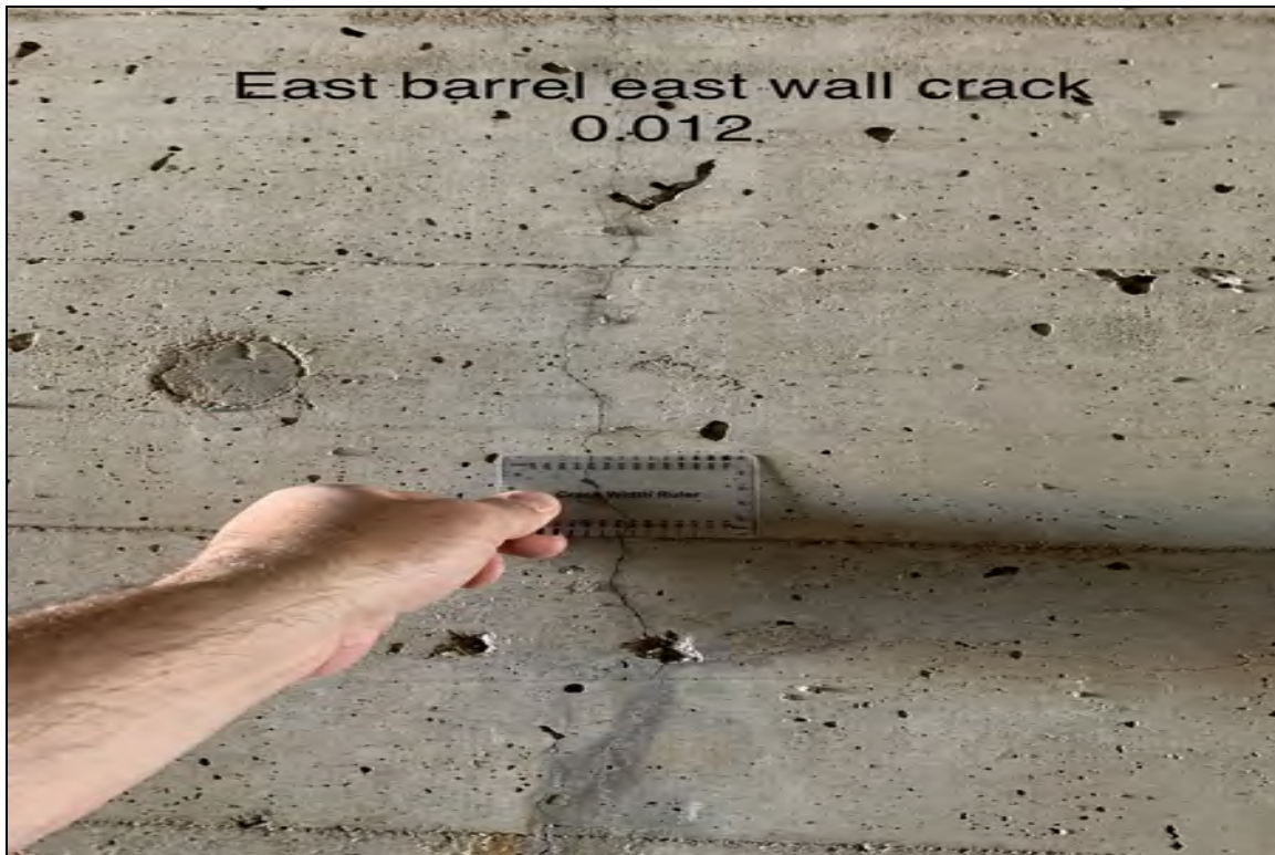
East barrel east wall crack .012
