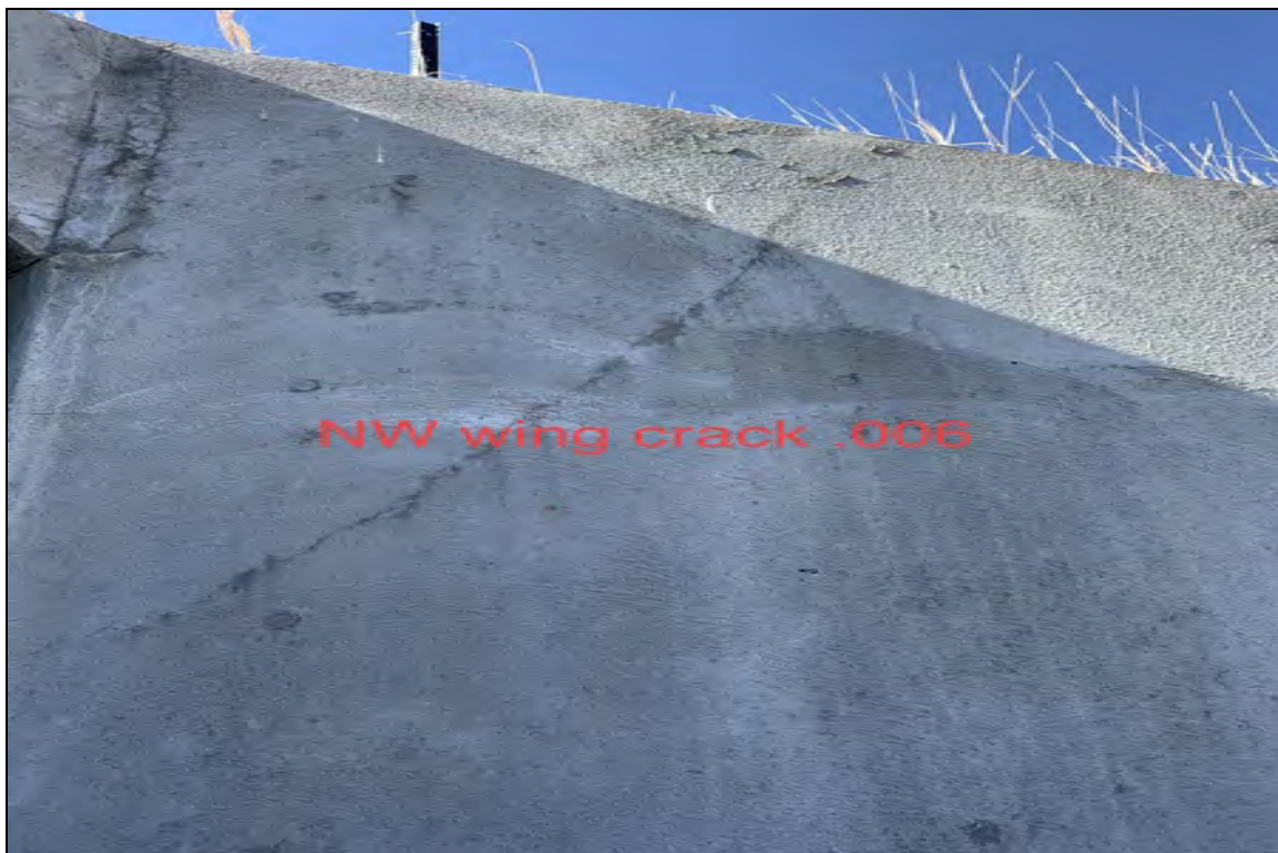
NW wing crack .006
