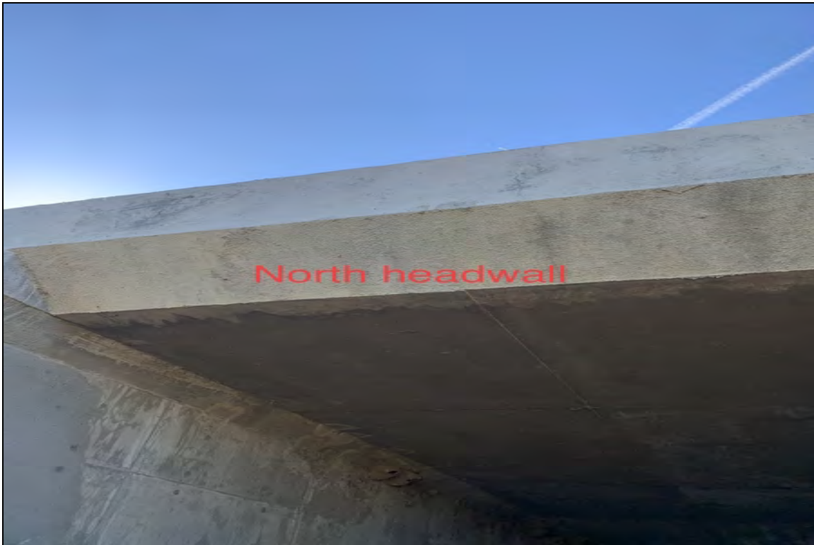
North headwall crack
