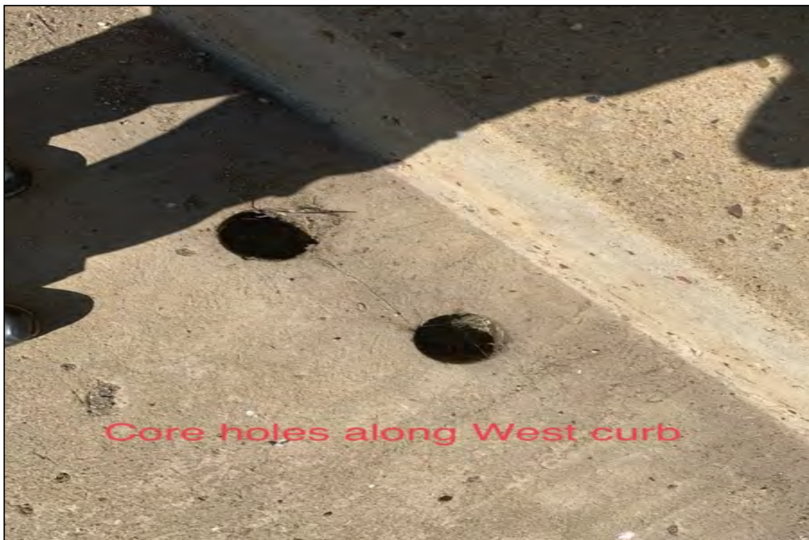
Core holes along west curb
