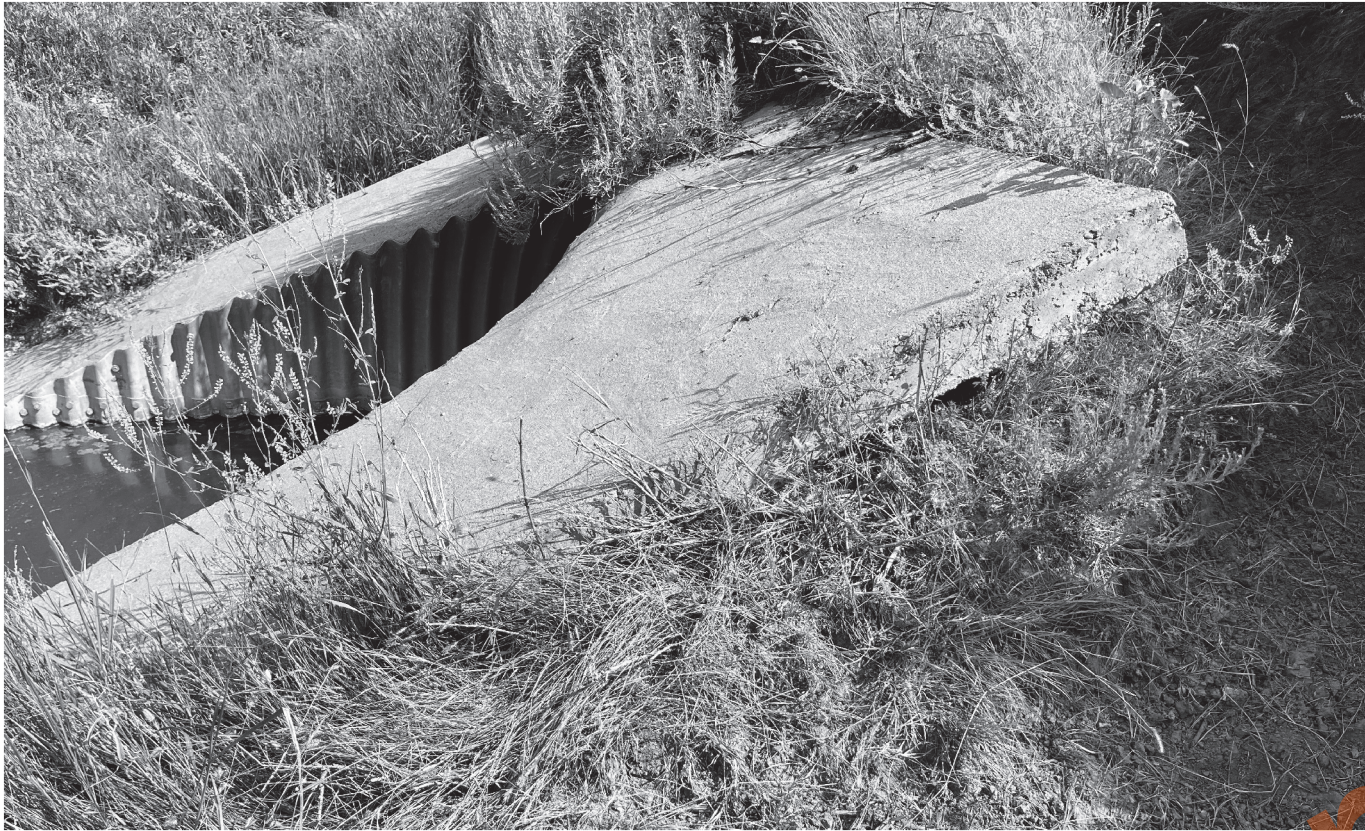
Headwall Undermining Site 2 Sta 5905+04
