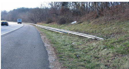
Photo A: Stacked Rails System - Foreslope is steeper than 10:1 and no steeper than 4:1. Top rail remains parallel to the road elevation (to a maximum of 46" height) so no override should occur. Once the top rail crosses the toe of the backslope (the BLON), the anchorage must be developed.
