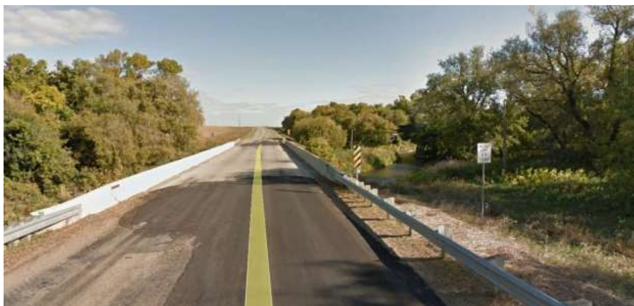
Figure 25: Existing Posted Bridge – North of Portland, ND.
