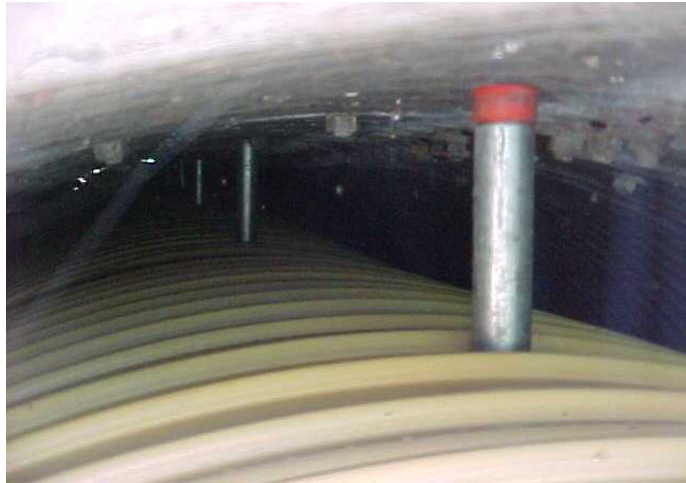
Bracing to host structure through 12 o'clock grout port
