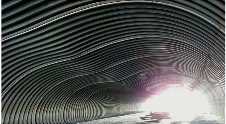
With the right pre-cautions, this type of failure can easily be avoided
