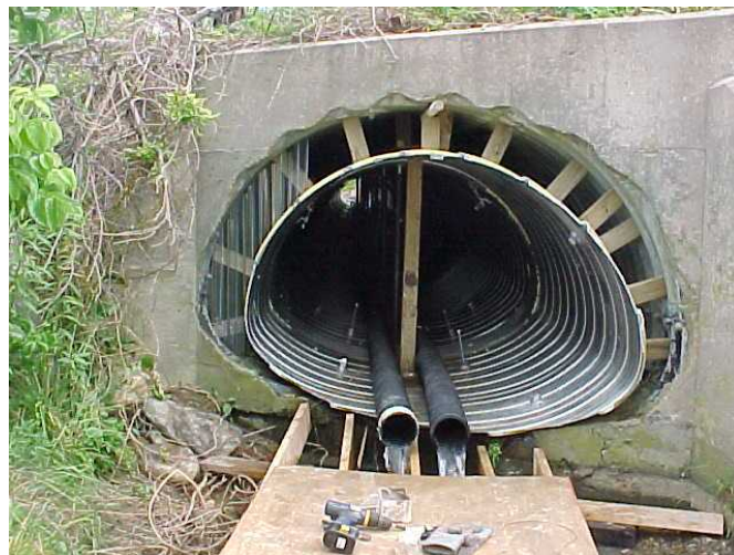
Bypass piping at outlet
