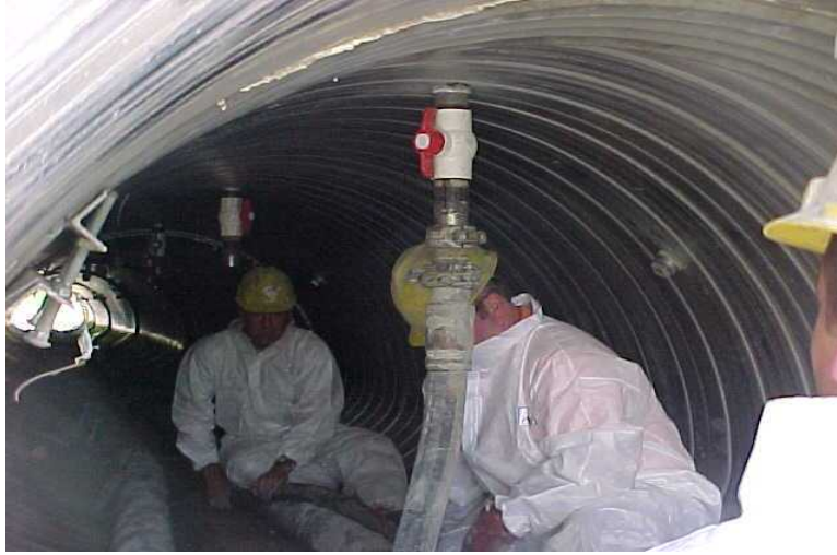
Day 8 –Last grout lift. Back grout procedure complete.
