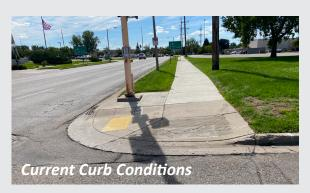
Replace sidewalk crossings with curb ramps at intersections to provide adequate accessibility and meet ADA standards.
