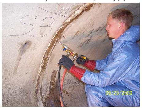
Photo 139: Subsurface injecting flexible foam
