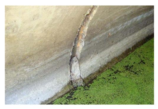
Photo 7: Condition at Joint #14, previous repair (inventory reference photo 29-004)
