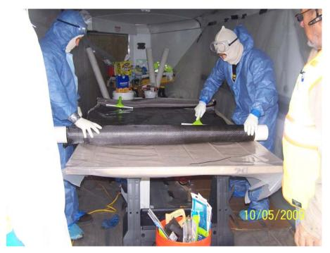
Photo 142: QuakeWrap being saturated before installation
