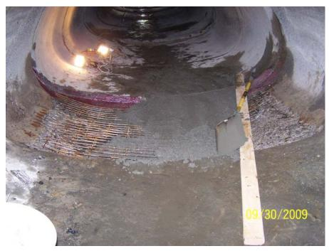
Photo 136: Cretex tied wire mesh to existing steel reinforcement and then filled deteriorated section with concrete
