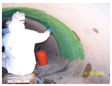
Photo 143: QuakeBond<sup>™</sup> J201TC Tack Coat being installed. Does not need to be placed on the bottom.
