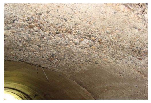
Photo 6: Deteriorated condition of concrete near Joint #10, (inventory reference photo 29-003)
