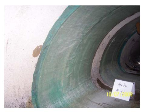
Photo 145: QuakeWrap<sup>™</sup> VB26G Glass Fabric installed
