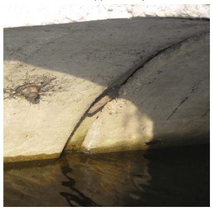
Photo 4: Condition of separated segment
