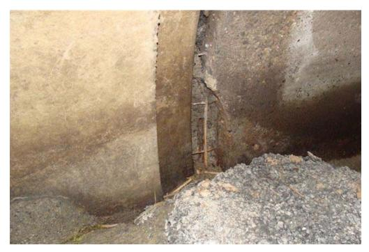
Photo 5: Condition of Joint #10, missing male section of joint, (inventory reference photo 29-002)
