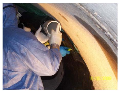
Photo 144: QuakeWrap<sup>™</sup> TB20C Carbon Fabric being installed
