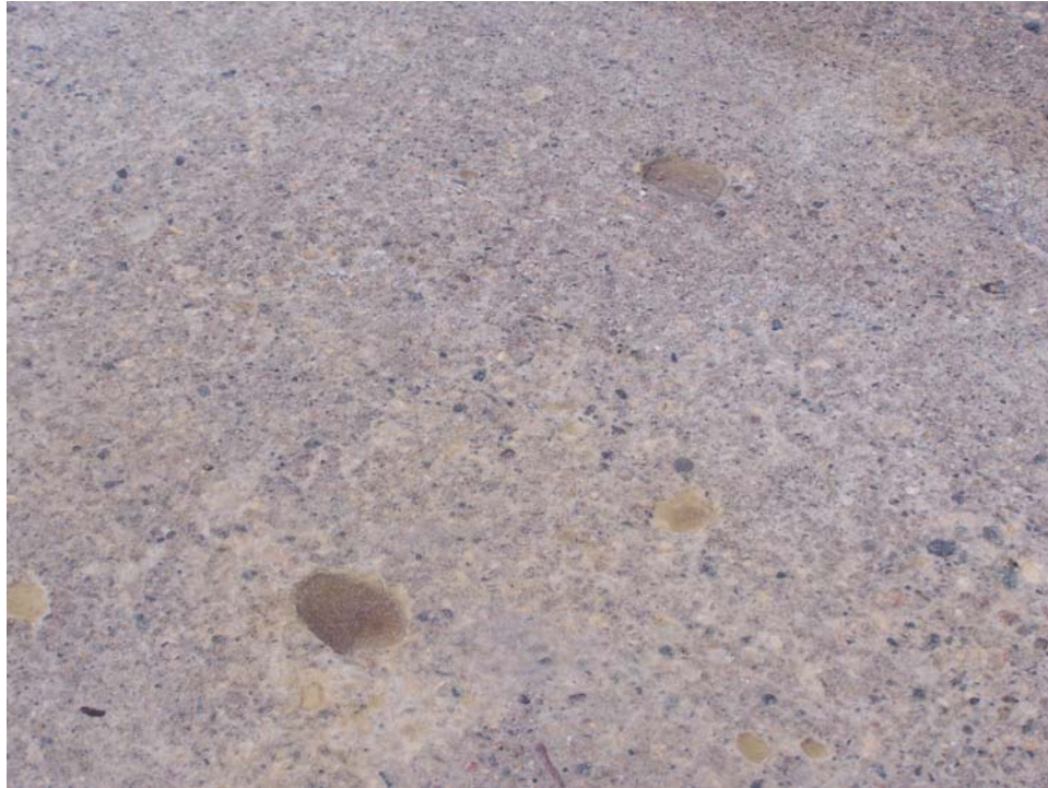
Photo 24 - Popouts filled with Degusa sealer.
