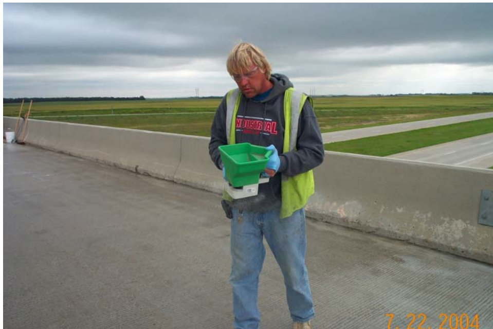
Photo 12 - Broadcasting sand to help maintain skid resistance to the Degusa Degadeck Crack Sealer section.
