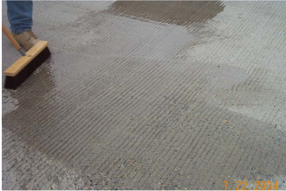
Photo 11 - Applying Degusa Degadeck Crack Sealer with a broom.
