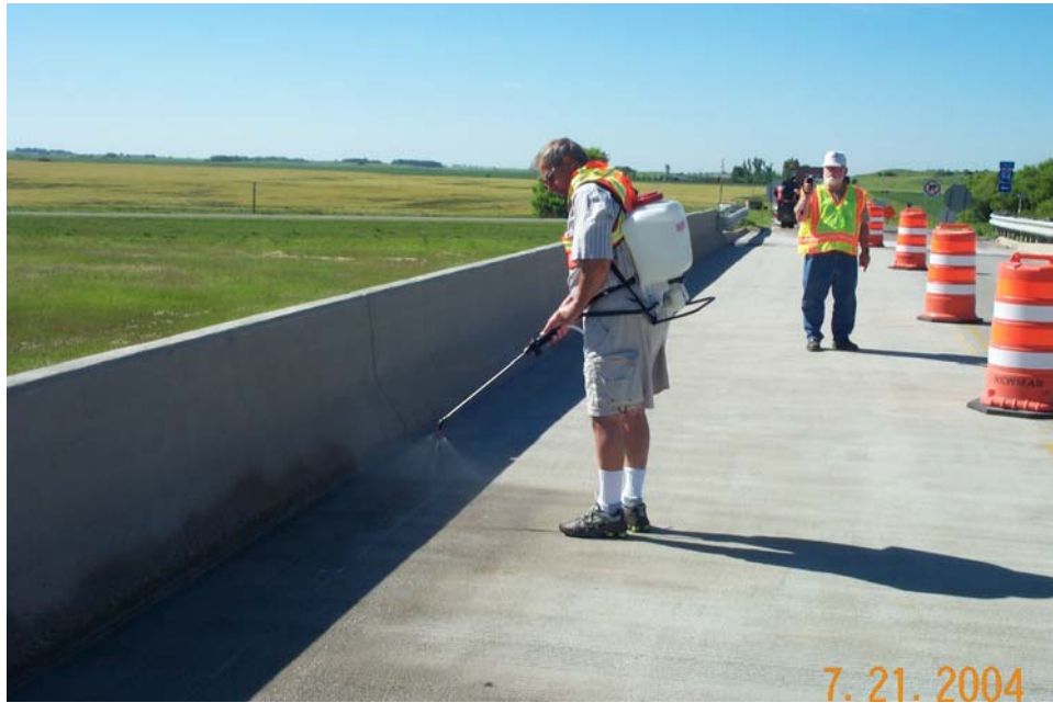
Photo 6 - Backpack sprayer and application of Radcon Formula #7.
