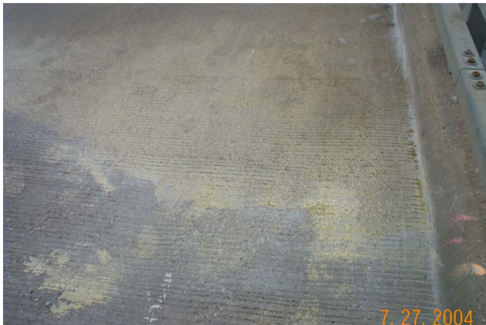
Photo 14 - Chemical reaction between the Radcon Formula #7 and Degusa Degadeck Crack Sealer. Radcon was applied first and did not allow the Degusa Degadeck Crack Sealer to penetrate the concrete for adherence.
