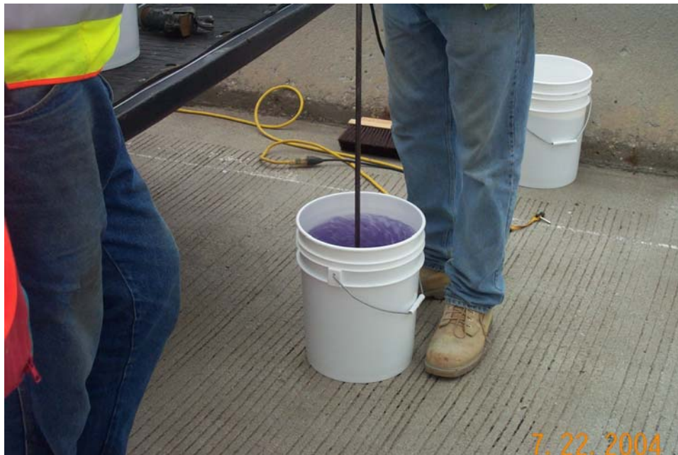
Photo 10 - Mixing the resin and hardener of the Degusa Degadeck Crack Sealer.
