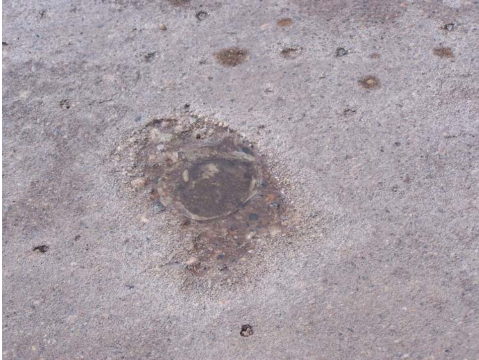
Photo 27 - Material in popout. Note the Tamms material is clearer than the Degusa product.
