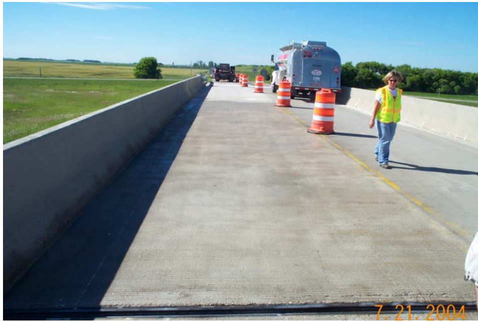
Photo 8 - Overview of Radcon Formula #7 section of the deck after application.
