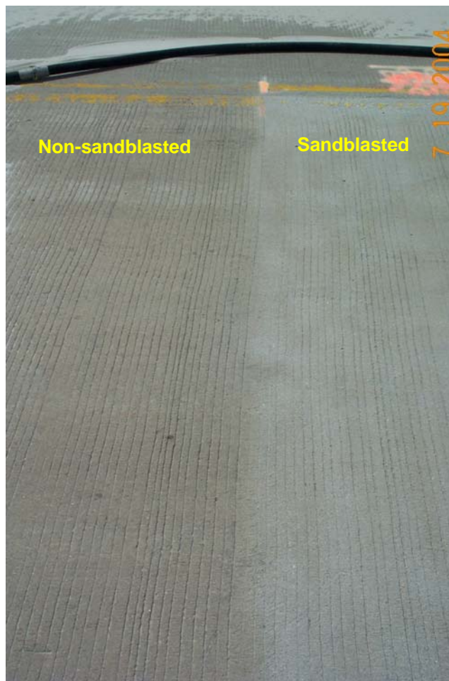
Photo 2 - Difference between sandblasted and non-sandblasted portion of the deck.
