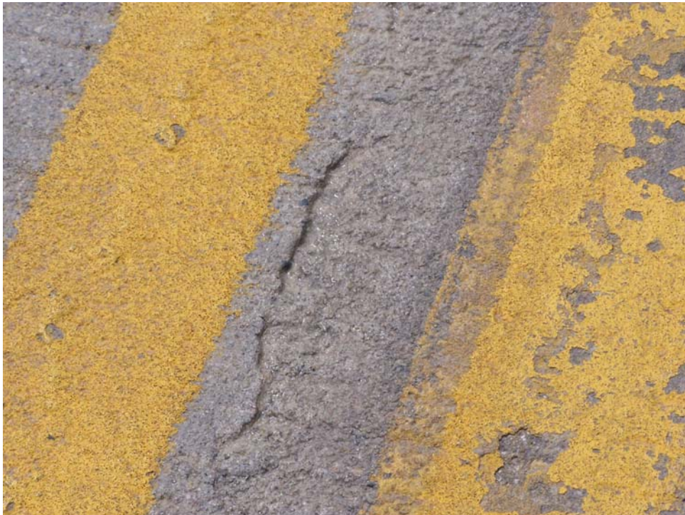
Photo 28 - Crack filled with Tamms Dural 335.
