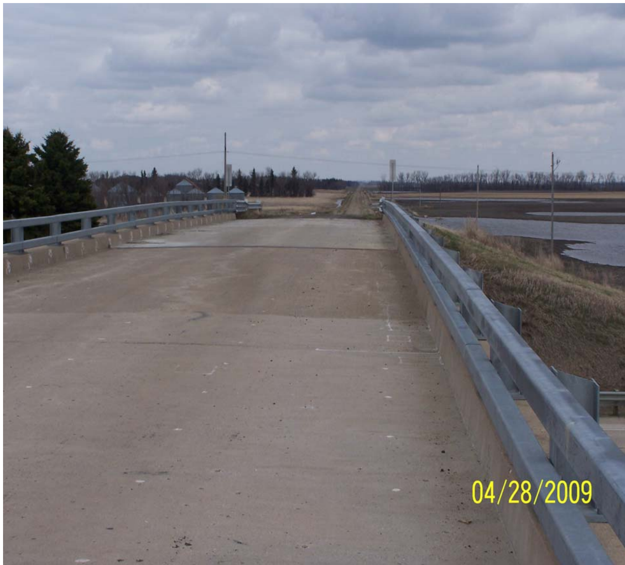
Photo 31: West Sanborn Separation Bridge
