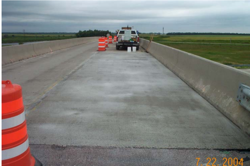
Photo 13 - Overview of a Degusa Degadeck Crack Sealer section after sand was applied.
