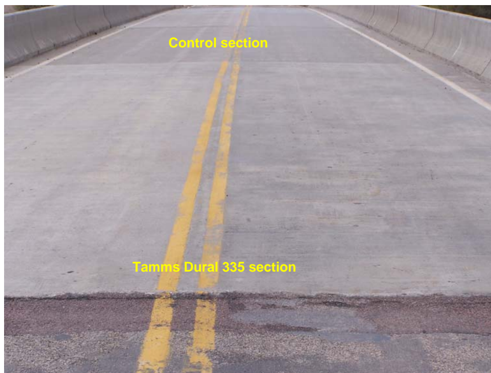
Photo 26 - Overview of a Tamms Dural 335 section.
