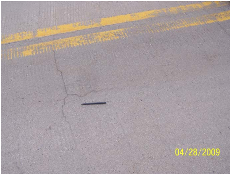
Photo 30: Eckelson Interchange moisture visible near cracks only in control section
