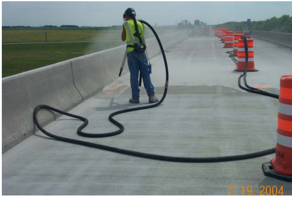
Photo 1 - Sandblasting the bridge deck.
