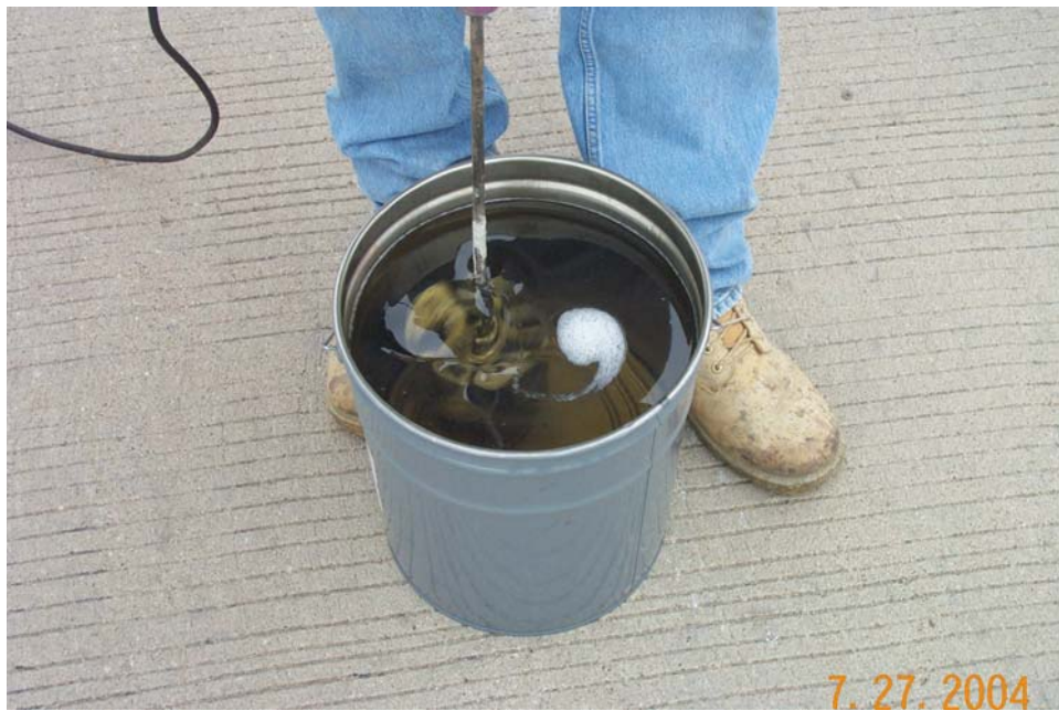
Photo 17 - Mixing the resin and hardener of the Tamms Durall 335 Sealer.
