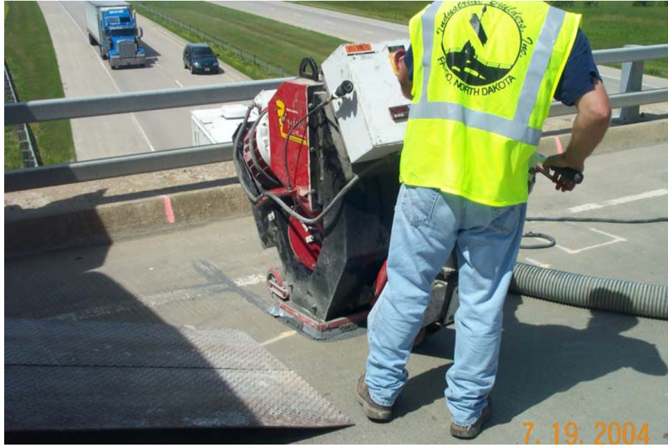
Photo 3 - Shotblasting the bridge deck.
