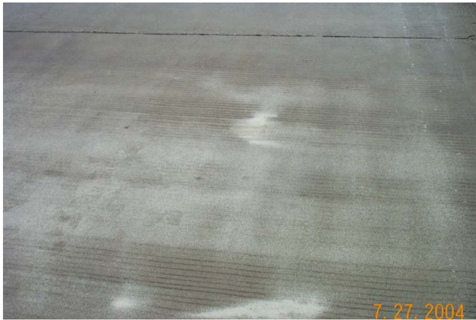
Photo 19 - Applied sand to the Tamms Dural 335 sealer.
