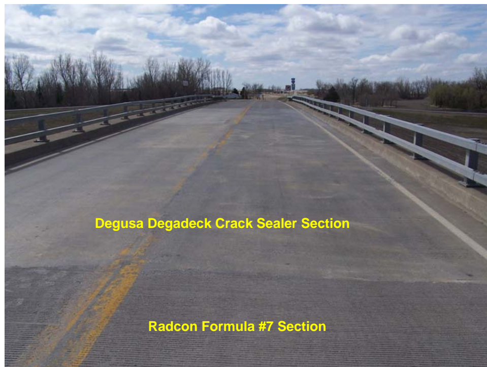
Photo 23 - Overview of a Degusa Degadeck Crack Sealer section.
