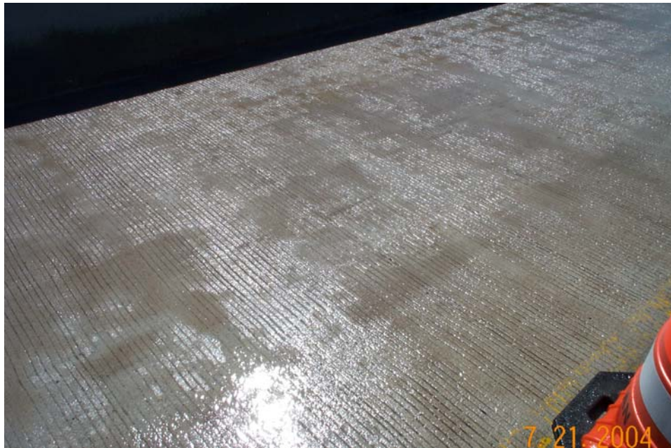
Photo 7 - Radcon Formula #7 applied to the bridge deck.
