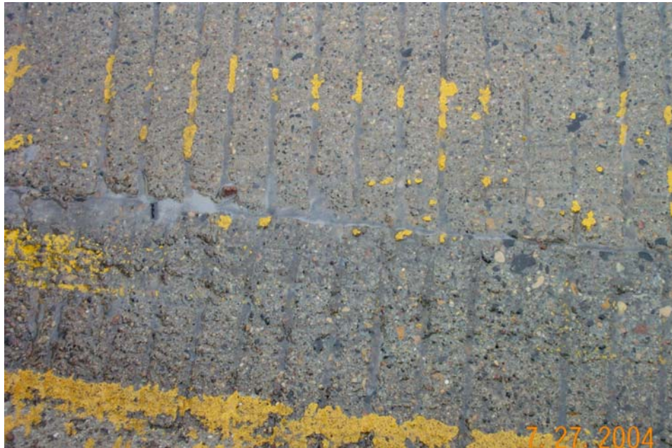
Photo 20 - Crack sealed with Tamms Dural 335.
