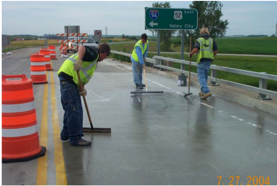
Photo 18 - Applying Tamms Dural 335 Sealer with a squeegee.
