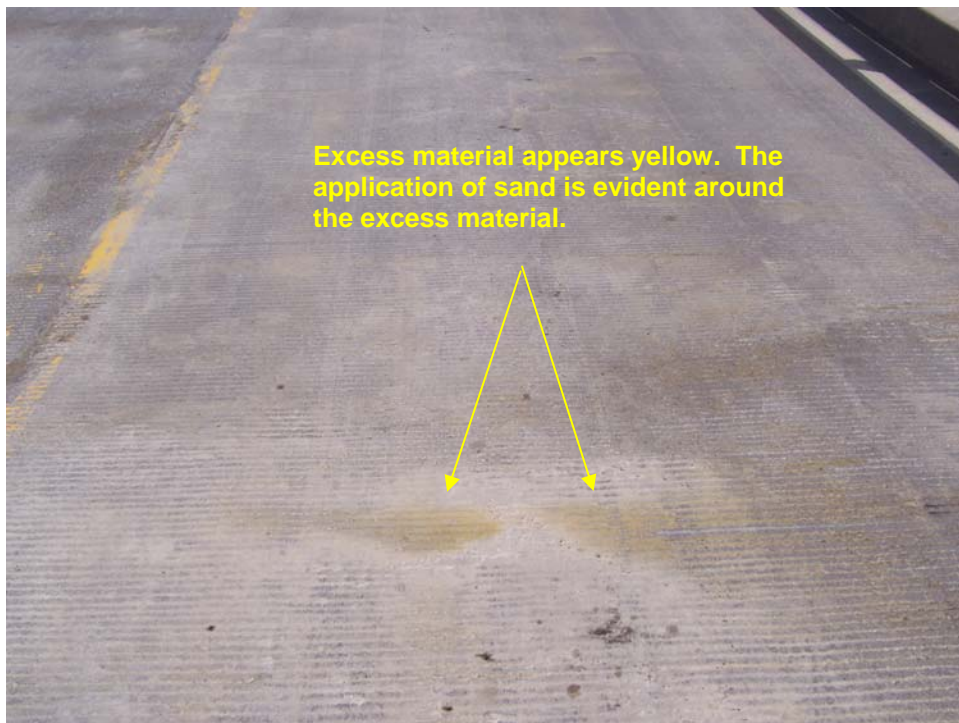
Photo 25 - Excess material applied in a Degusa section. Applied sand is visibly noticeable as well.
