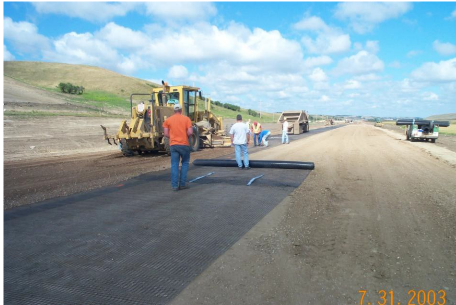
Photo 4 – Starting new roll of geogrid.
