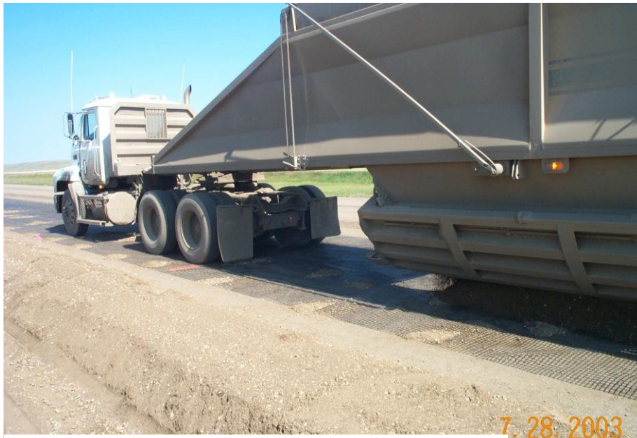
Photo 8 – Placing the base material on the geogrid.
