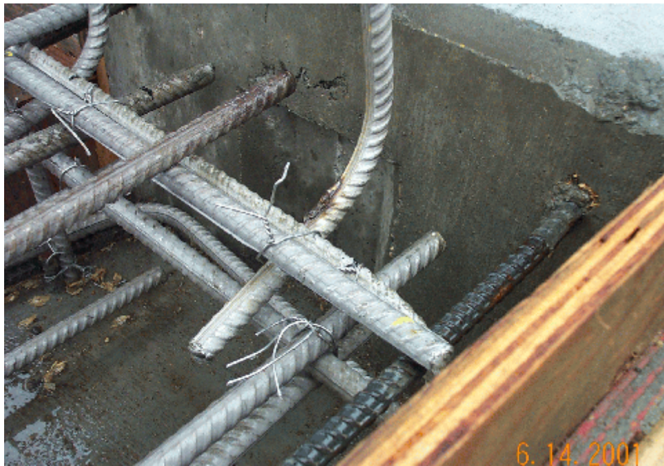
Photo 7. k-type bar cut and welded
