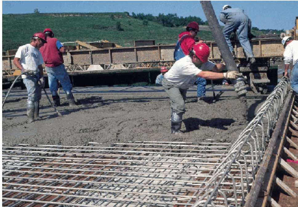
Photo 9. Bridge deck being poured
