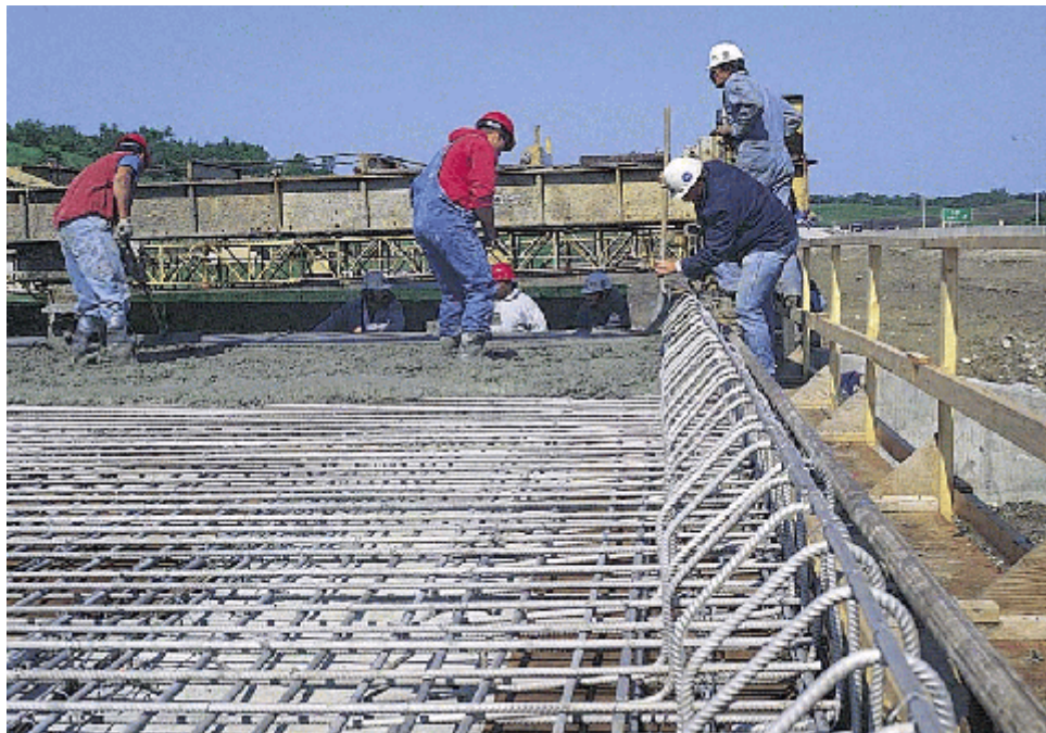
Photo 10. Bridge deck being poured
