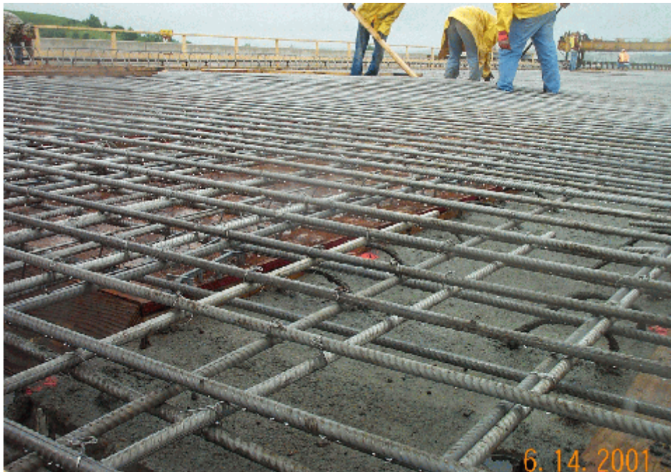
Photo 6. Placement of Stainless Steel Clad Rebar
