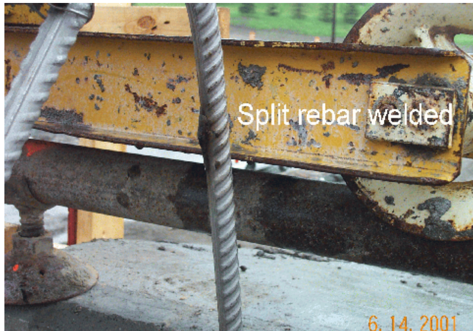
Photo 8. Split rebar welded
