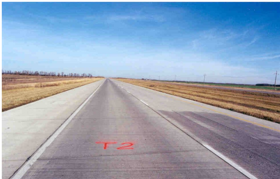
Photo 8 - Overall view of Test Section 2
