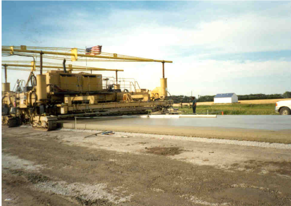
Photo 3 - Finished PCC pavement prior to carpet drag
