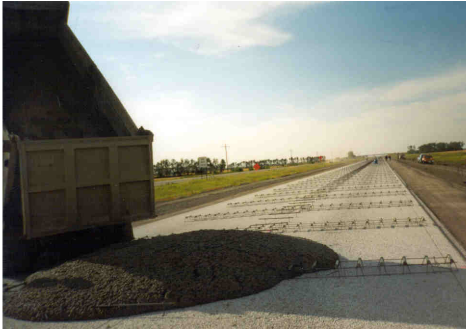
Photo 2 - Placing of the concrete
