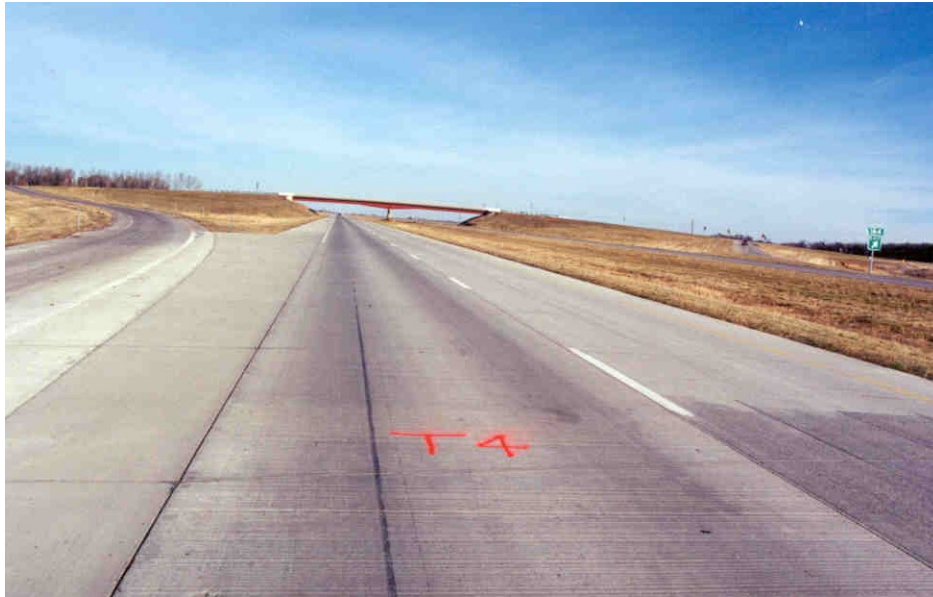
Photo 12 - Overall view of Test Section 4
