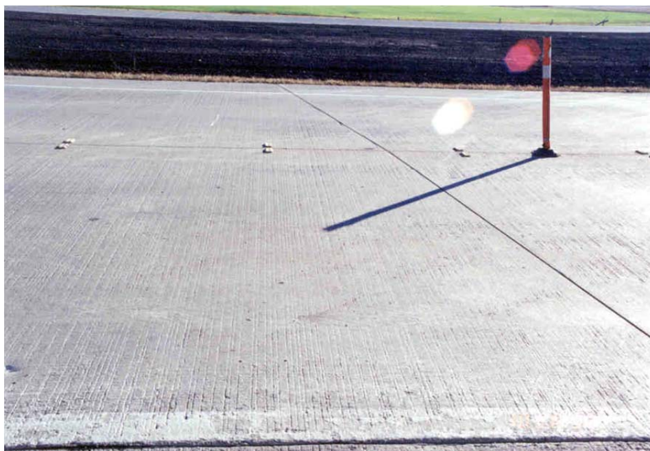
Photo 9 - Tining in Test Section 2 at Station 8930+00
