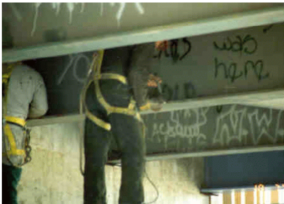
Photo 7: View of worker spot grinding.
