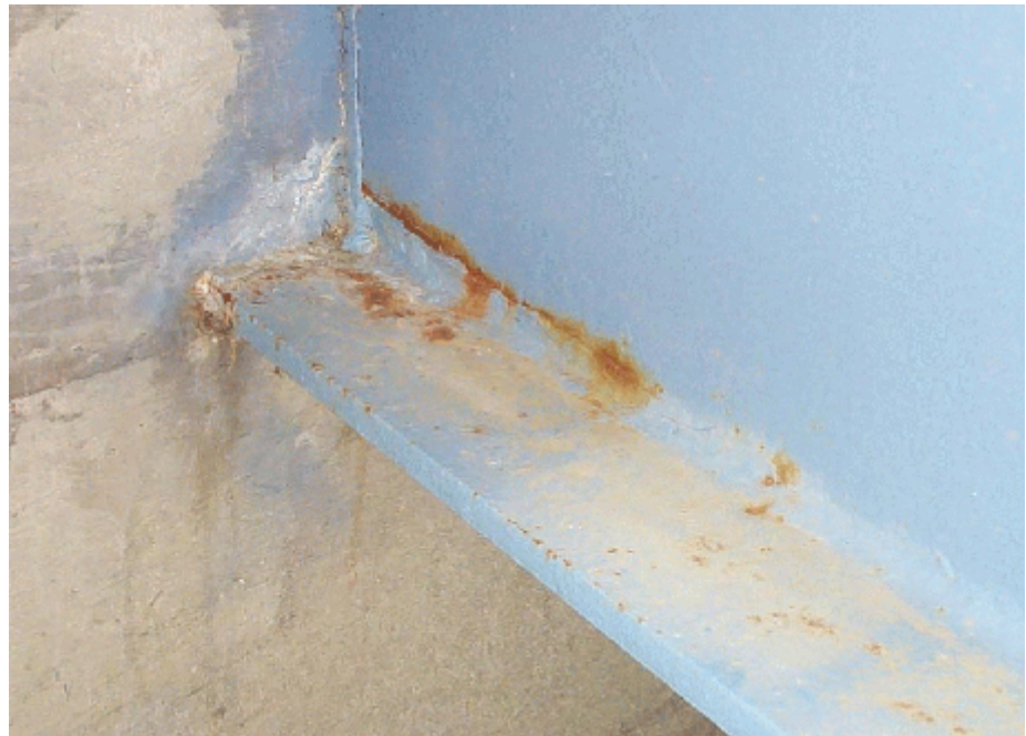
Photo 17: Damaged south beam on westbound structure.
