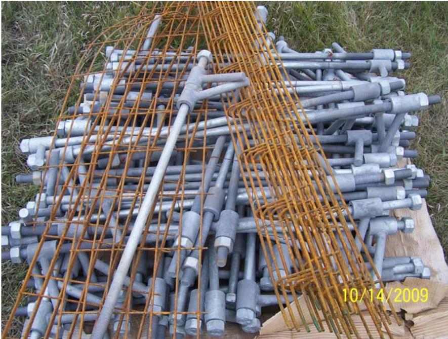
**Photo 141: Internal Joint Ties**
