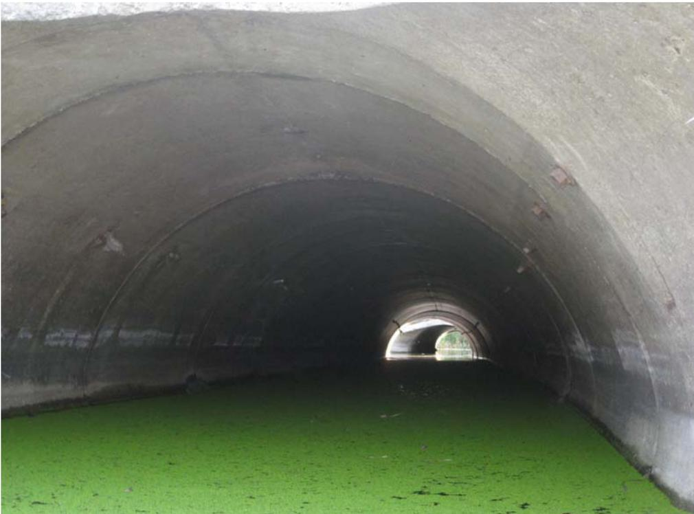
**Photo 2: Conditions inside pipe, note standing water and algae**
