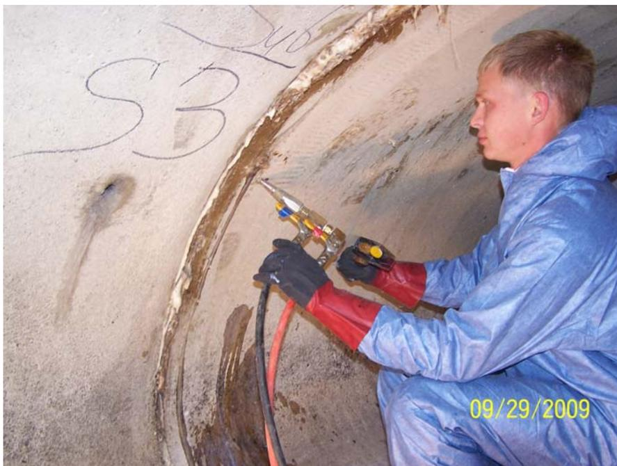
**Photo 139: Subsurface injecting flexible foam**
