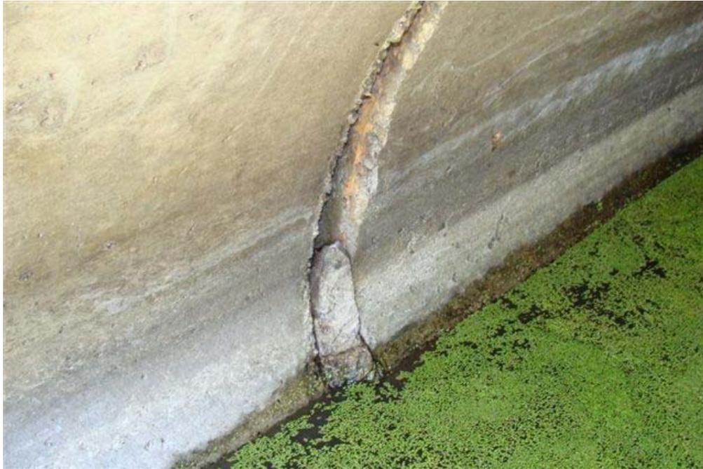
**Photo 7: Condition at Joint #14, previous repair (inventory reference photo 29-004)**
