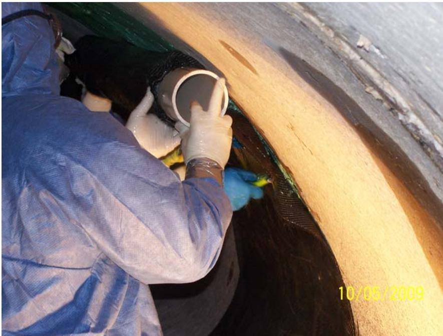
**Photo 144: QuakeWrap™ TB20C Carbon Fabric being installed**
