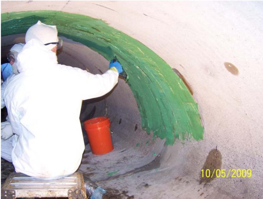
**Photo 143: QuakeBond™ J201TC Tack Coat being installed. Does not need to be placed on the bottom.**
