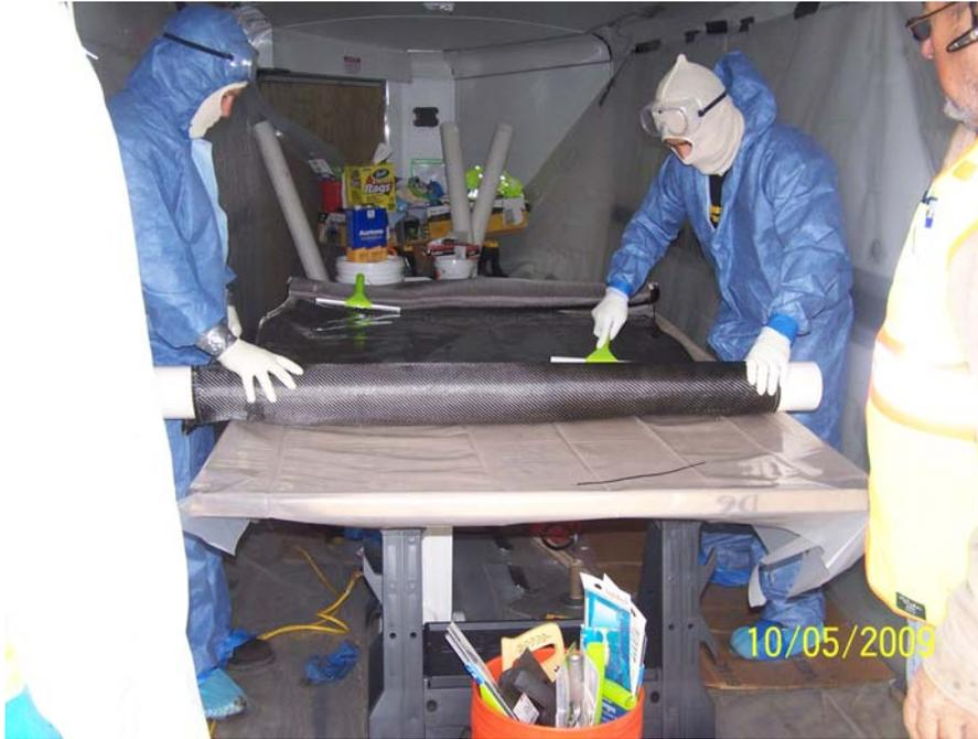
**Photo 142: QuakeWrap being saturated before installation**
