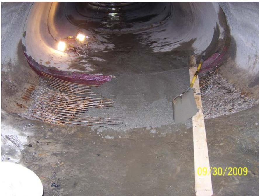
**Photo 136: Cretex tied wire mesh to existing steel reinforcement and then filled deteriorated section with concrete**
