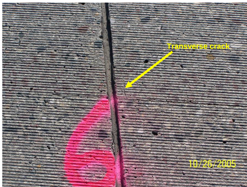
Photo 9 - Transverse crack location is likely the early signs of a coreboard failure.
