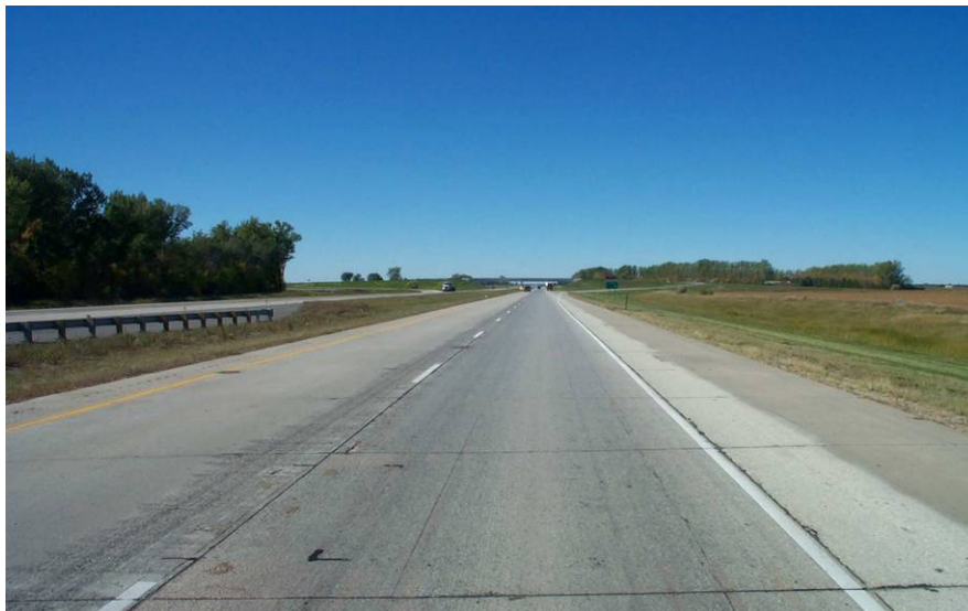
Photo 5 - Overall view of control section 2.
