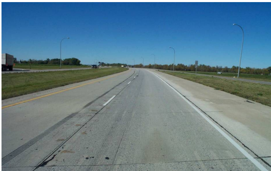
Photo 1 - Overall view of control section 1.
