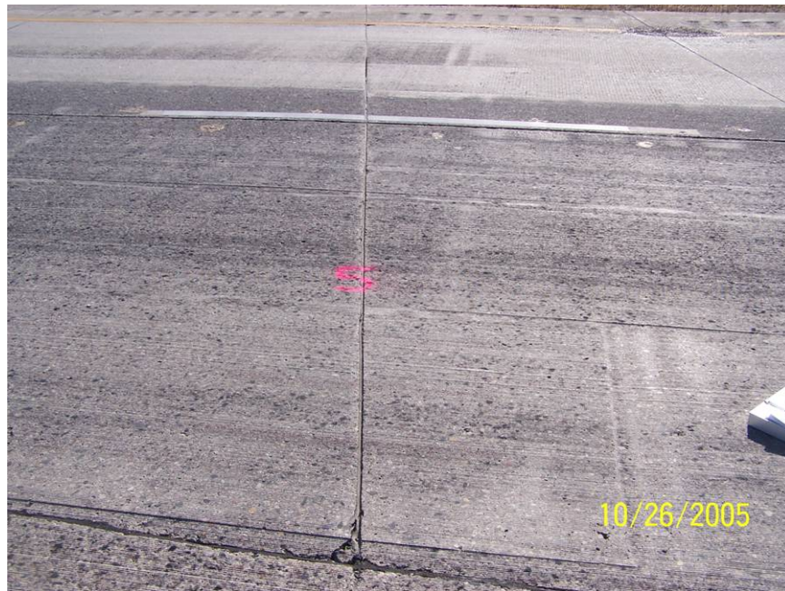
Photo 8 - Typical joint in experimental section.
