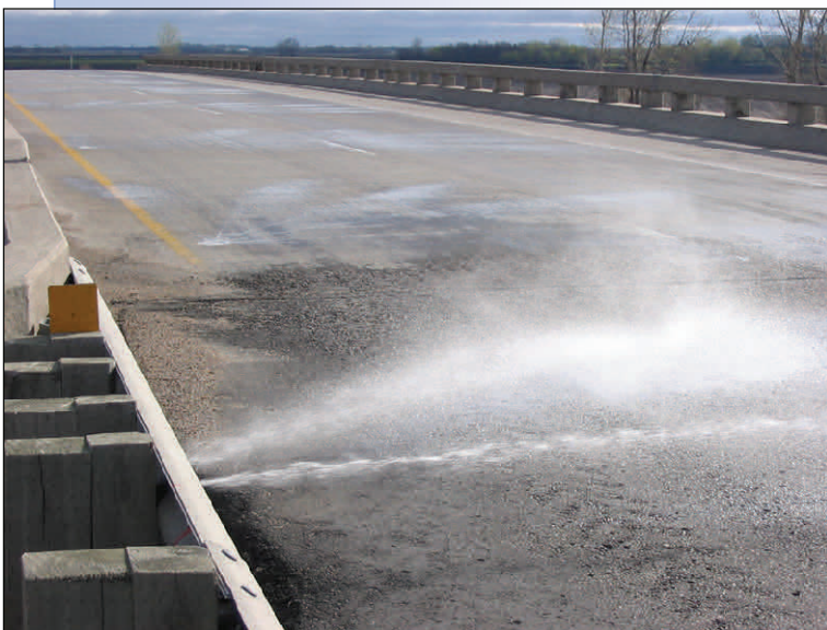
Spray nozzle in guardrail on Interstate 29 Buxton Bridge south of Grand Forks, ND
