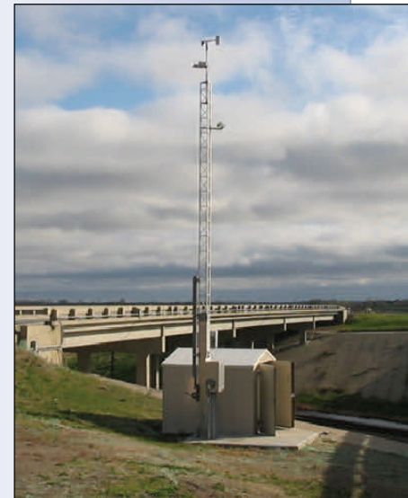
Pump house and ESS on Interstate 29 Buxton Bridge south of Grand Forks, ND
