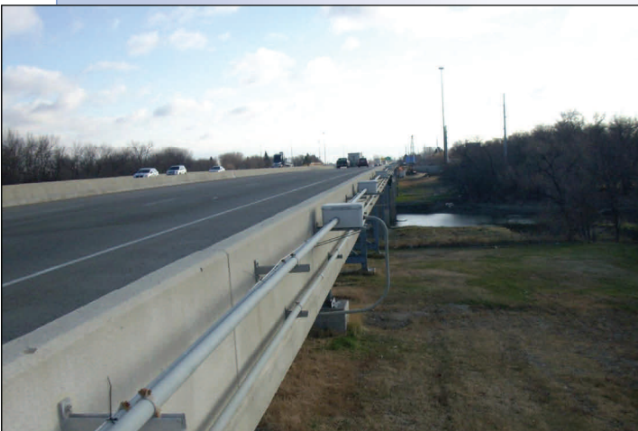
FAST plumbing system on Interstate 94 Red River Bridge between Fargo, ND and Moorhead, MN
