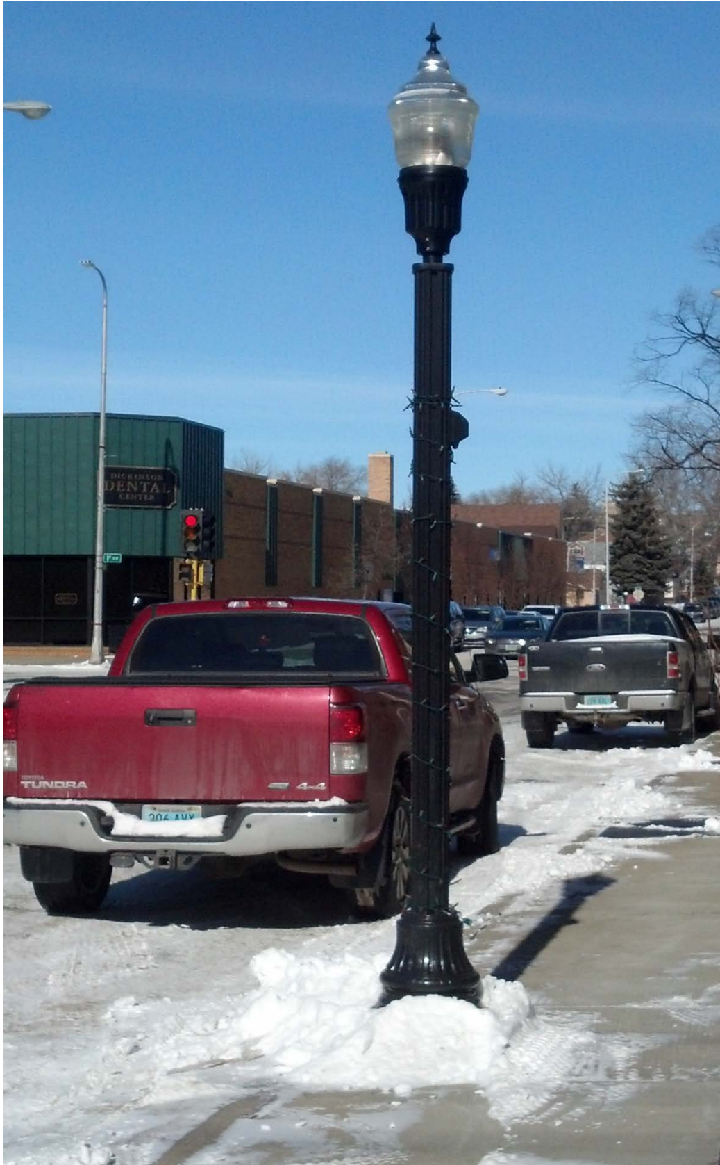
Figure 11: New Holophane post-top mounted decorative light installed in 2017. These poles by themselves won't be expected to provide adequate roadway lighting. However, they offer the most intimate lighting for pedestrians. Supplemented with taller lights for adequate roadway lighting, you can already begin to feel the difference this project will create compared to the much taller galvanized poles by the dental office in the background.
