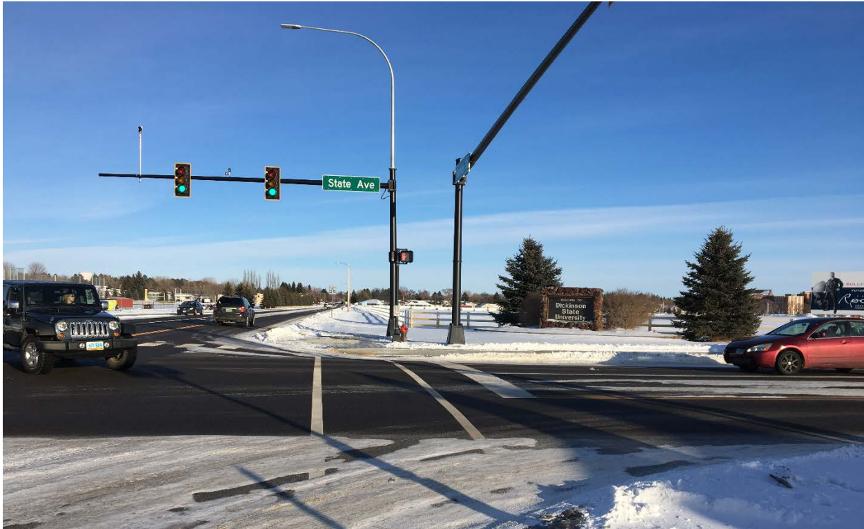
Figure 7: New Matte Black Traffic Signals by Dickinson State University 2017. We will install signal standards and mast arms similar to these at ND Hwy 22/Villard St. and Sims St./Villard intersection. If roadway lighting is necessary to be mounted on top of the signals, we will use matte black arms instead of the galvanized arms we had used on these signals
