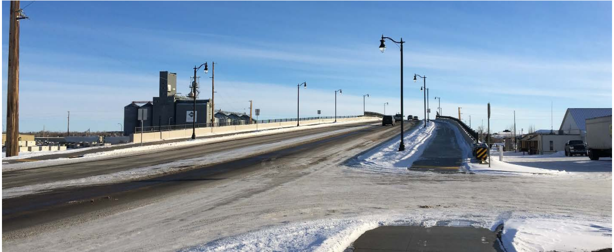
Figure 8: Taller style Holophane decorative lighting on State Ave RR Bridge installed in 2016. This was an NDDOT led project that created a second grade separated RR crossing in Dickinson. Working with the design team, the City selected these Holophane brand lights as our decorative standard at that time because of the company's longevity and reputation
