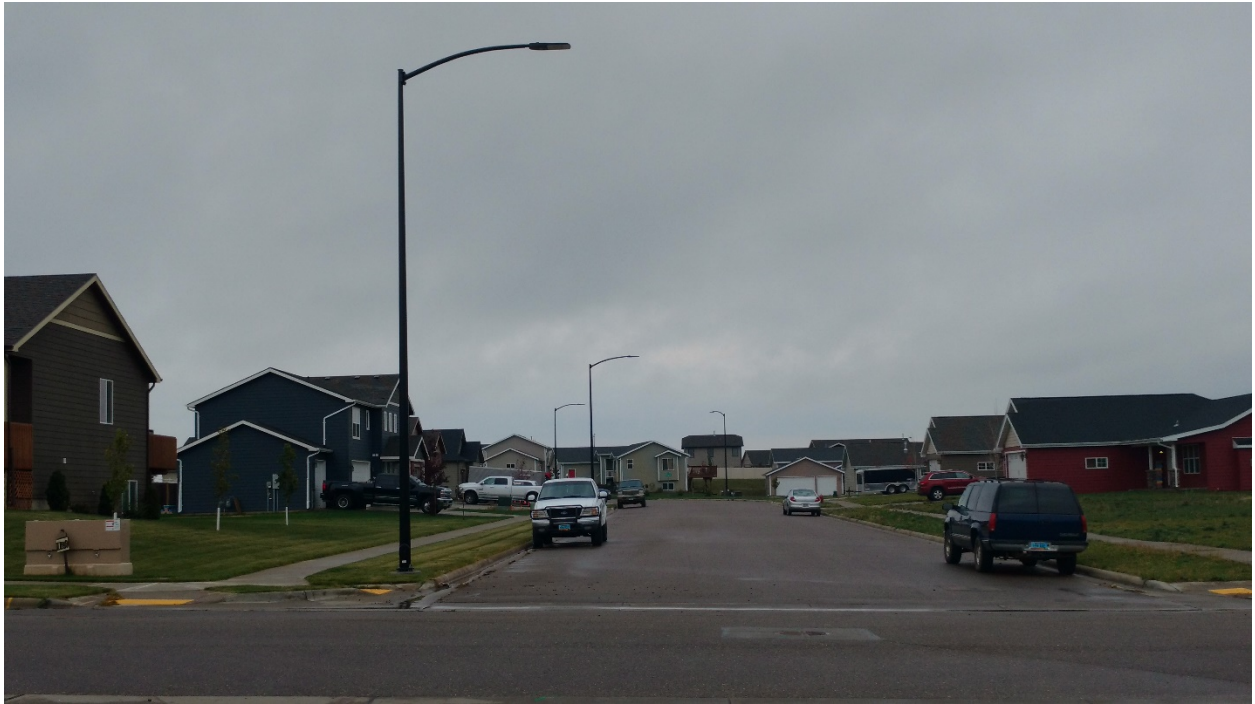
Figure 6: New City Standard Metal Light Poles in Residential Neighborhood installed in 2016. These are 30' metal poles with 8' mast arms and LED luminaires. The poles and arms are galvanized and powder coat painted in matte black. The city began installing these poles as our city standard on residential street and on collector/arterial roadways back in 2013. So far we have seen excellent corrosion and fade resistance. Depending on final lighting design we anticipate using this pole design, or something slightly taller for the west and east ends of the project. Lighting styles would transition from this style of pole to the decorative style around the renaissance zone boundary
