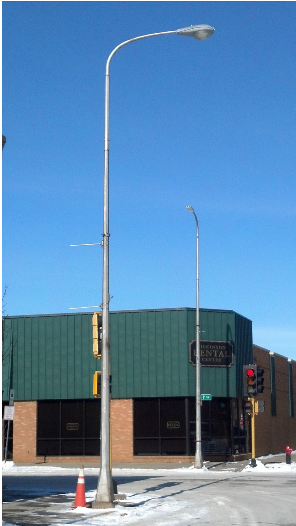
Figure 3: Existing condition at Sims St and 1st St with mixture of LED and HPS lights and outdated signals
