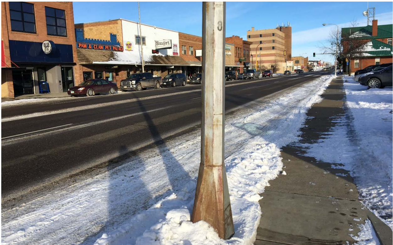
Figures 4&5: Outdated light standards on Villard St. These poles are seriously corroded, especially near the bottoms where snow, salt and brine have the most contact with the metal.
