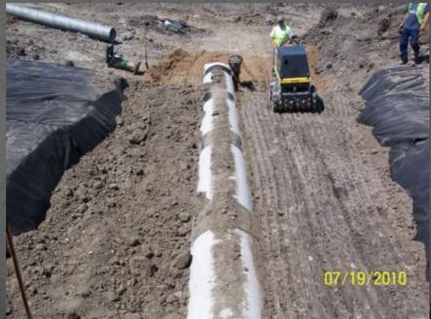
Compaction of Native Material
