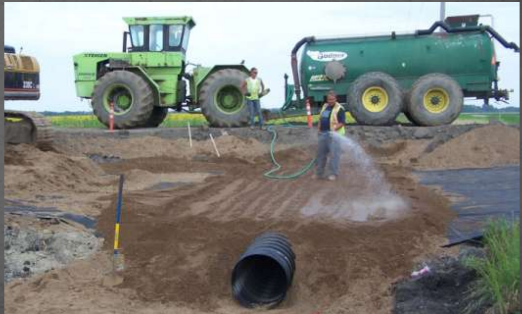
Adding Water to Aggregate
