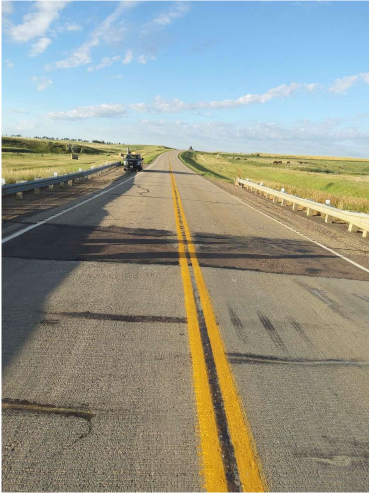
3 84+1872 South end of bridge
