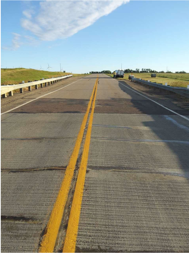
5 84+1948 North end of bridge
