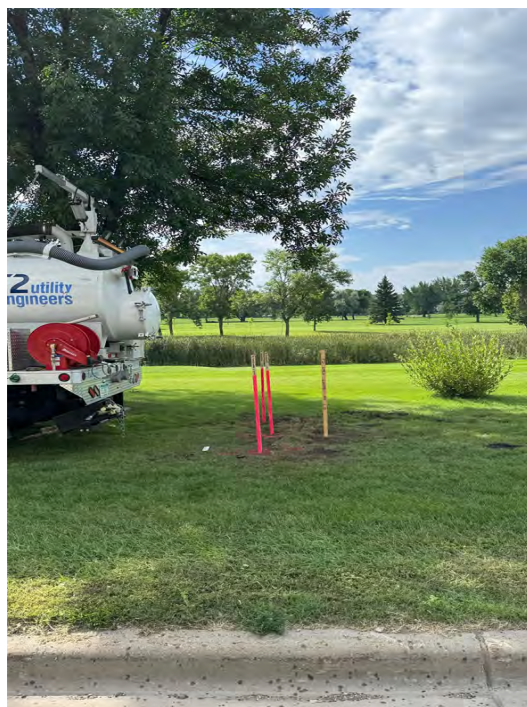
Photo No. 4 Site Photo - After Photo - South
