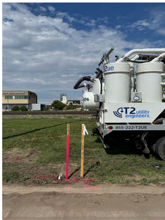
Photo No. 4 Site Photo - After Photo - North
