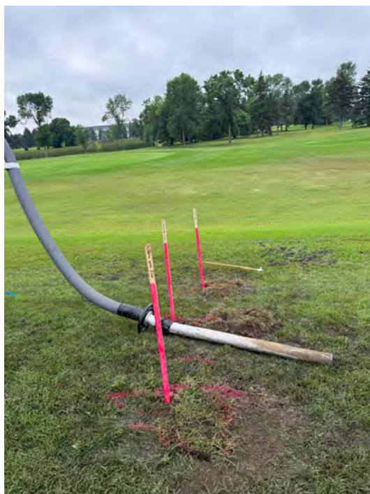
Photo No. 3 Site Photo - After Photo - South
