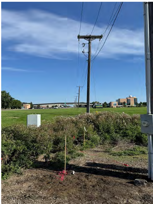
Photo No. 3 Site Photo - After Photo - North
