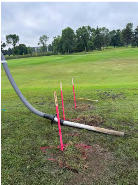
Photo No. 3 Site Photo - After Photo - South
