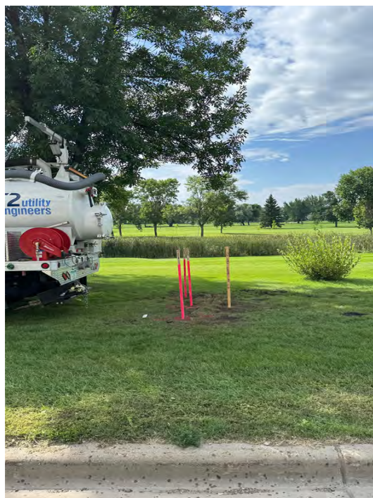
Photo No. 4 Site Photo - After Photo - South
