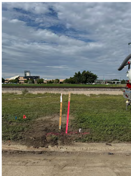
Photo No. 4 Site Photo - After Photo - North
