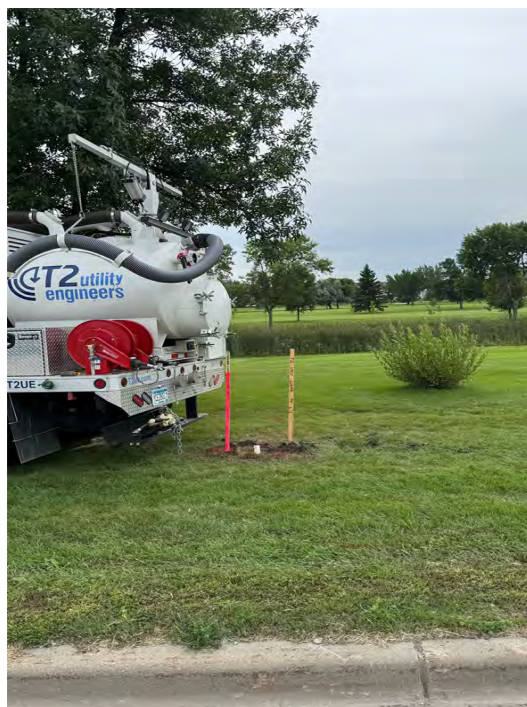
Photo No. 4 Site Photo - After Photo - South
