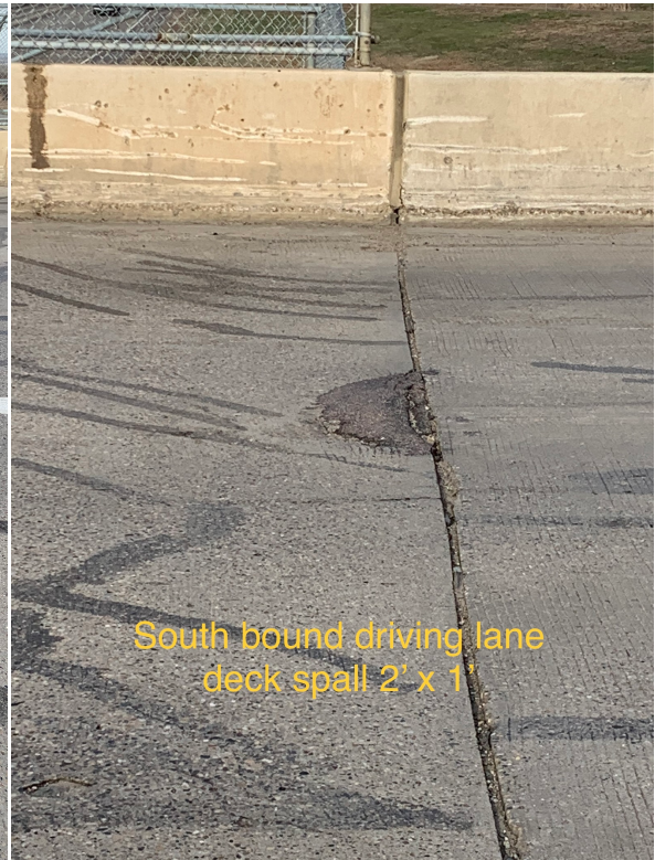
North bound South end deck spalls
