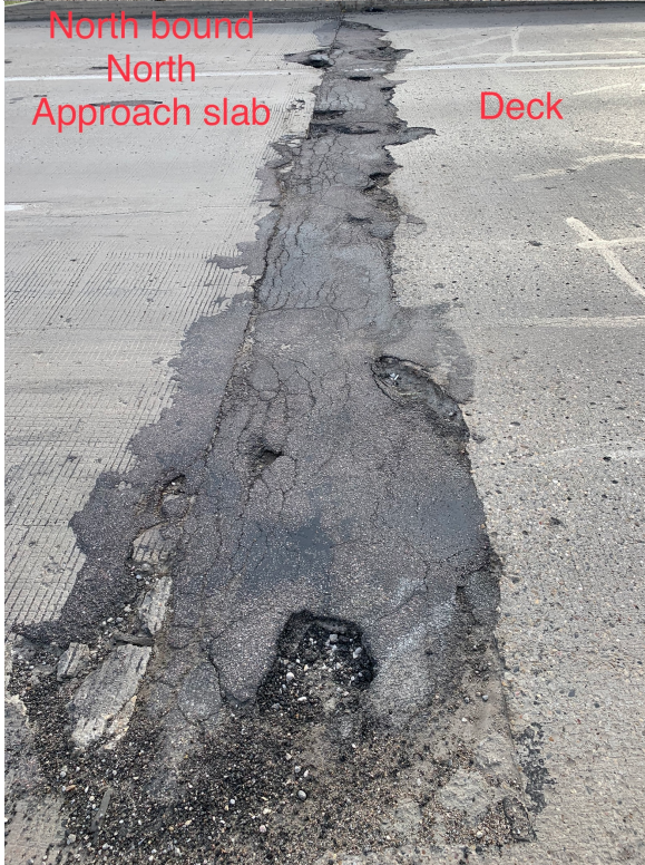
North bound South end deck spalls
