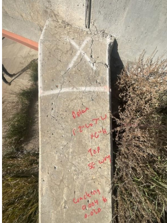
Photo 11: Spall repair at southeast wingwall (6 SF)
