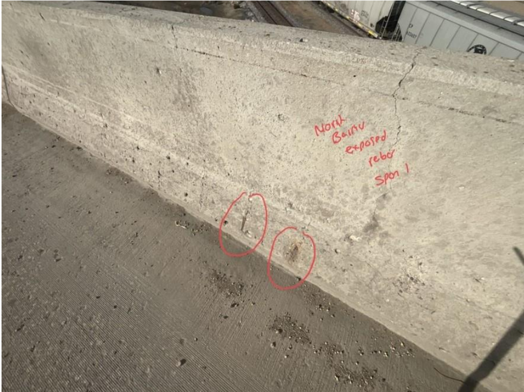
Photo 1: Spall repair at north barrier in Span 1 (2 SF)
