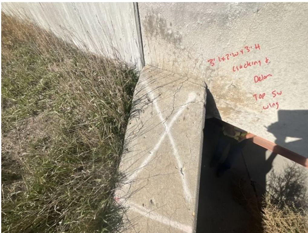
Photo 8: Spall repair at southwest wingwall (6 SF)
