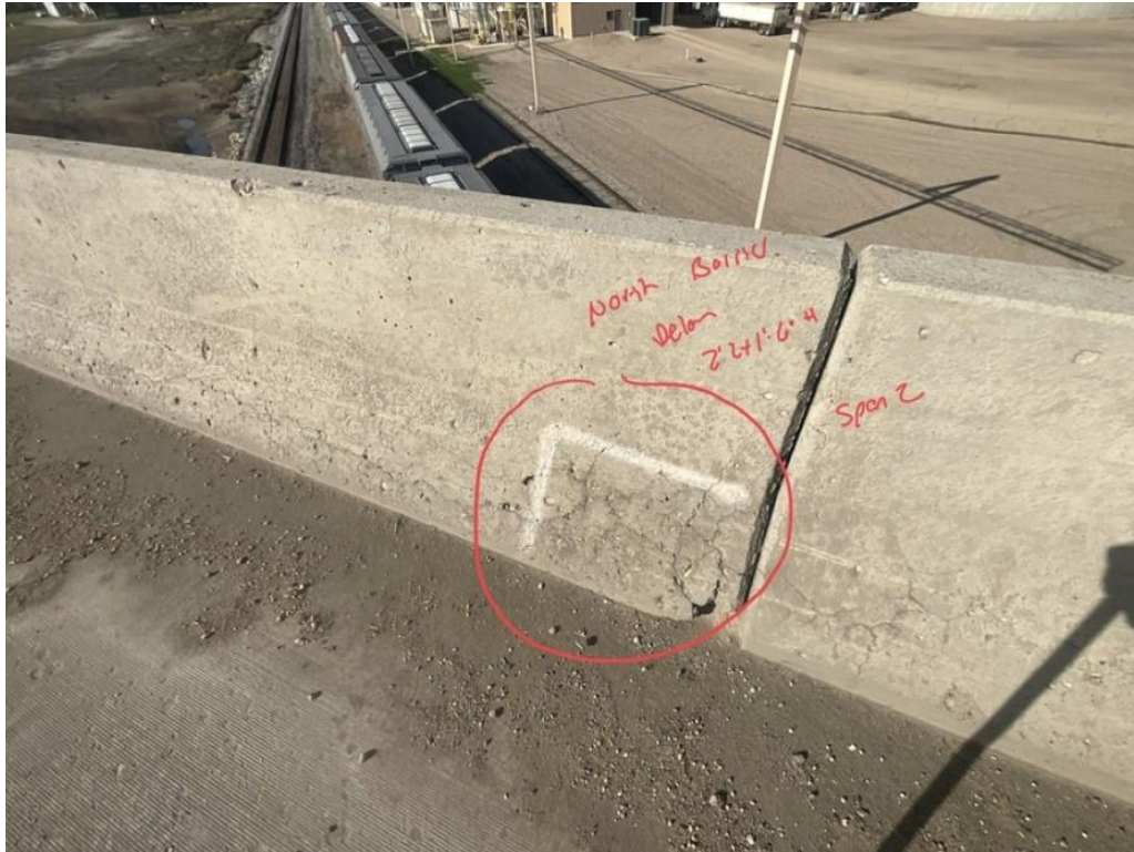
Photo 3: Spall repair at north barrier in Span 2 (3 SF)
