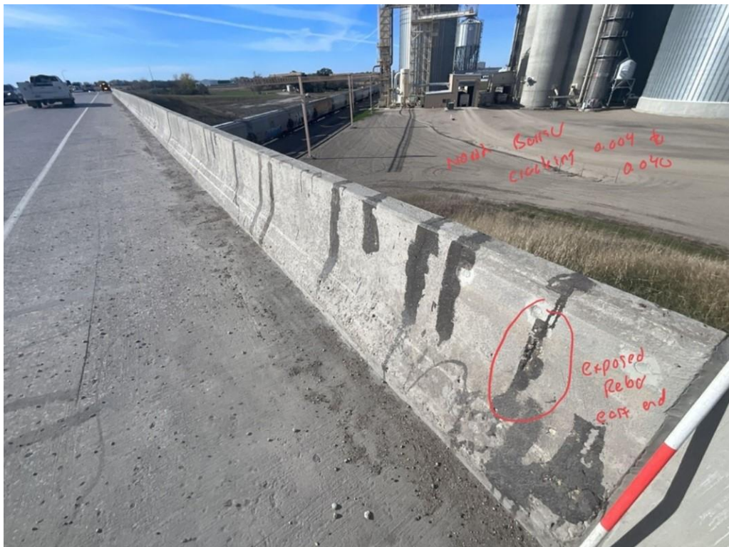
Photo 4: Spall repair at north barrier in Span 3 (2 SF)
