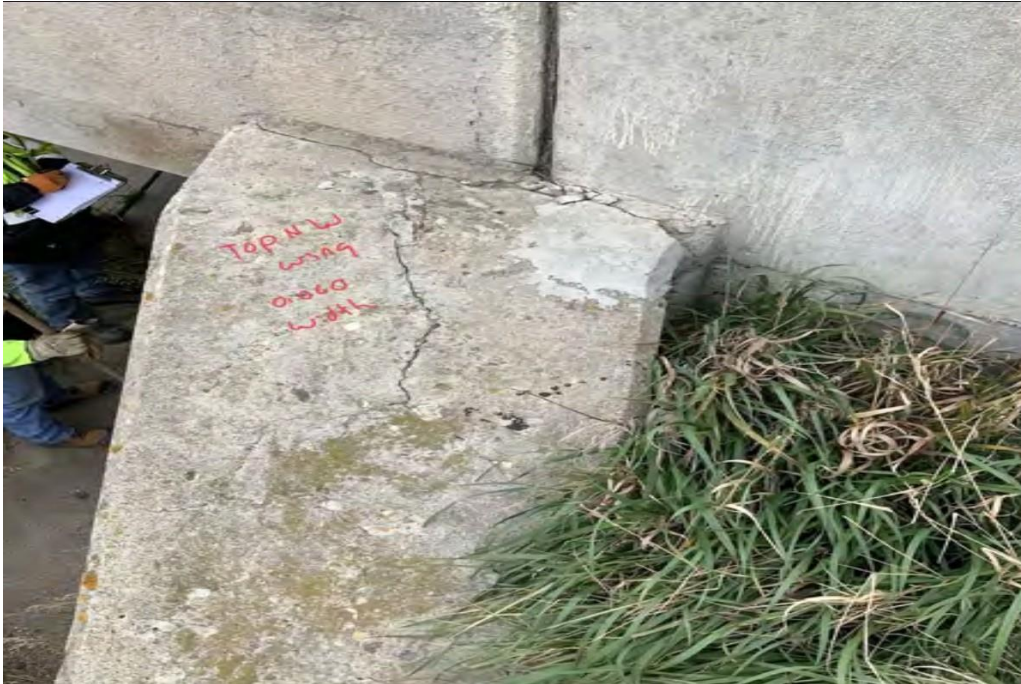
Photo 9: Spall repair at northwest wingwall (6 SF)
