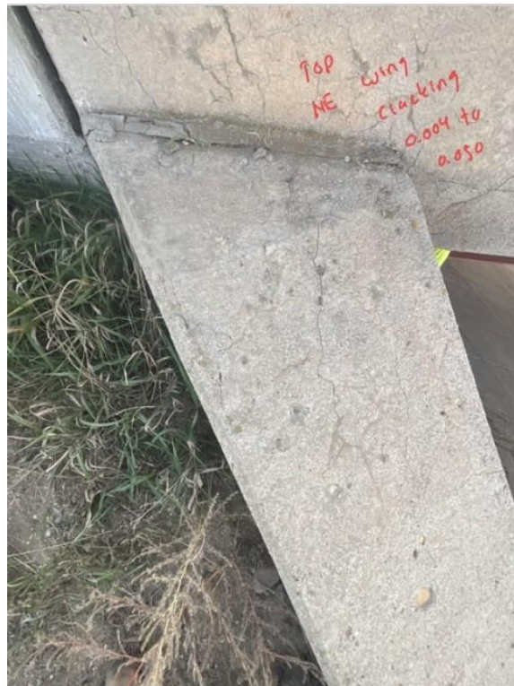
Photo 10: Spall repair at northeast wingwall (6 SF)
