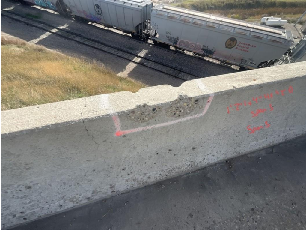
Photo 5: Spall repair at south barrier in Span 3 (4 SF)
