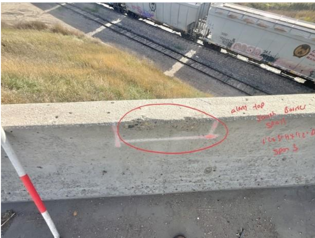
Photo 6: Spall repair at south barrier in Span 3 (3 SF)
