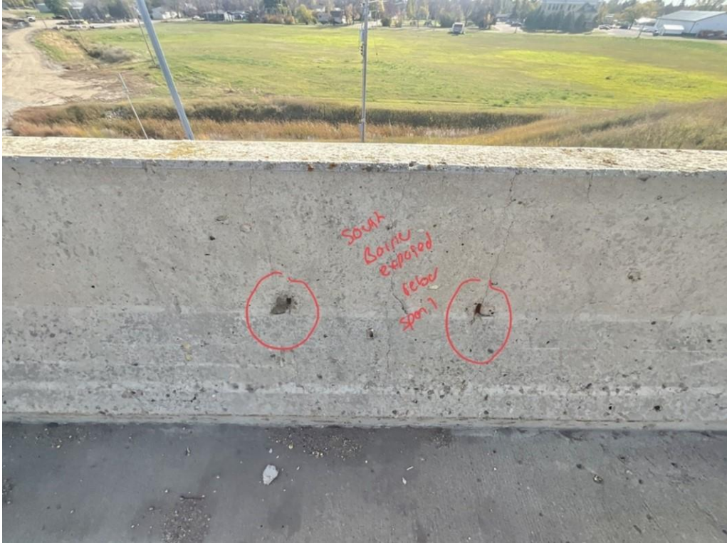
Photo 7: Spall repair at south barrier in Span 1 (2 SF)
