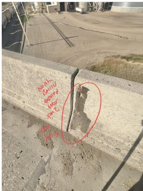
Photo 2: Spall repair at north barrier in Span 2 (3 SF)
