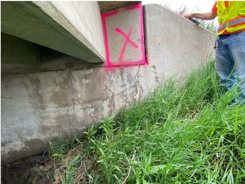
Photo 6: Spall repair at Abutment 3 (5 SF)
