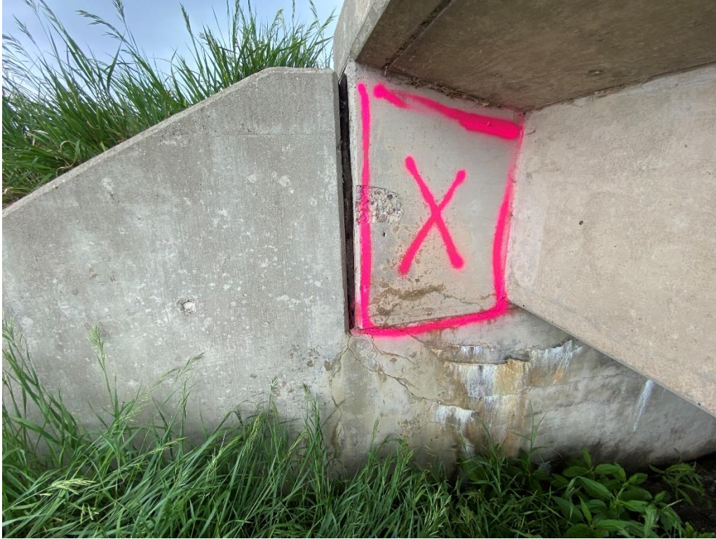
Photo 1: Spall repair at Abutment 1 (5 SF)
