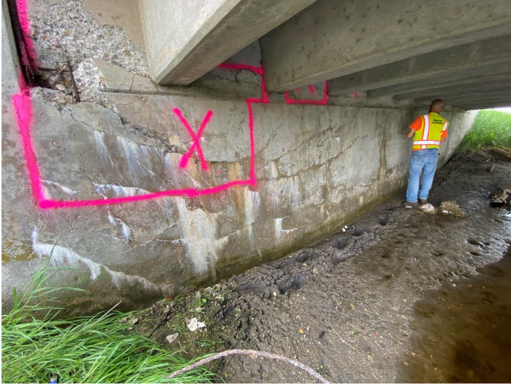
Photo 5: Spall repair at Abutment 3 (5 SF/Girder Bay = 35 SF)
