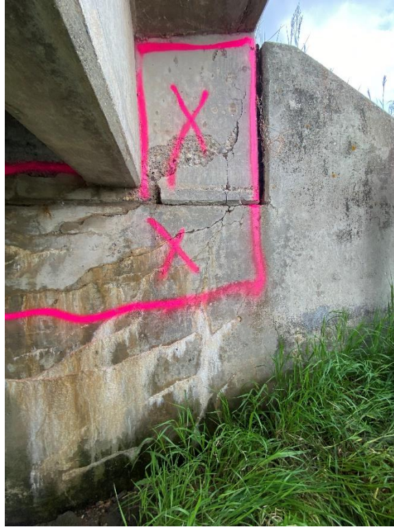
Photo 3: Spall repair at Abutment 1 (11 SF)
