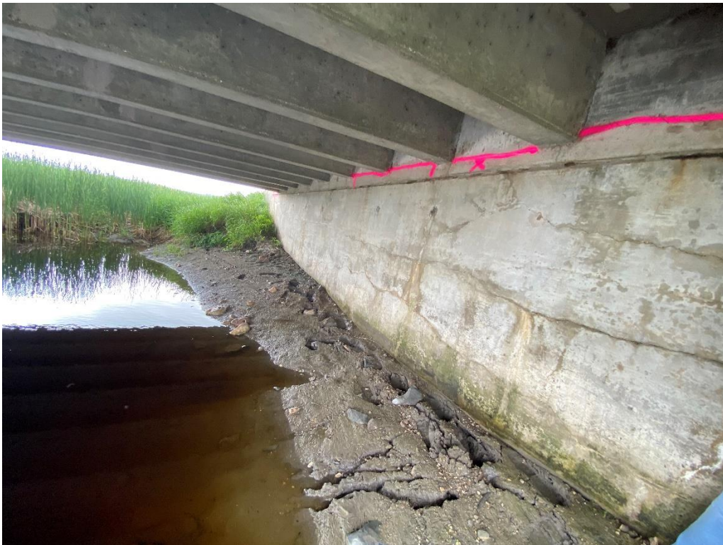
Photo 2: Spall repair at Abutment 1 (16 SF)
