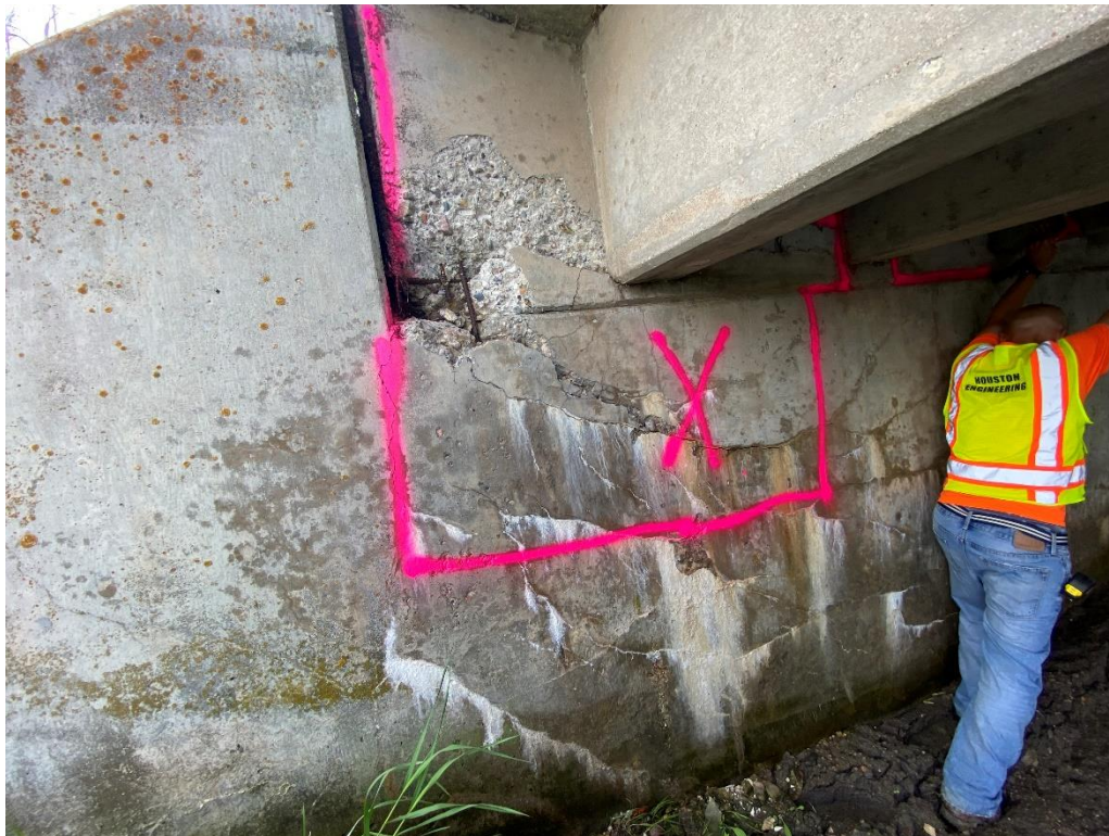
Photo 4: Spall repair at Abutment 3 (18 SF)
