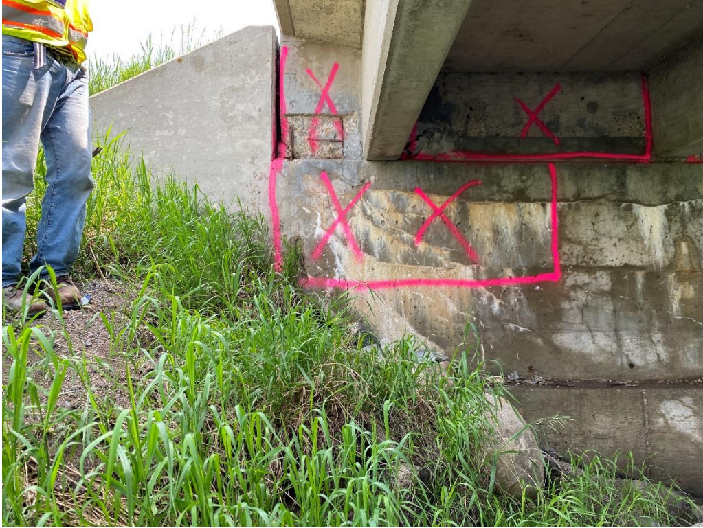
Photo 5: Spall repair at Abutment 4 (15 SF)
