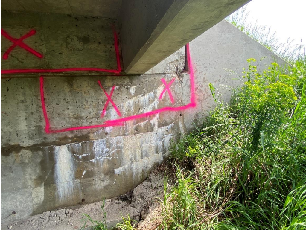
Photo 7: Spall repair at Abutment 4 (11 SF)
