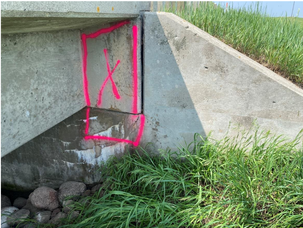
Photo 4: Spall repair at Abutment 1 (7 SF)
