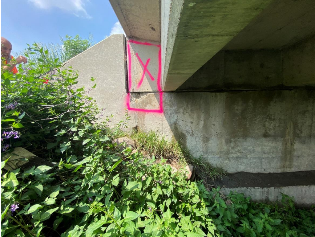
Photo 3: Spall repair at Abutment 1 (7 SF)
