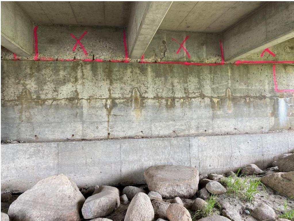
Photo 6: Spall repair at Abutment 4 (12 SF/ Girder Bay = 60 SF)
