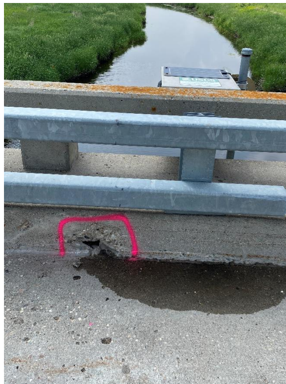
Photo 2: Spall repair in south curb (1 SF)
