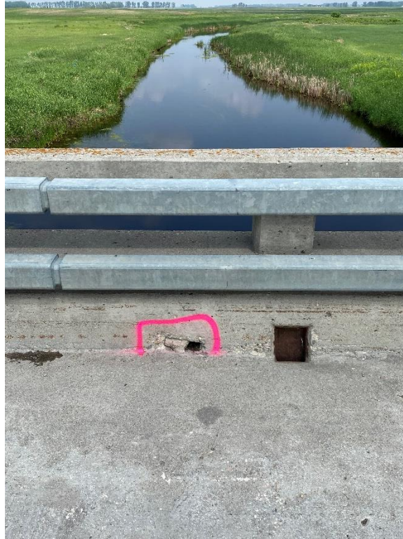
Photo 1: Spall repair in north curb (1 SF)
