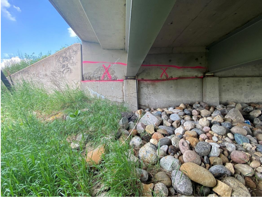
Photo 1: Spall repair at Abutment 1 (24 SF)
