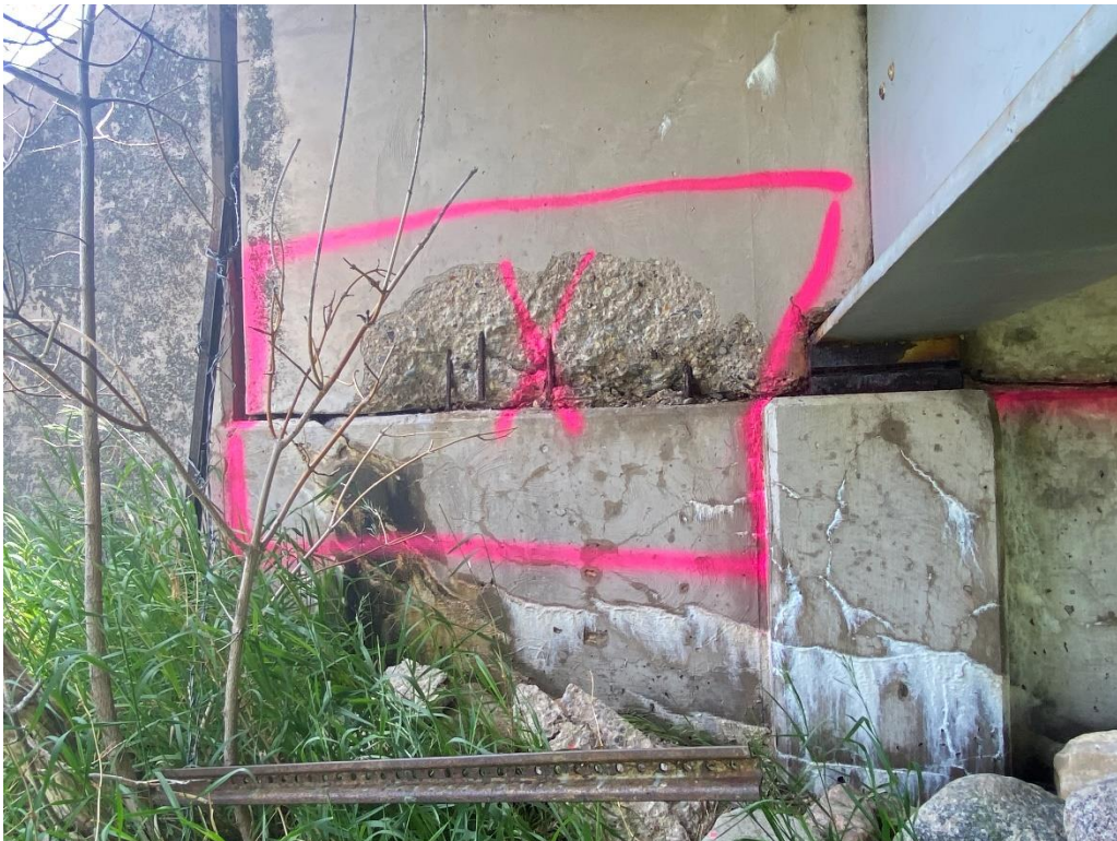
Photo 4: Spall repair at Abutment 4 (16 SF)
