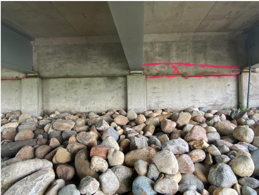
Photo 2: Spall repair at Abutment 1 (9 SF)
