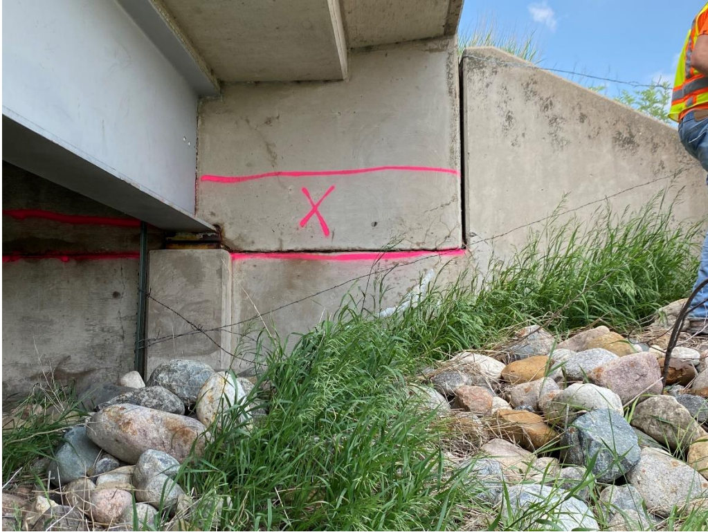
Photo 3: Spall repair at Abutment 1 (9 SF)
