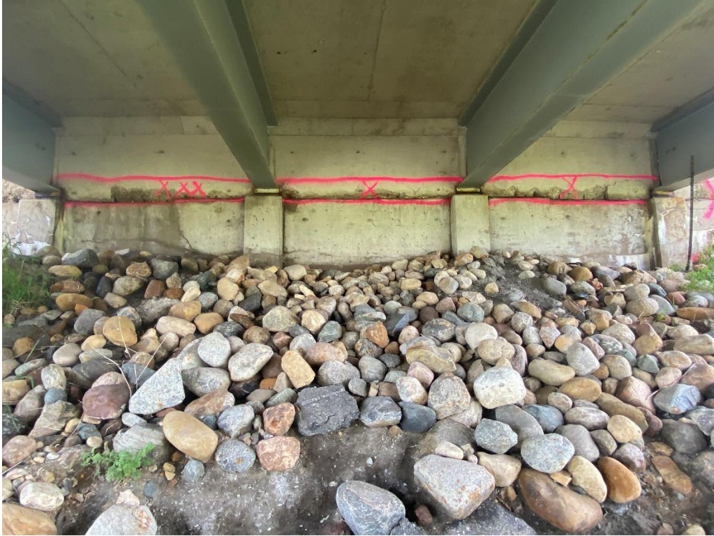
Photo 5: Spall repair at Abutment 4 (26 SF)
