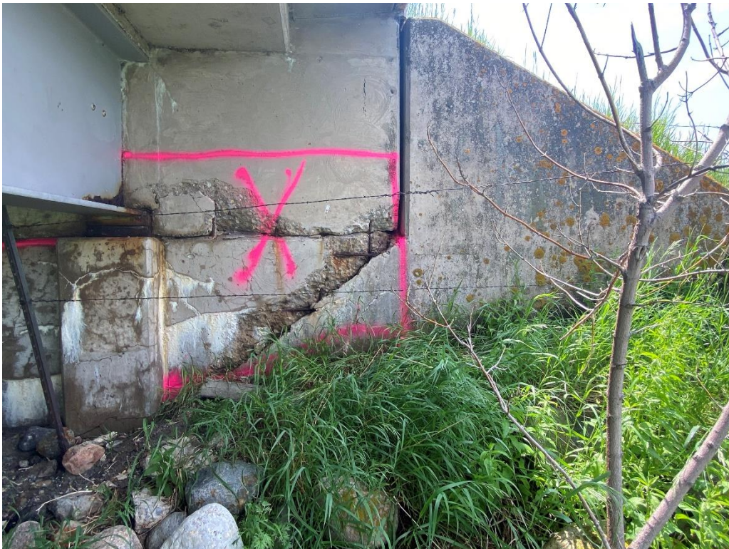
Photo 6: Spall repair at Abutment 4 (22 SF)
