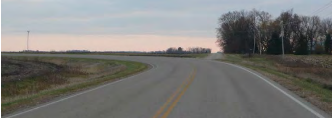
FIGURE 2-9 Example of a Visual Trap – Minor Road Intersects Roadway on a Curve
